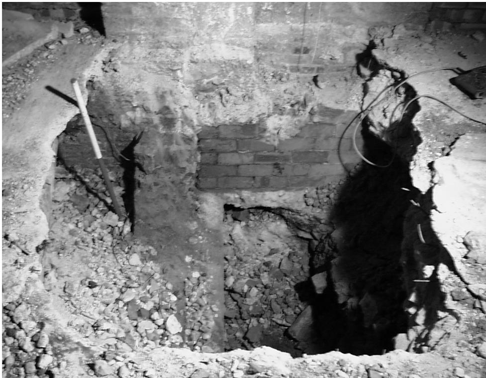
**Fig b** Cellar wall exposed in Test pit 2.
