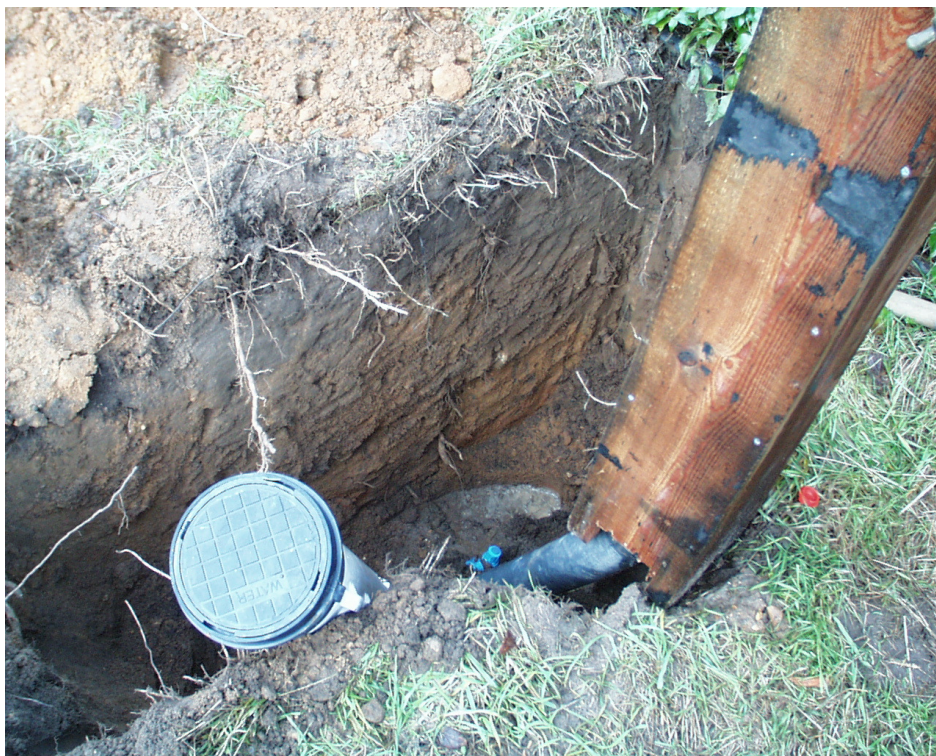
Plate 1 The trench after the stand-pipe had been inserted, looking south-west.
