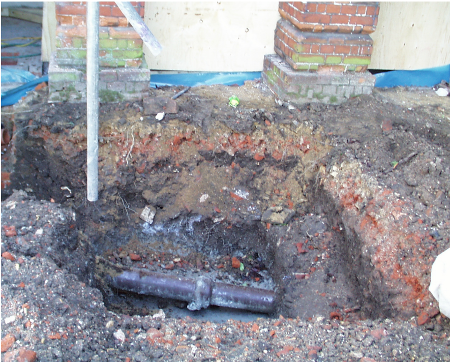
Plate 2 Manhole trench, looking south.
