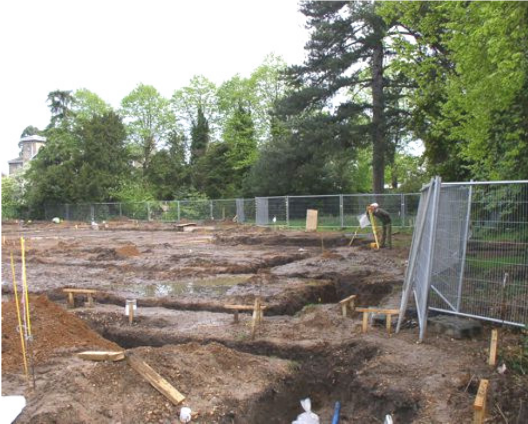
Plate 2: the site during excavation, view north-east (frame ref: 2448)
