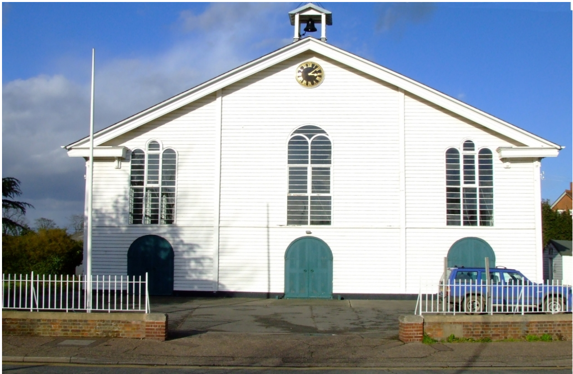
Figure 2. The Garrison Chapel, Colchester, from southwest, March 2007.
