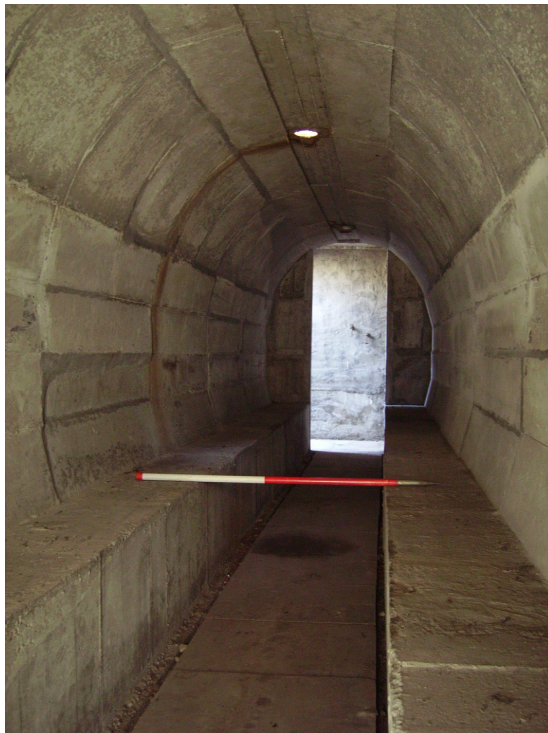
Plate 12: Shelter F1, Area J1 – internal view, looking north-east.
