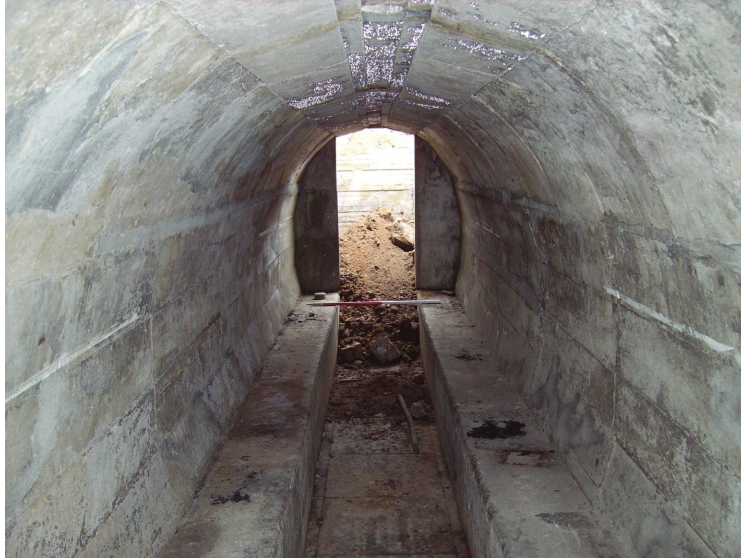
Plate 18: Shelter F1, Area P1 – internal view, looking north.
