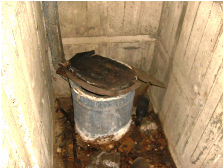
Plate 8: Shelter 3, Area C2 – detail of toilet in west recess, showing waste-gases pipe, looking south.
