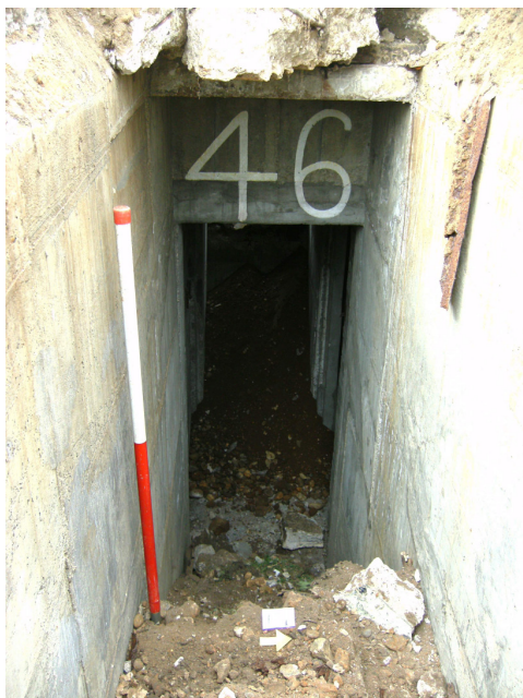
Plate 17: Shelter F1, Area P1, south entrance, showing white-painted number, looking west.
