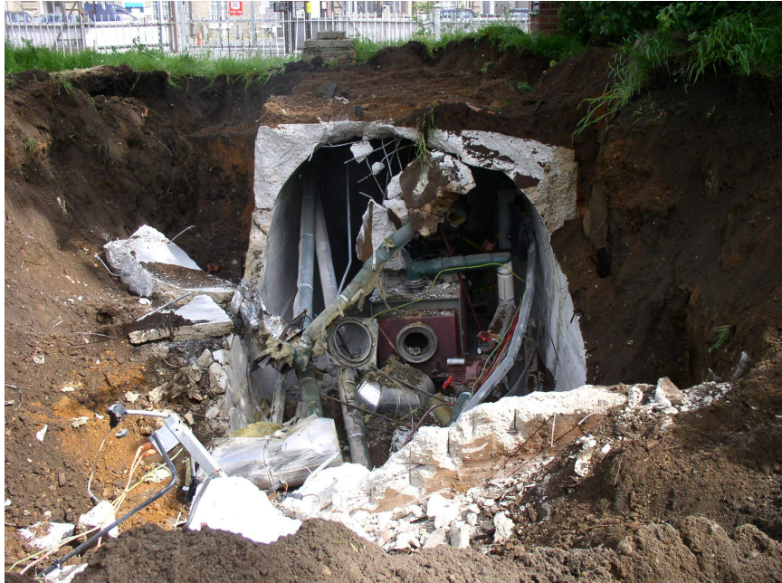
Plate 5: Shelter 2, Area C2 – south-western end during demolition, looking north north-east.
