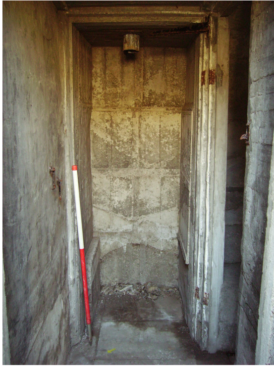
Plate 13: Shelter F1, Area J1 – detail of door hinges and latches, looking south-east.
