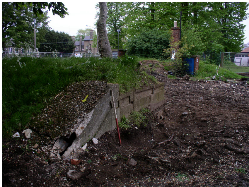
Plate 1 (above): Shelter 1, Area C2 – south-western corner, looking east, with shelter 2 in the background.
