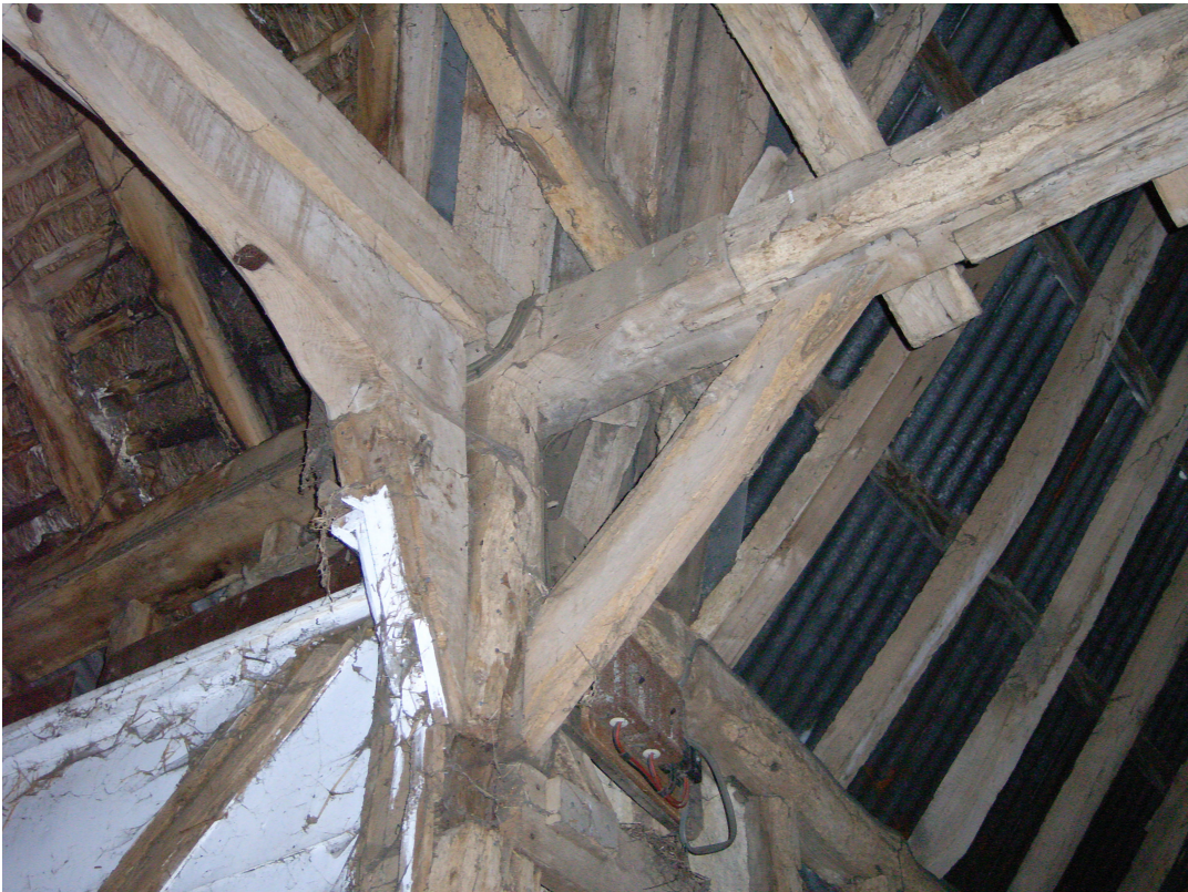
A2.10 Barn (1). Detail of face-halved-and-bladed (right) scarf joint in roof-plate above porch.
