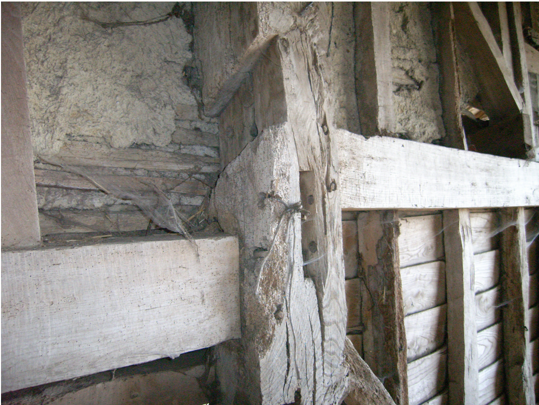
A2.8 Detail of passing brace trench in re-used storey post between bays B and A (left to right).
