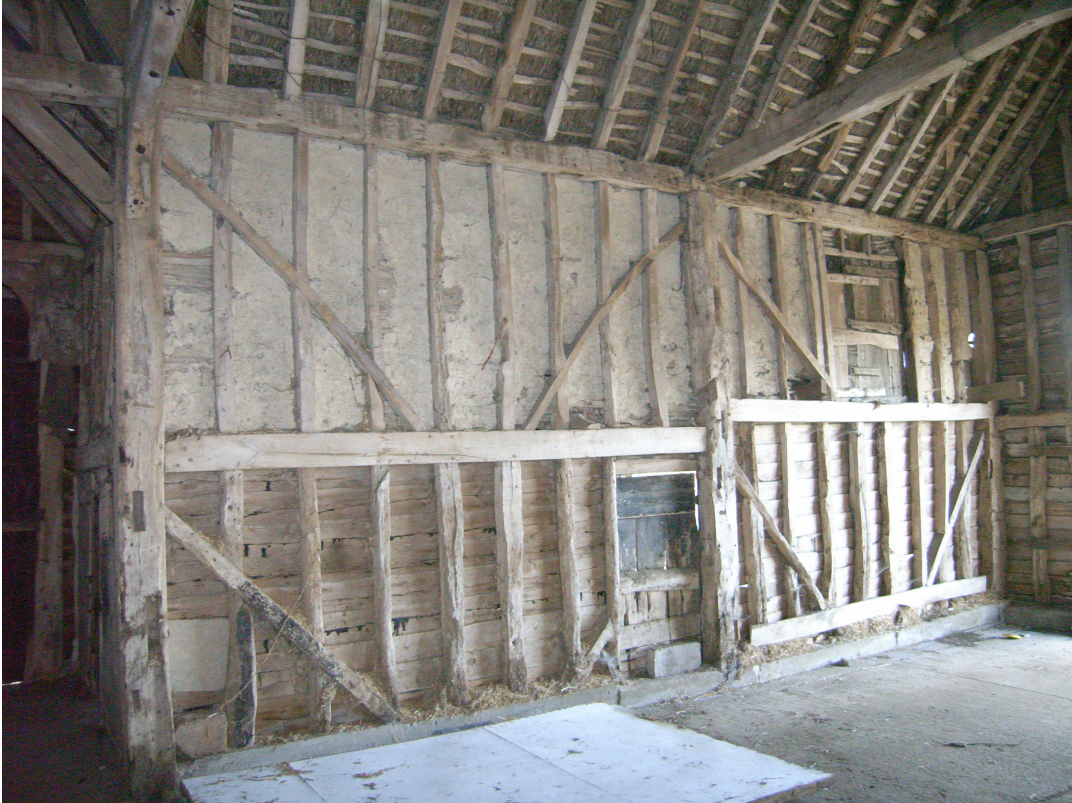
A2.7 Barn (1). Interior of bays B and A (left to right) from south-east, showing door and blocked hatch with re-used central storey post.
