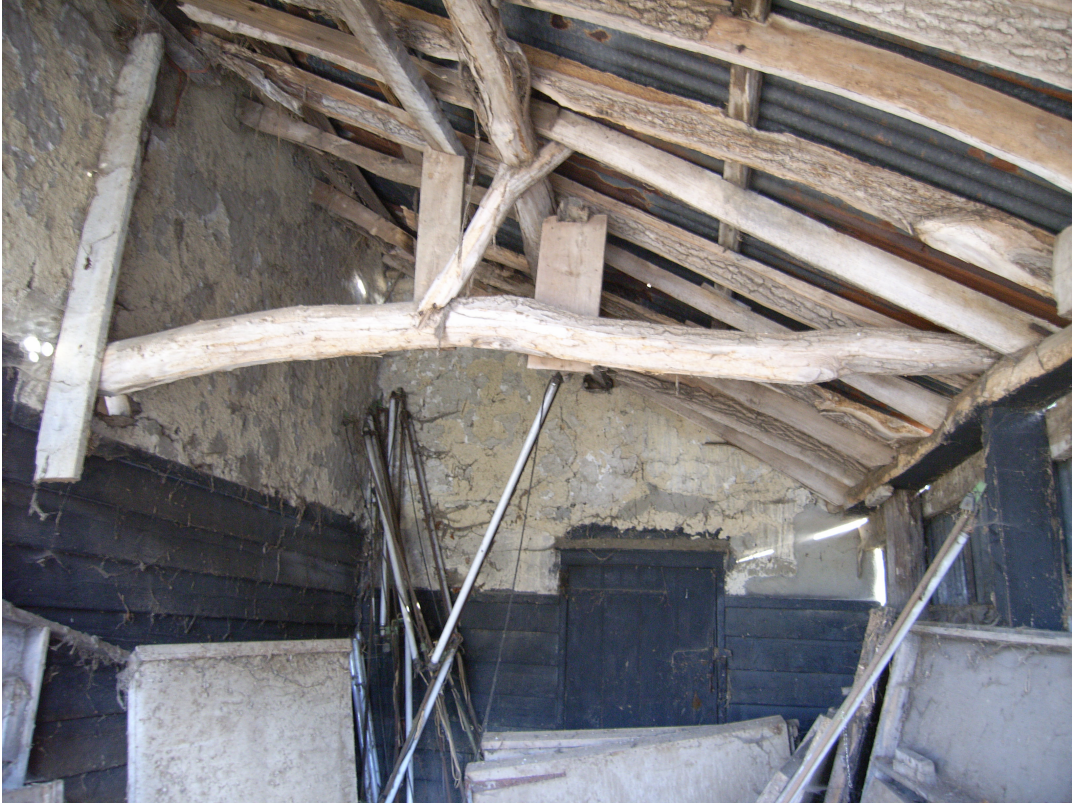
A2.9 Barn (1). Interior of northern lean-to from north, showing side-door of porch and original external cladding of roughcast daub above weatherboarding.
