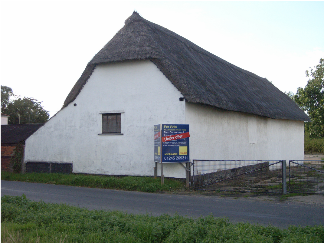
A2.4 Barn (1). Exterior from south-east, showing hatch in southern gable.
