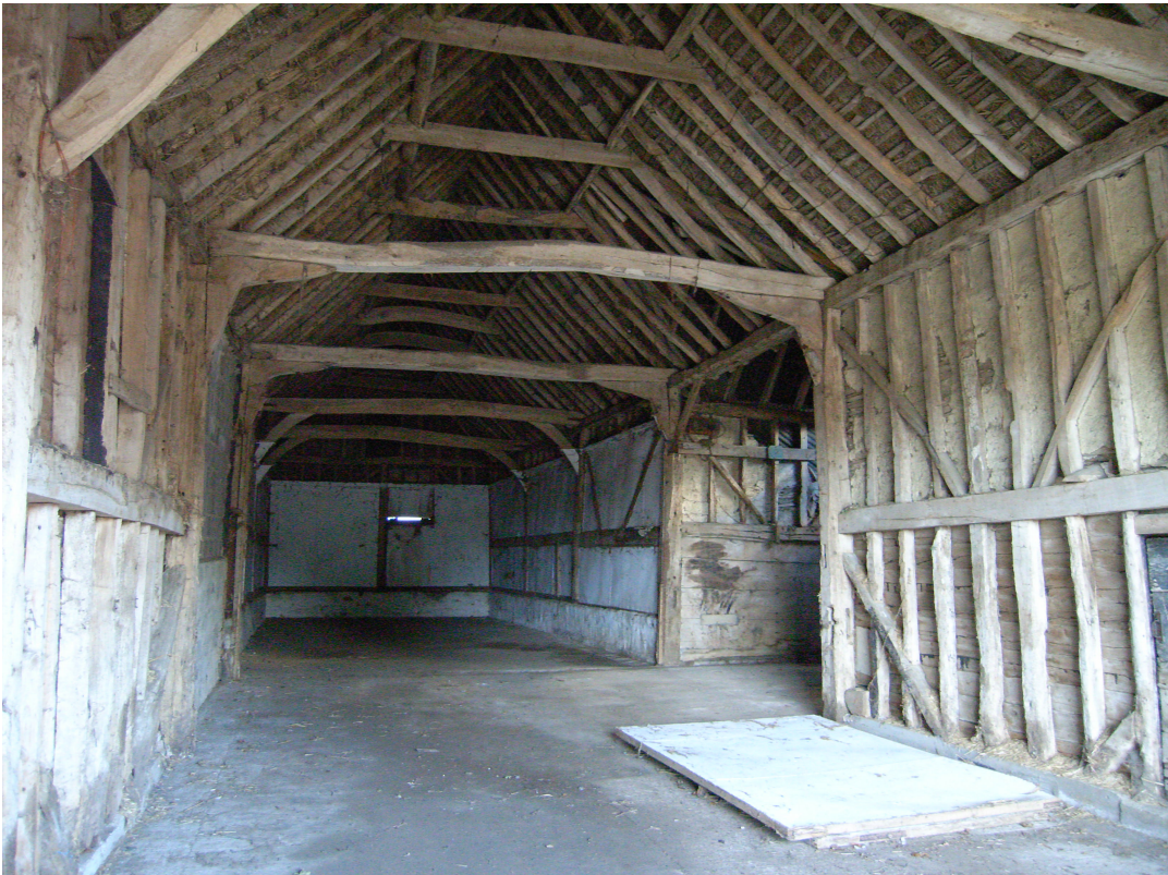
A2.6 General internal view of barn (1) from north.
