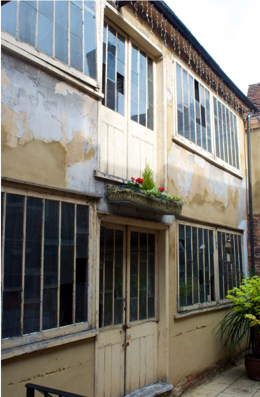
31 East elevation of Day's Warehouse.
