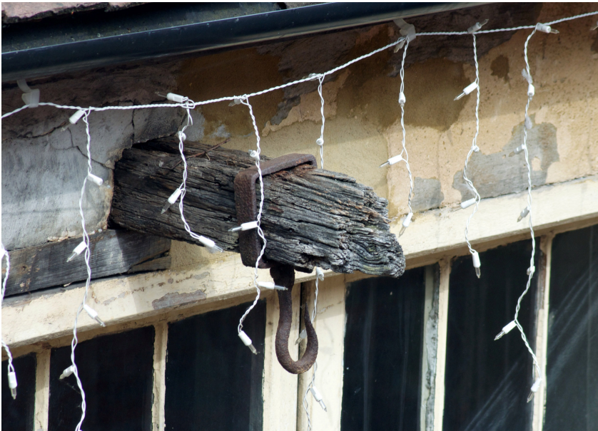
32 Surviving part of the lifting gear on the east elevation of Day's Warehouse.
