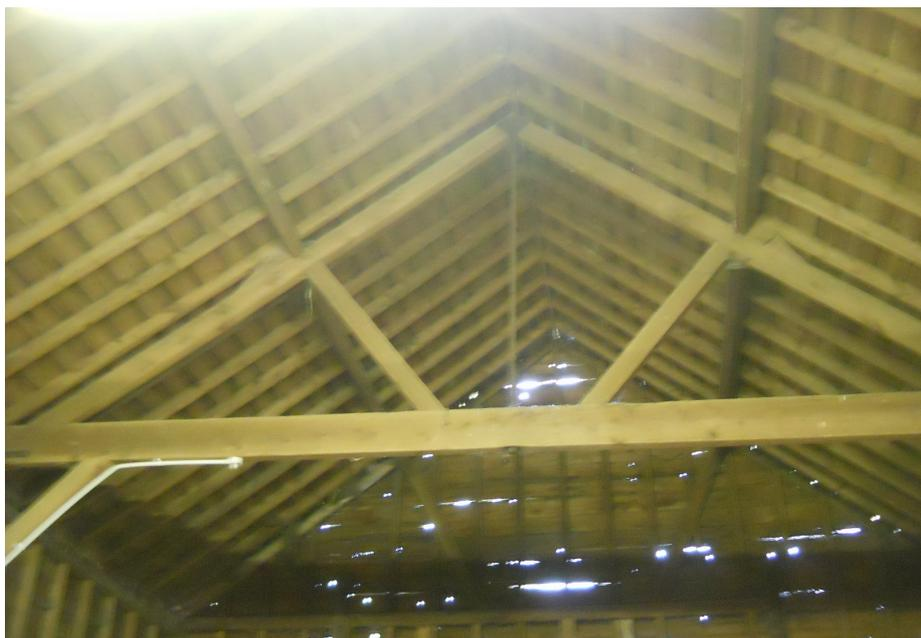
**Plate 10 Large barn (E), interior, roof truss with part of down brace to post.**
