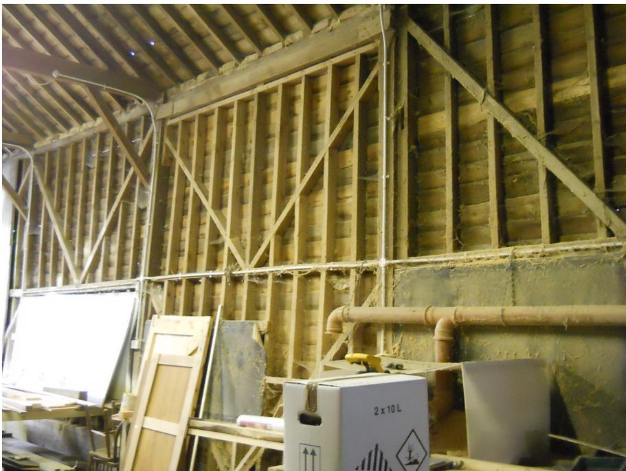
**Plate 9 Large barn (E), interior, north-east wall, showing blocking of central door by matching framing.**
