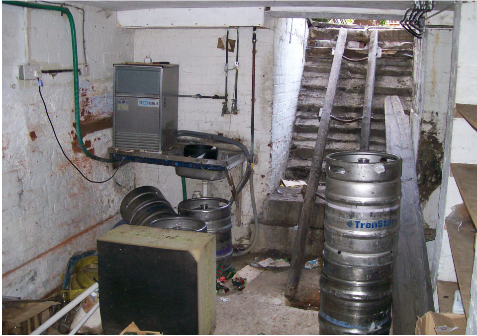
Plate 6 The cellar hatch and barrel ladder.
