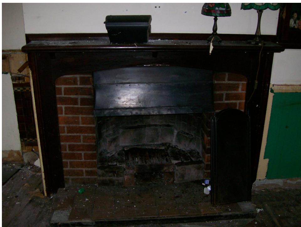
Appendix Plate 8 The lounge fireplace.
