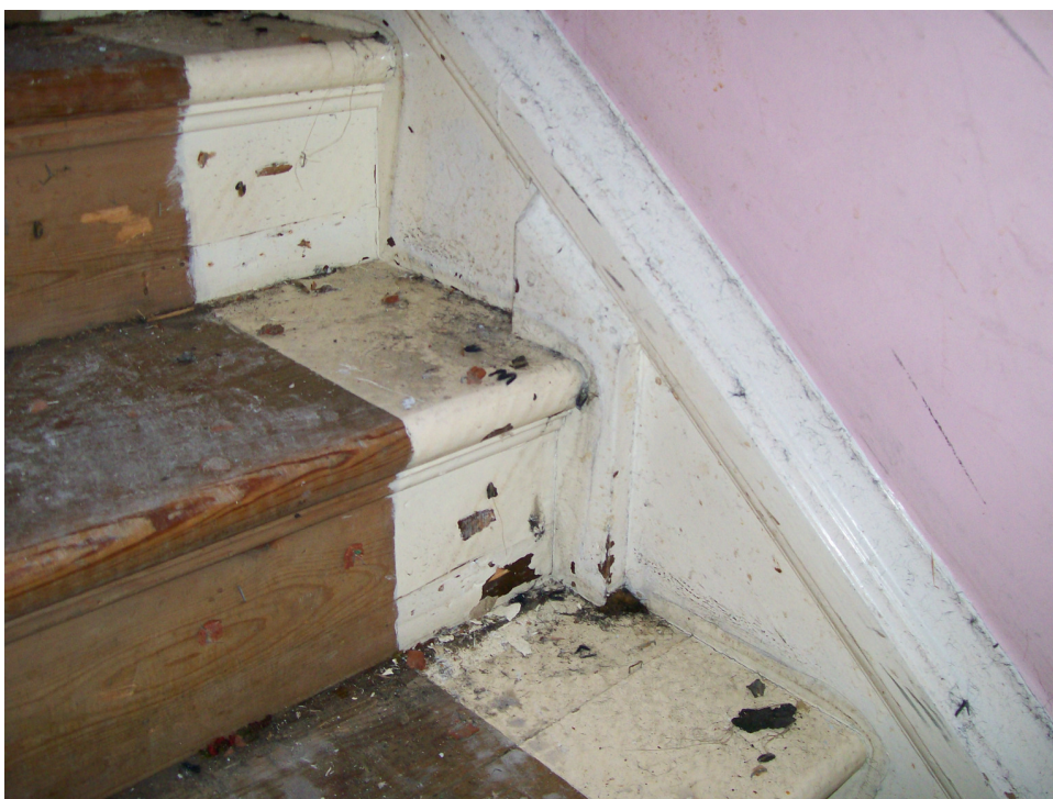
Appendix Plate 13 Groundfloor stairs with remains of original newel post.
