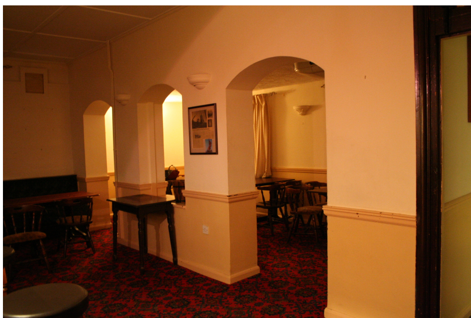
Appendix Plate 10 The extension to the lounge cut through the original west wall.
