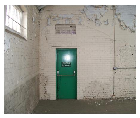
Plate 9: Building 5; the bricked-in archway of the original entrance with modern fire door where the opening would have been.
