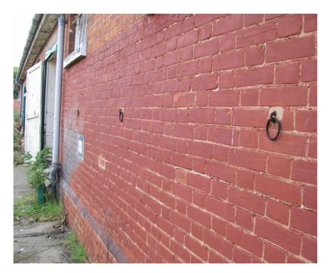
Plate 8: tethering rings on exterior of Building 5.
