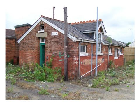
Plate 12: Building 7; the Ablution House with replacement dormer window and inserted entrance on short elevation. The later extension can be seen to the rear.
