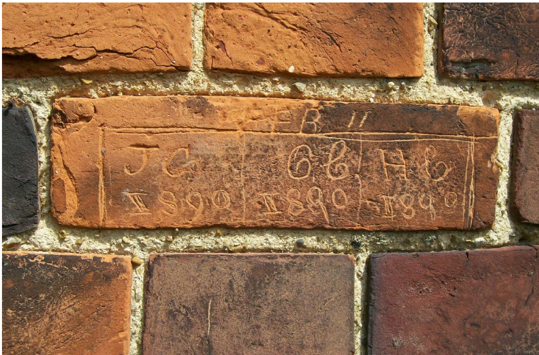
Plate 8 Graffiti dated 1890 on west wall of No.2.
