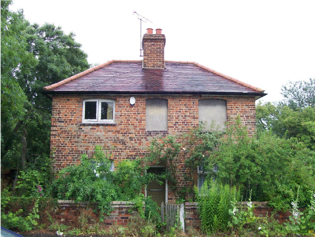
Plate 15 No.3 showing blocked windows and alterations to remaining fenestration.
