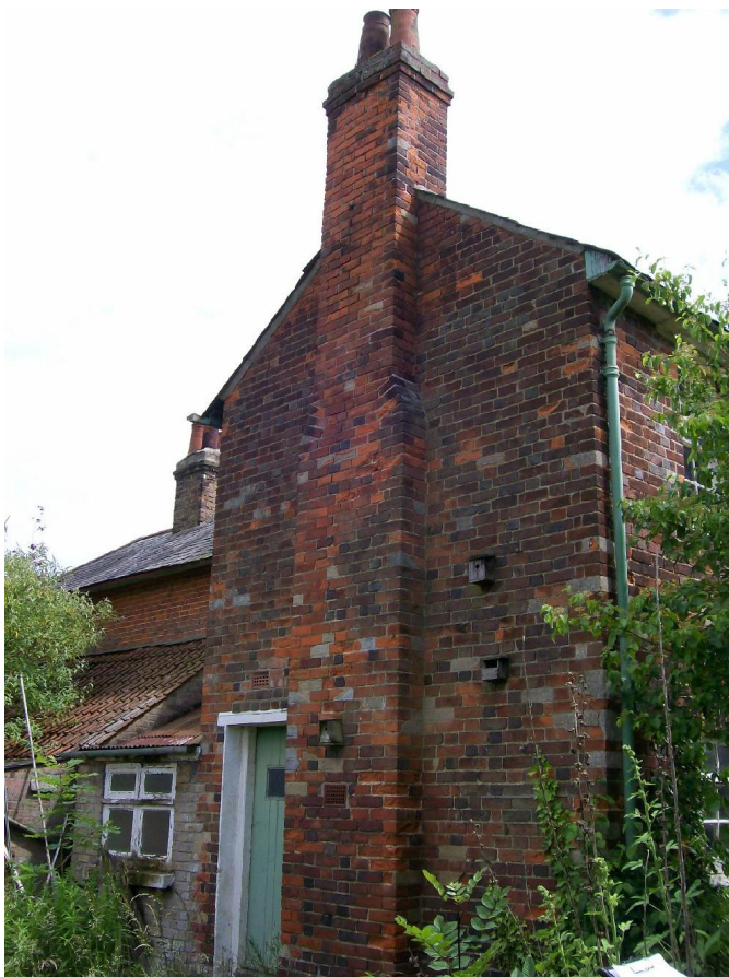
Plate 9 No.2 north elevation showing later extensions
