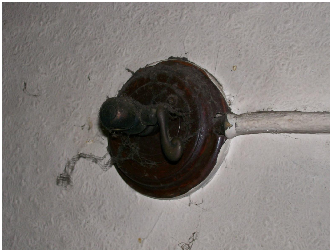
Plate 13 Early gaslight fitting.
