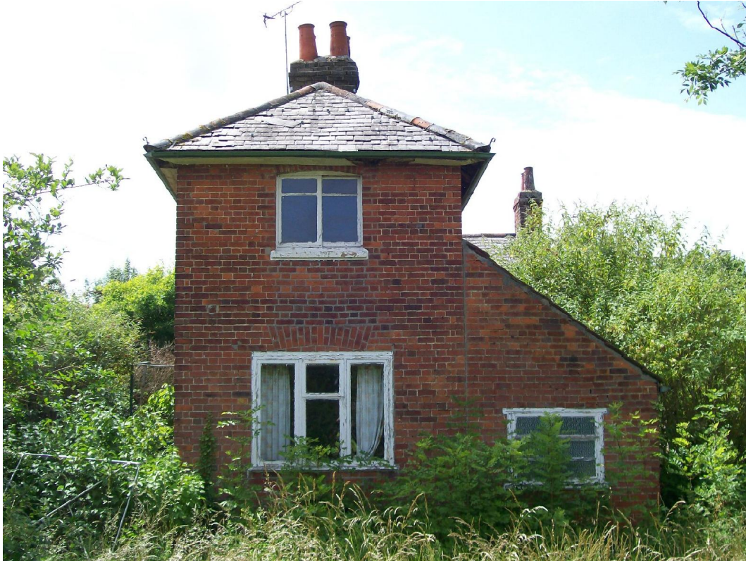
Plate 7 No.1 east elevation showing altered windows and the earliest phase of extension.
