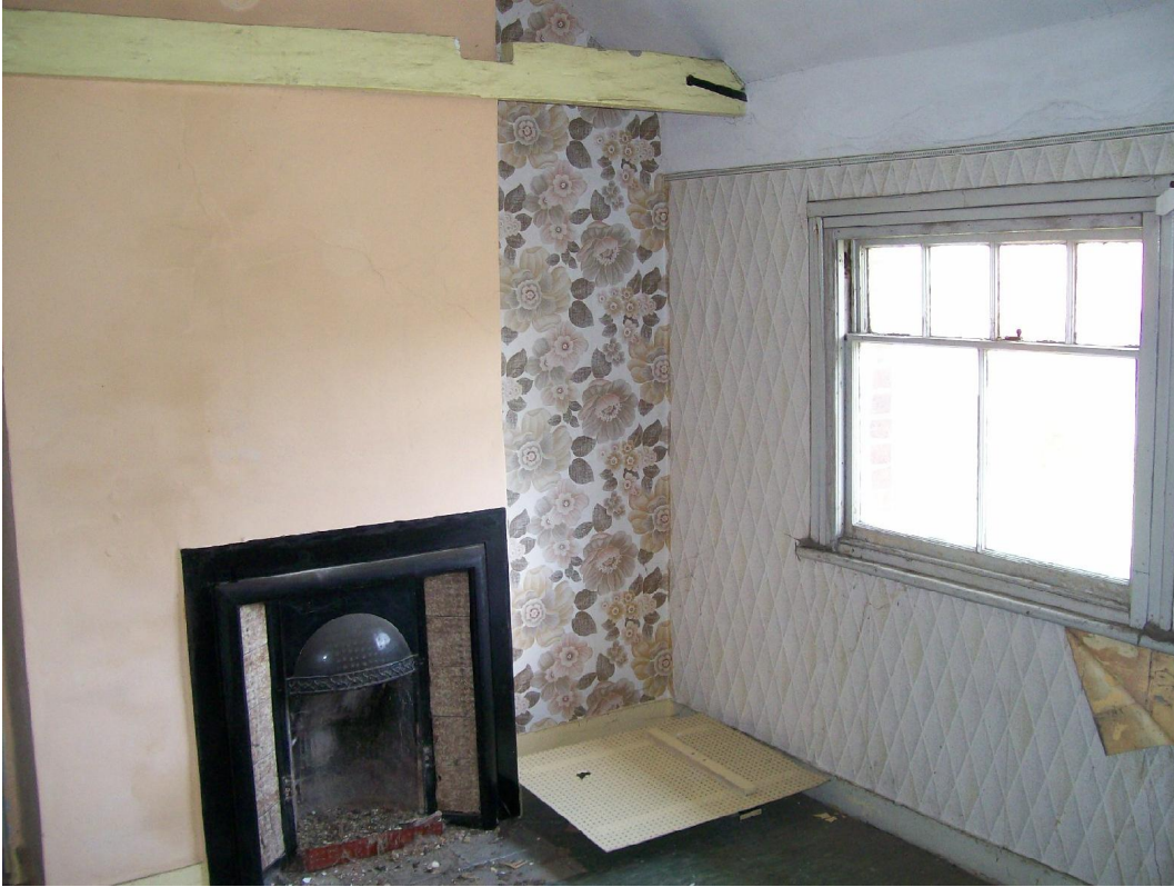
Plate 11 No.1, bedroom 1 showing the wooden tie beam, Victorian fireplace and the four-over-two hybrid sash window.
