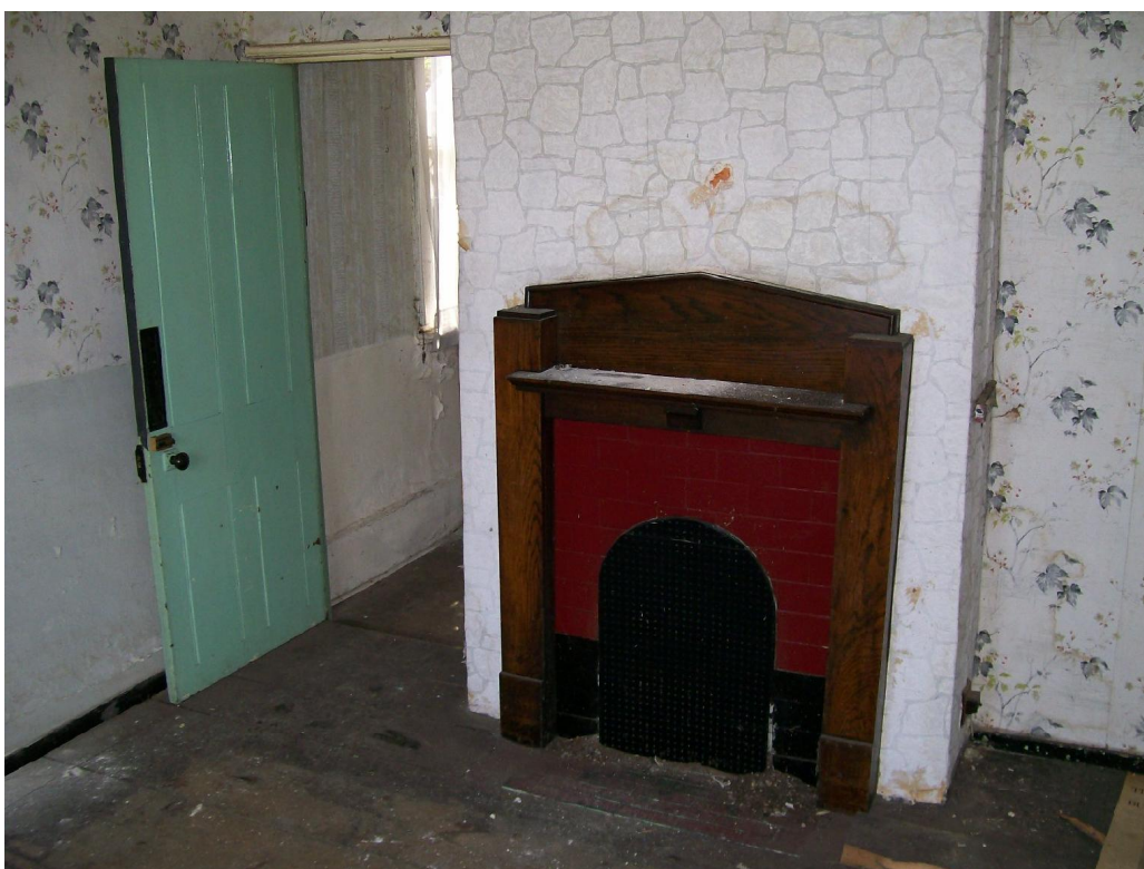
Plate 10 No.1 room 2 fireplace with possible contemporary grate.
