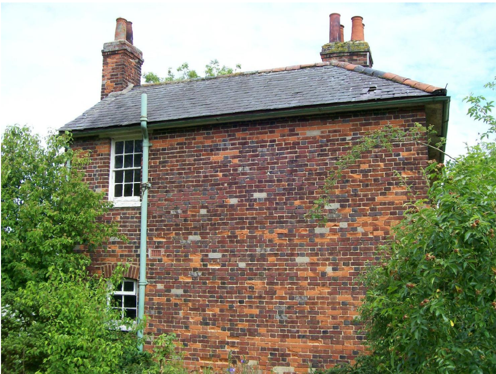
Plate 4 The west elevation of No.2 showing the lower quality brickwork.
