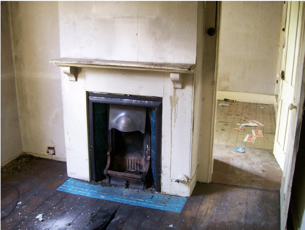
Plate 12 The fireplace in ground floor room 2 of No.2 with the original hardwood flooring to the foreground and the later softwood flooring of the extension to the rear.
