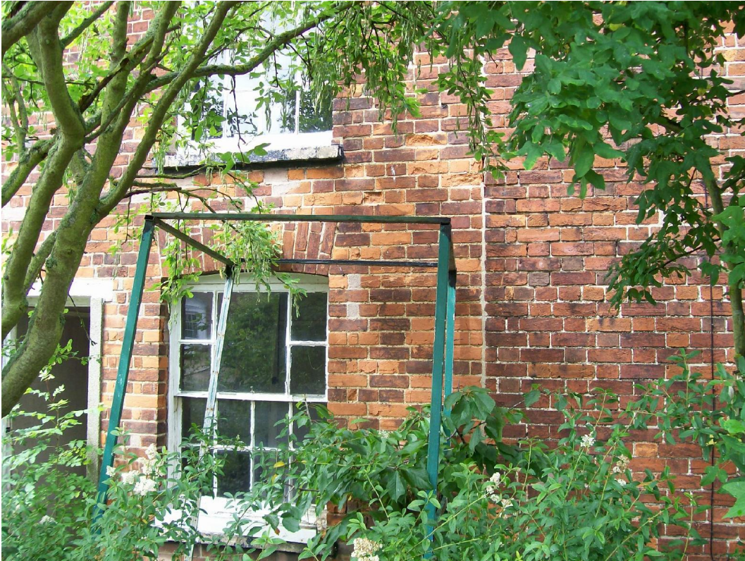
Plate 5 The join between Nos.1 and 2 and the repaired sash window.
