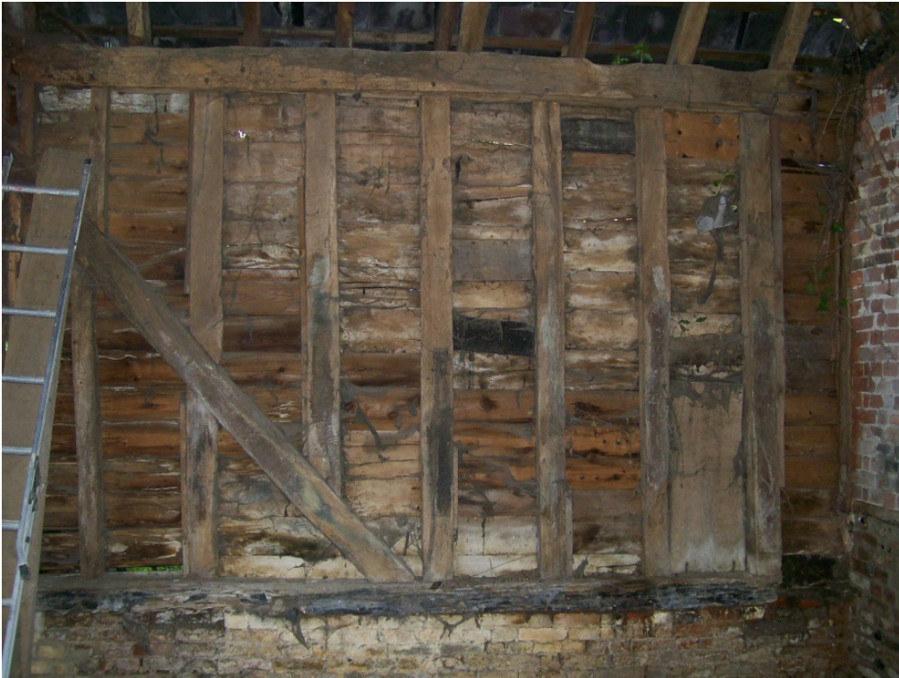
Plate 5 Bay 1, south-west wall frame with internal plank brace - view south-west
