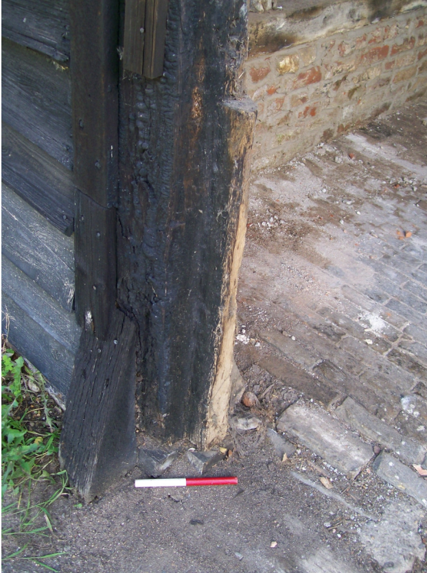
Plate 13 Recess for the original threshold leap
