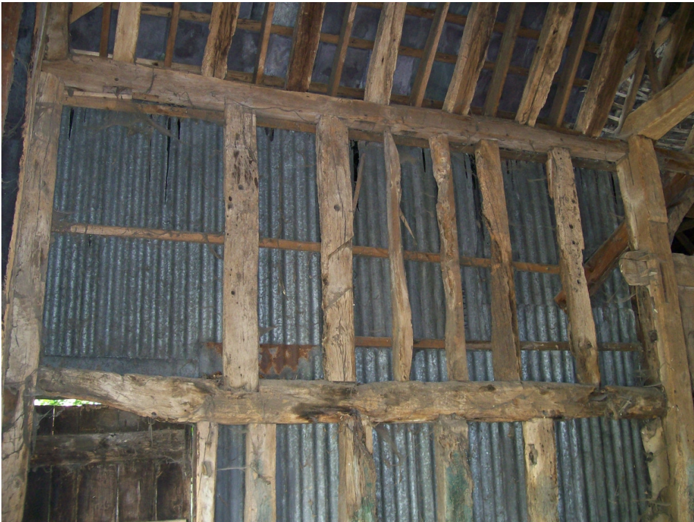
Plate 12 Midstrete, north-west wall frame, showing greater height of corner posts
