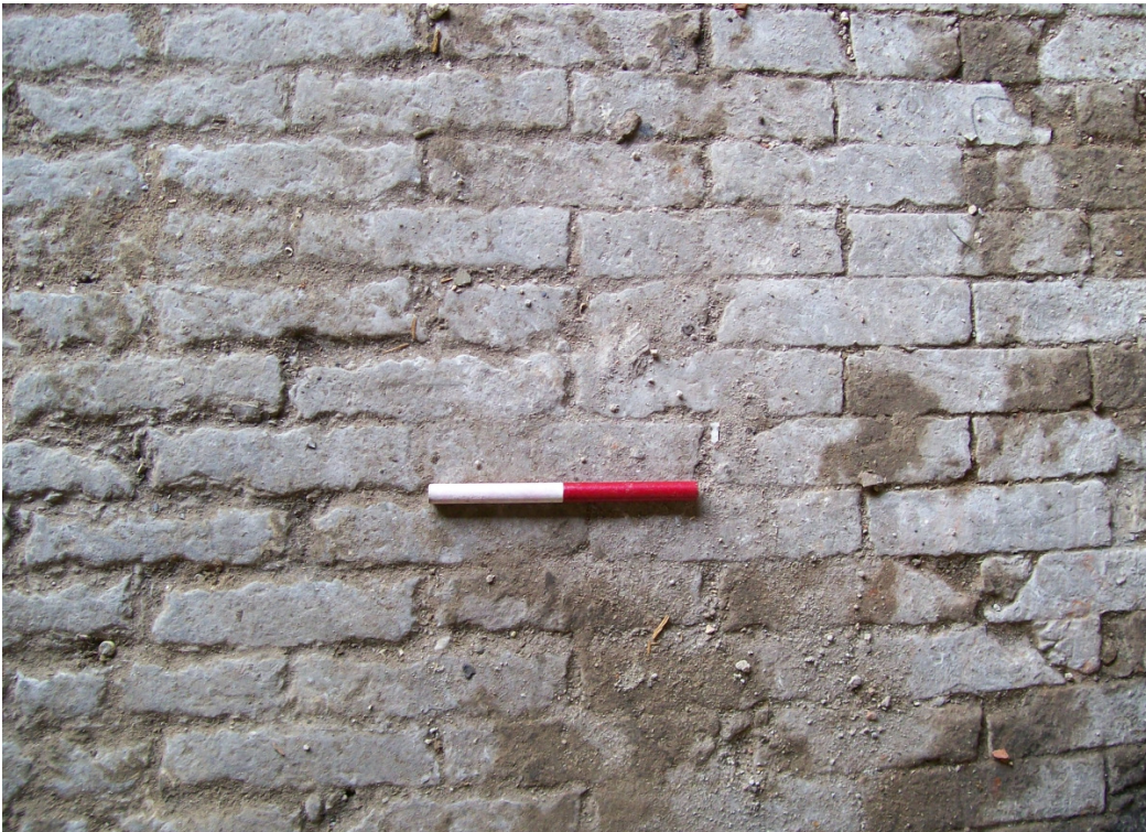
Plate 4 Brick threshing floor showing worn bricks to the left
