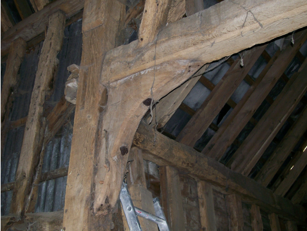
Plate 9 Elbow brace at south-west end of truss A with midstrey to the left
