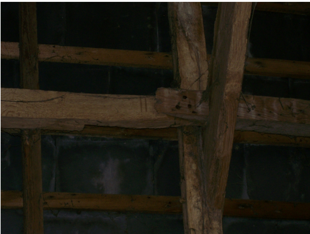
Plate 16 Bay 1, carpenters' mark (II) on purlin of north-east roof pitch and splayed scarf joint
