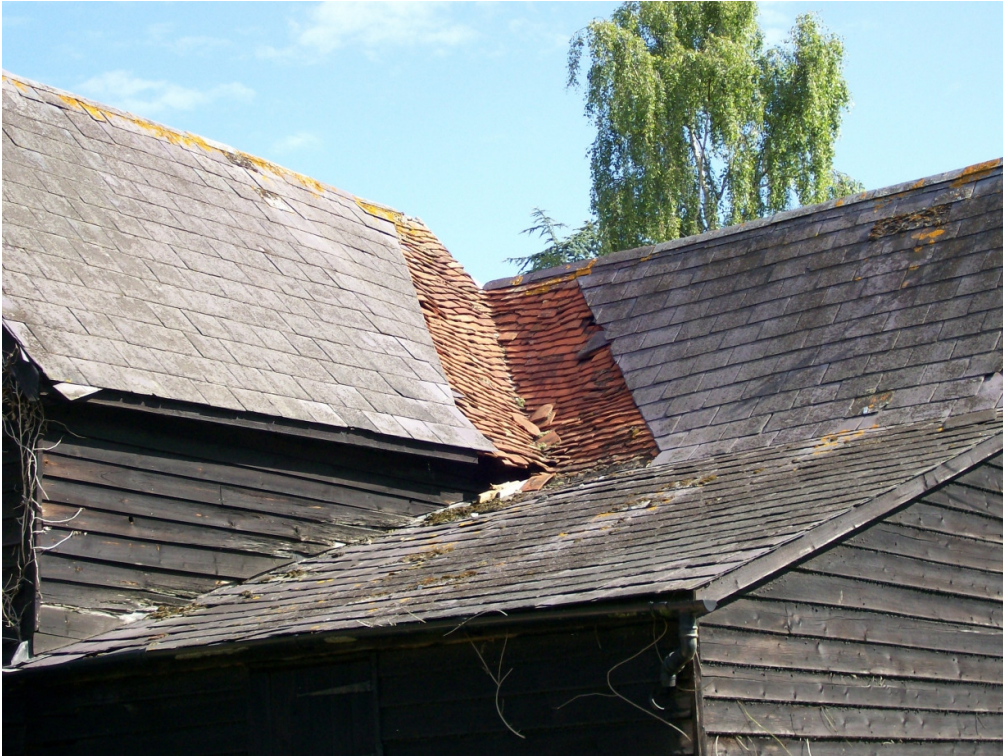
Plate 1 Peg-tile valley between main barn and midstrey - view north
