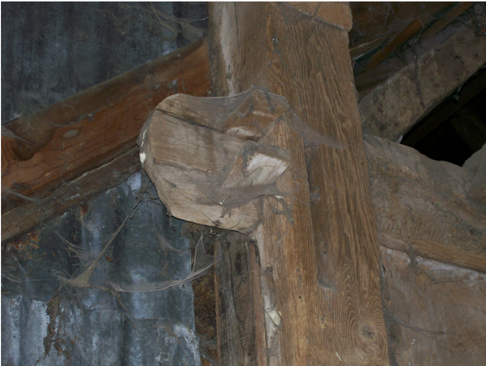
Plate 10 Tie-beam of truss A tusk-tenoned through inner midstrey corner post
