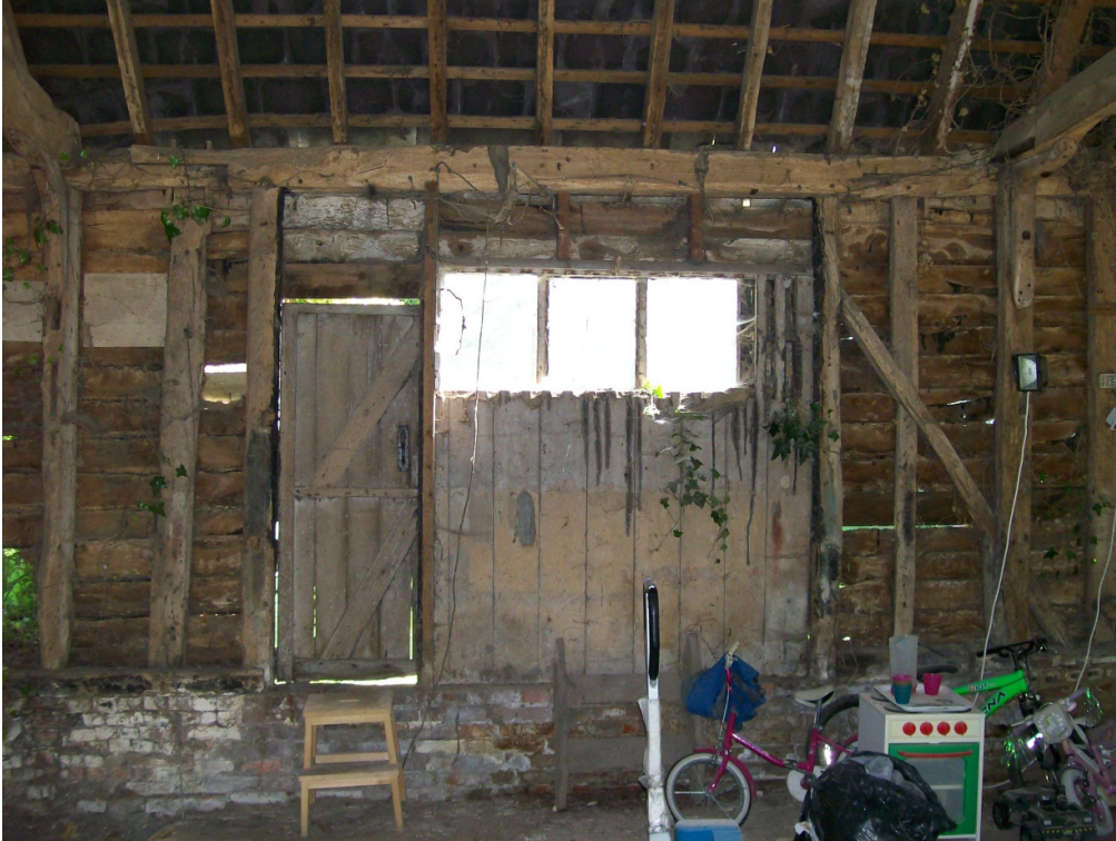
Plate 7 Bay 2, north-east wall showing inserted door and blocked midstreay opening - view north-east
