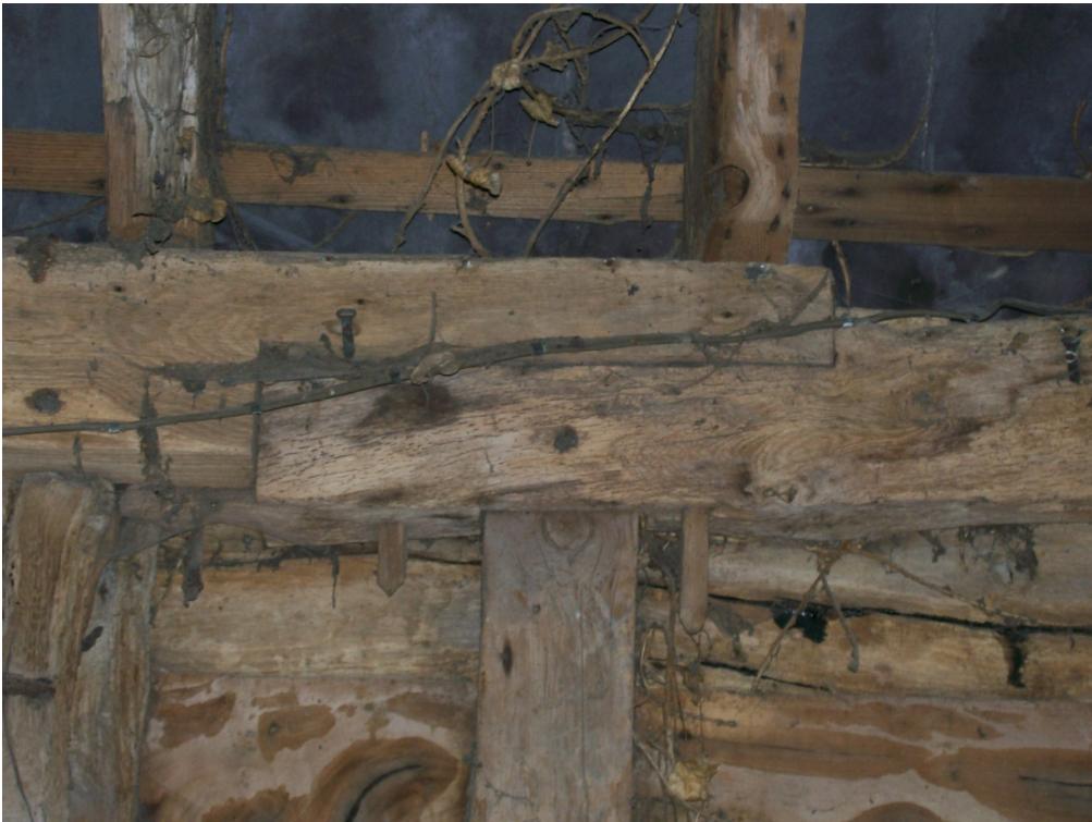
Plate 8 Bay 2, edge-halved scarf joint with untrimmed pegs - view north-east
