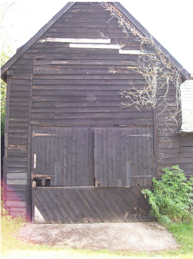
Plate 2 Midstrey showing the modern cart doors below the original opening
