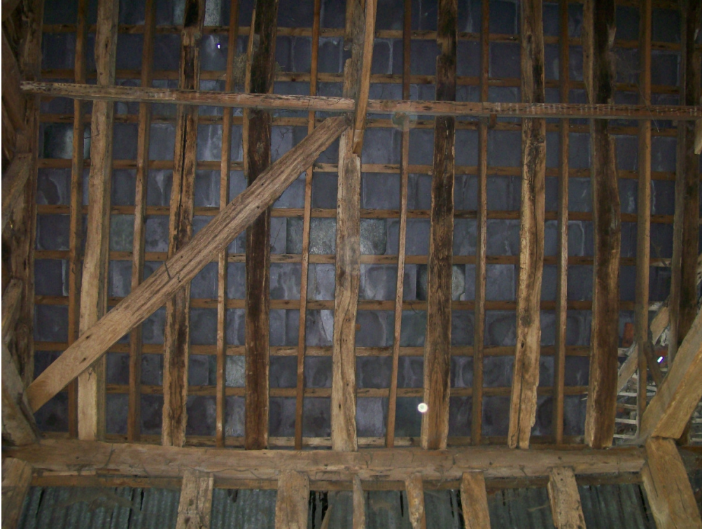
Plate 17 Midstrey roof with smoke-blackened re-used timbers
