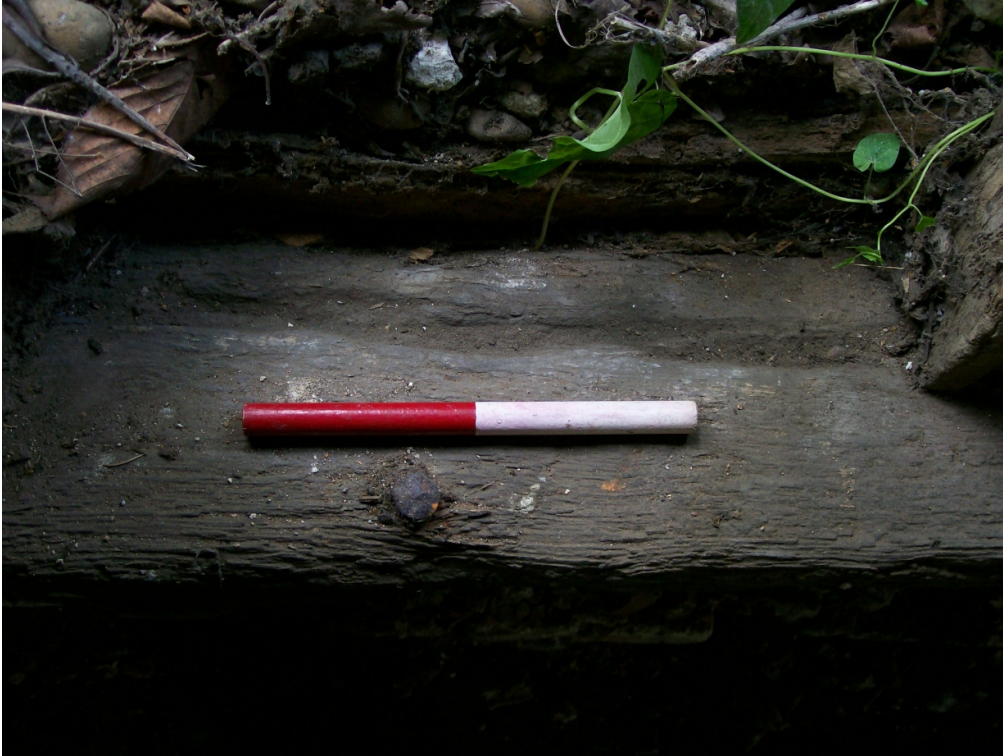
Plate 11 Bay 1, evidence for original wattle and daub stave groove in north-east sill beam
