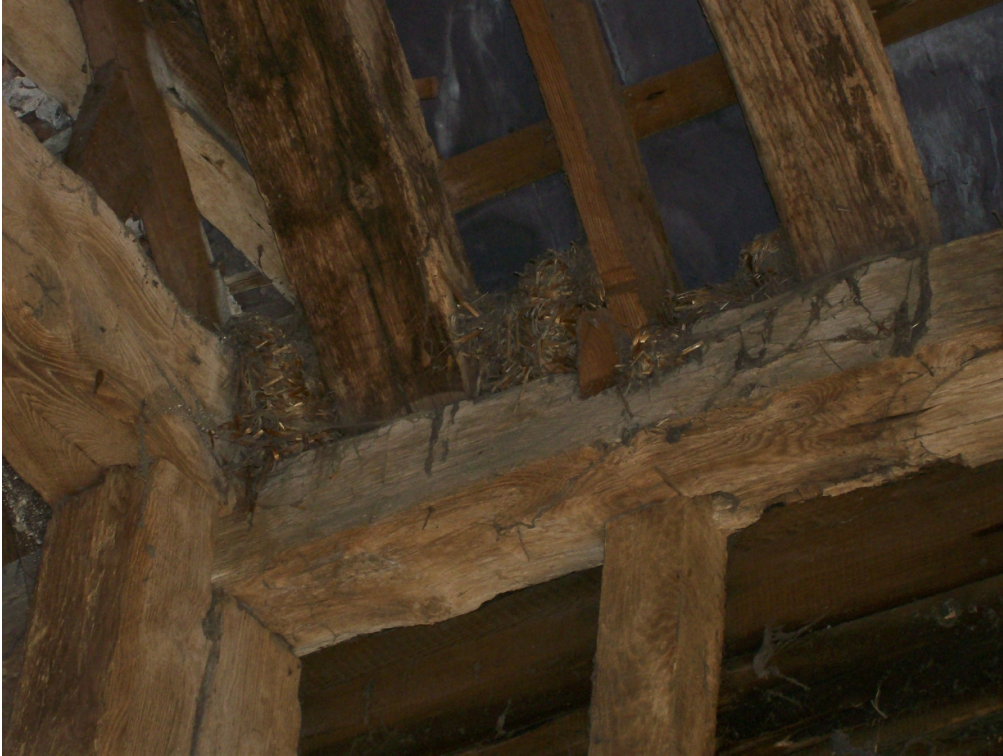
Plate 15 Remains of thatch on midstrey south-east wall plate
