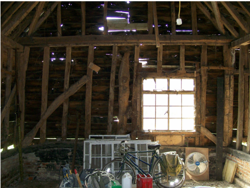
Plate 6 South-east wall frame showing curved sill beam and inserted Crittall window - view south-east
