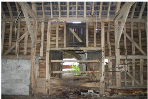
Plate 13 Barn 2a, showing jowled bases to rear barn doors, threshold leap and inserted pitching door – view south
