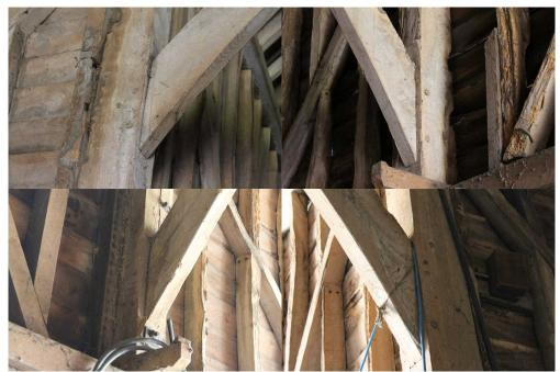
Plate 5 Carpenters' marks on posts and braces of trusses B (top) and C (bottom)
