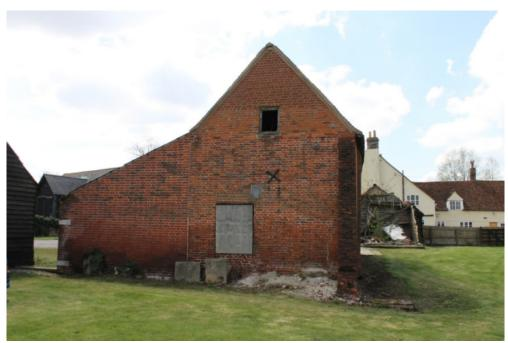
Plate 35 Stable/granary 4a, showing converted doorway, rebuilt gable and later buttress – view south-west
