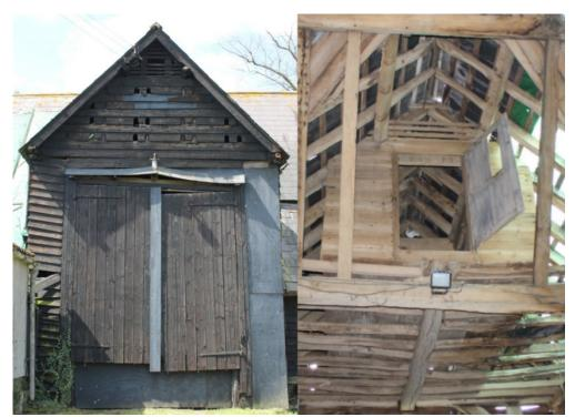
Plate 28 Barn 3a, showing exterior and interior of midstrey with pigeon loft in gable
