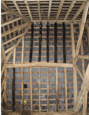
Plate 15 Barn 2a, detail of fire-blackened and reused timbers in roof of bay 1
