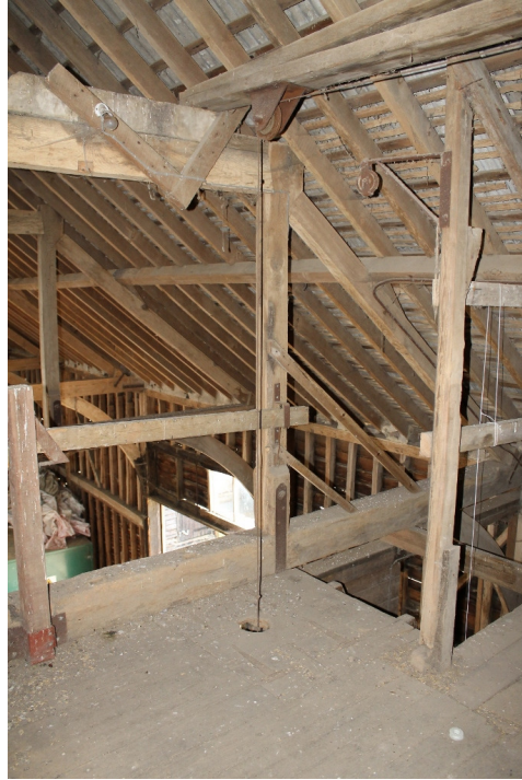
Plate 11 Second floor of the mezzanine showing grain hoist trap door and ladder to the first floor - view south-east.
