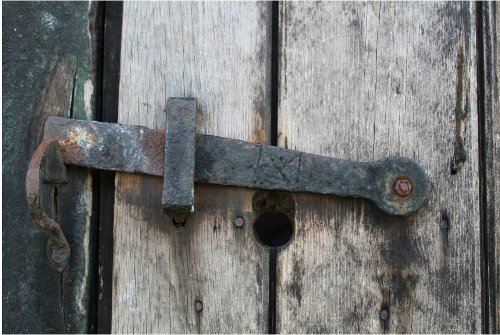
Plate 31 Detail of iron latch on door of structure 5; possibly original to the building it shares similarities (the incised (IXI)) with a carpenter's mark on a tie beam in structure 2
