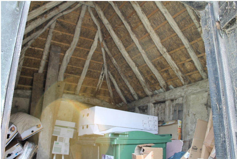
Plate 32 Interior of structure 5 – view south-east
