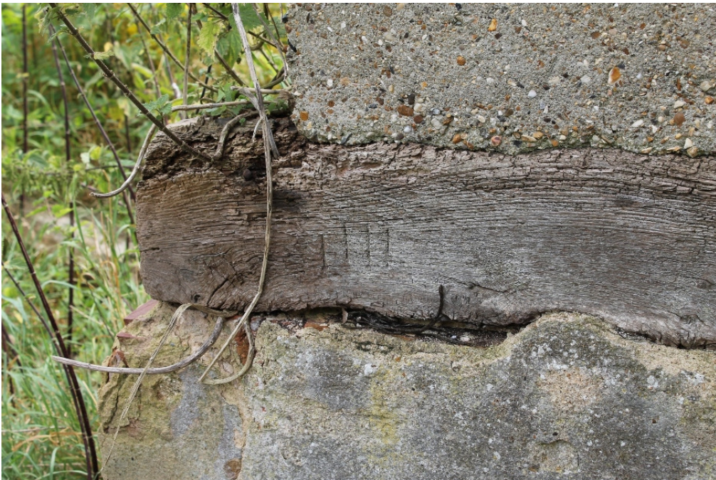
Plate 28 Structure 4, carpenter's mark (III) on aisle sill beam to bay 3/4 - view south-east
