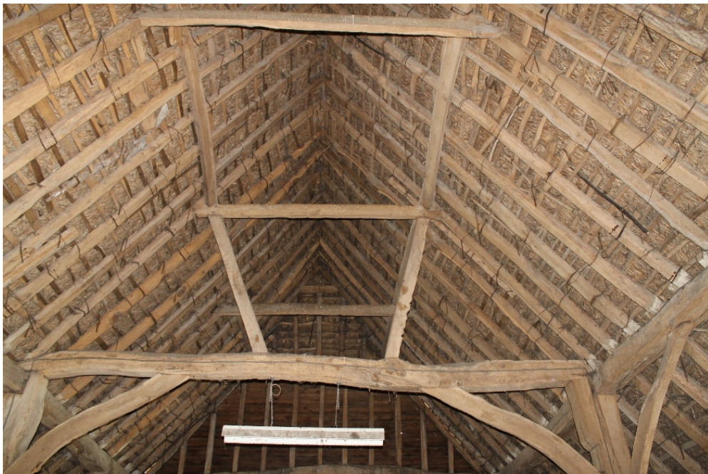
Plate 18 Structure 2, truss A of the mid-late 17th-century barn with inclined queen posts – view west
