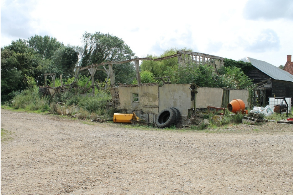
Plate 27 Structure 4, with the 19th-century extension in the foreground – view south-west
