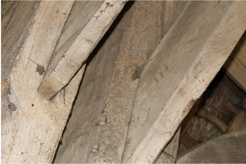
Plate 19 Carpenter's mark (III) on south arcade post and tie beam brace of truss B - view south-west
