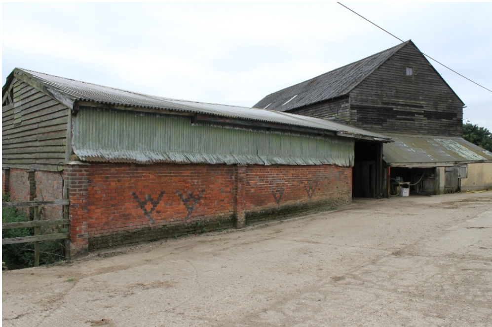
Plate 38 19th-century brick wall to structure 10 – view south-east
