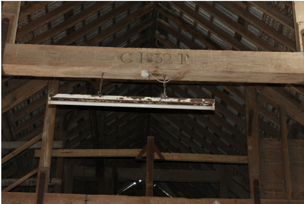
Plate 7 Structure 1, inscription "G 1832 P" on tie beam of truss C, probably commemorating the date the barn was built and the initials of the builder - view north-west.
