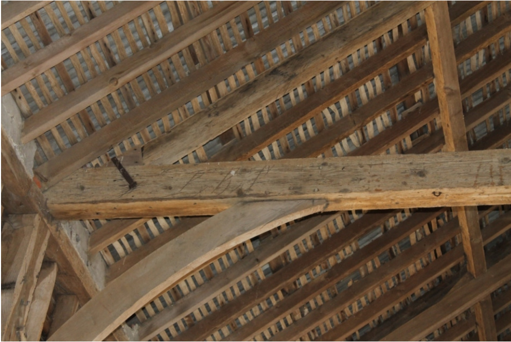
Plate 5 Baltic marks on tie beam of truss D – view west
