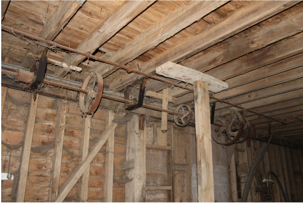
Plate 9 Structure 1, drive belt linkage in bay 1 below the mezzanine. The power was transferred from the wheels via belts passing through voids in the mezzanine floor to machinery on the first floor - view north-west.
