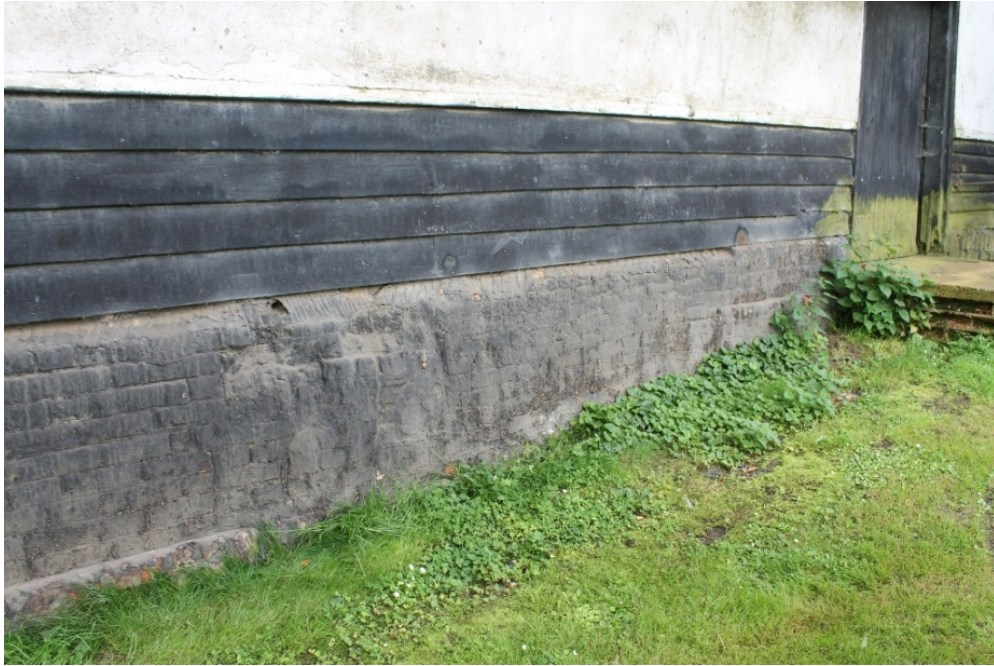
Plate 13 The brick plinth to the north elevation of structure 2, showing the change in brickwork where the original cart door entrance has been filled in - view south-west.
