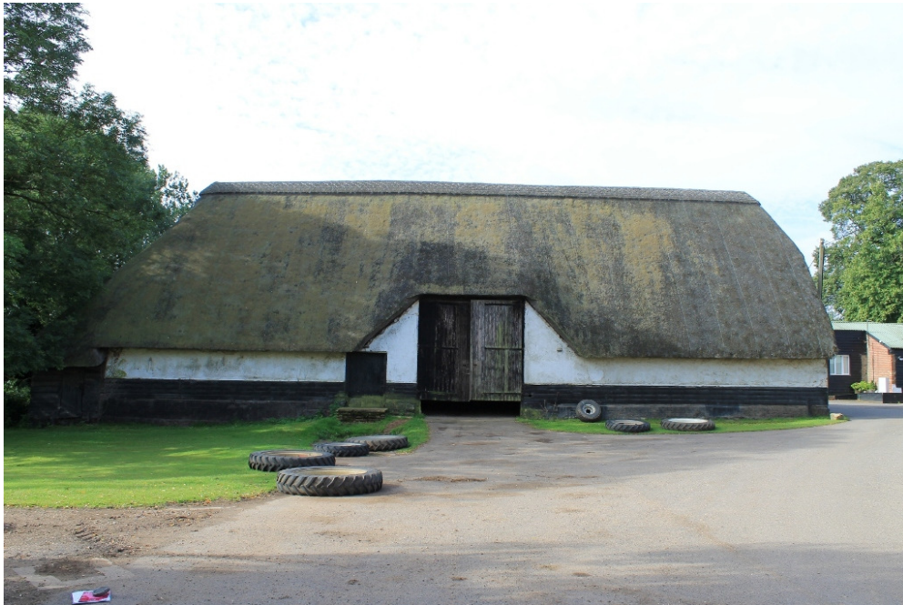
Plate 12 Structure 2, 17th-century aisled barn - view south.
