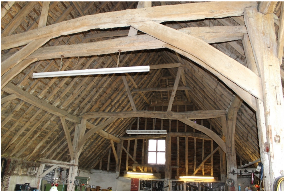
Plate 16 Abutting arcade posts to trusses of structure 2 where the early 17th-century barn joins the mid-late 17th-century barn - view west
