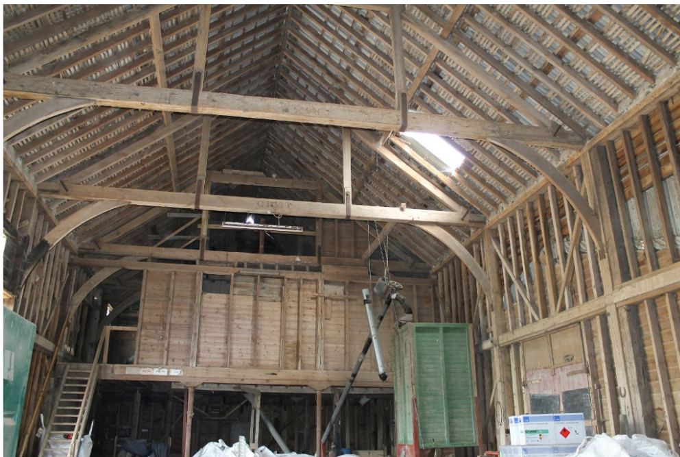
Plate 8 Mezzanine occupying bays 1 and 2 - view north-west.
