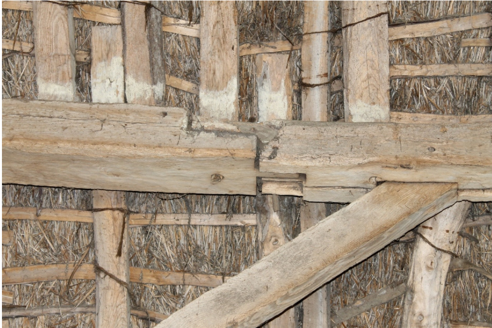
Plate 21 Edge-halved scarf joint with bladed abutments on south arcade plate of bay 3 – view south
