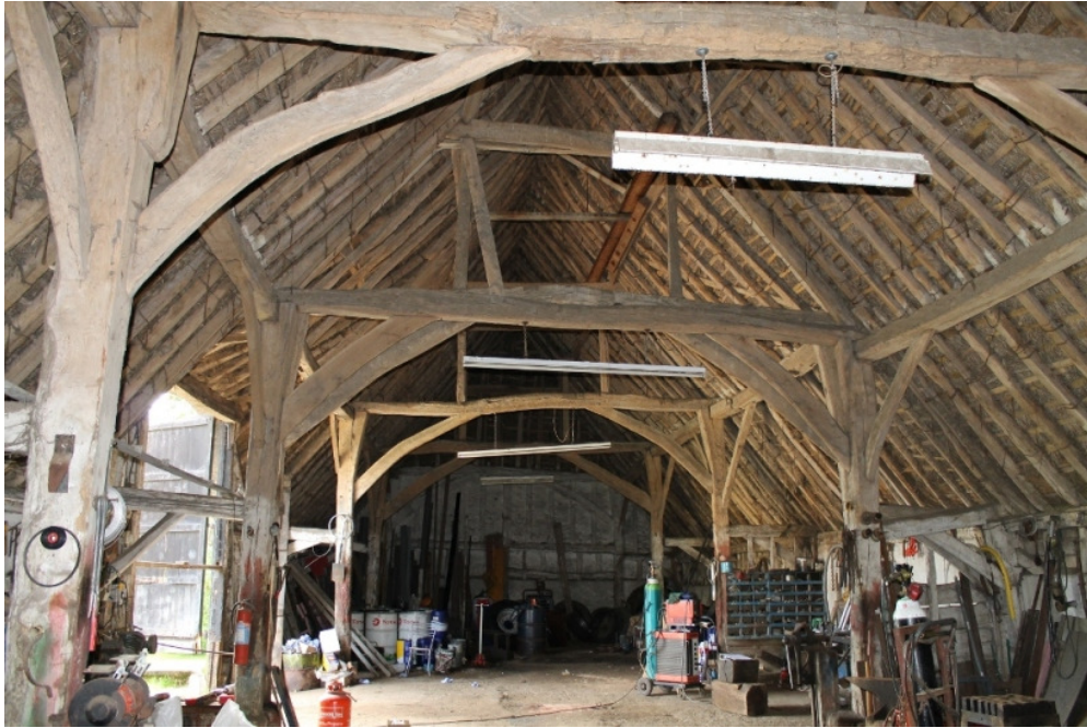
Plate 15 Interior of structure 2 – view east
