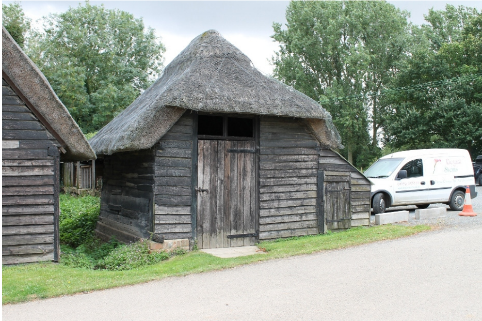
Plate 29 Structure 5, 17th-century outbuilding with 20th-century attached lean-to and structure 2 on the left – view south-east
