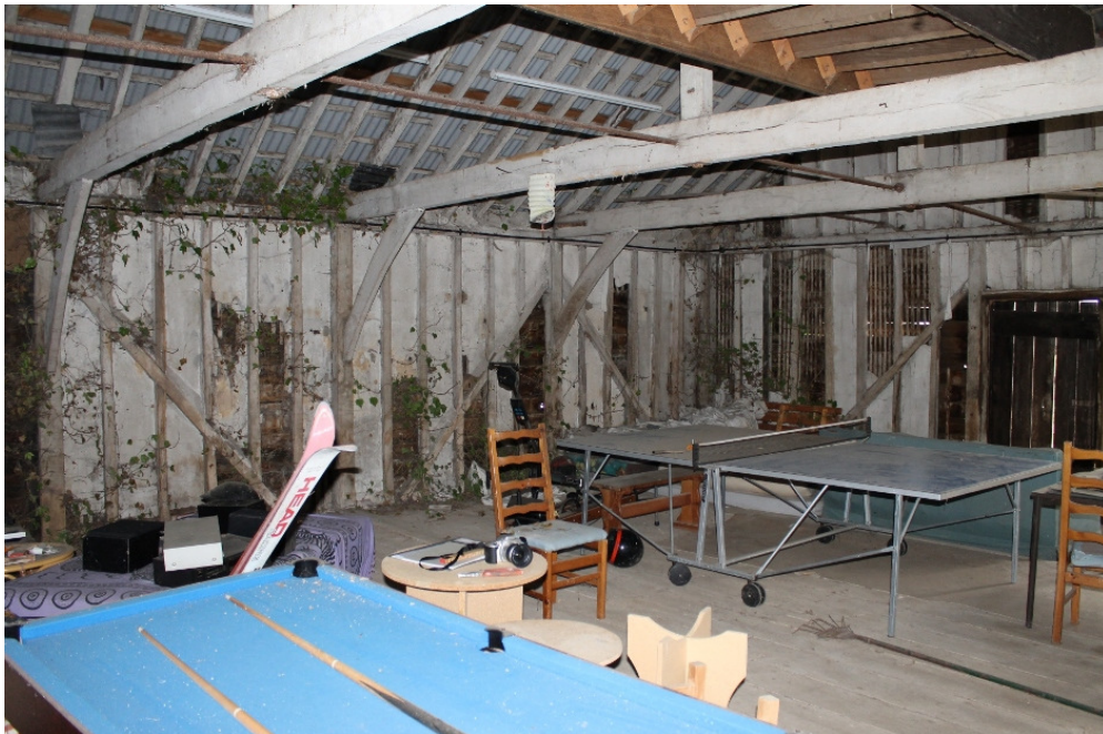
Plate 24 Interior of structure 3, 19th-century granary – view south-west
