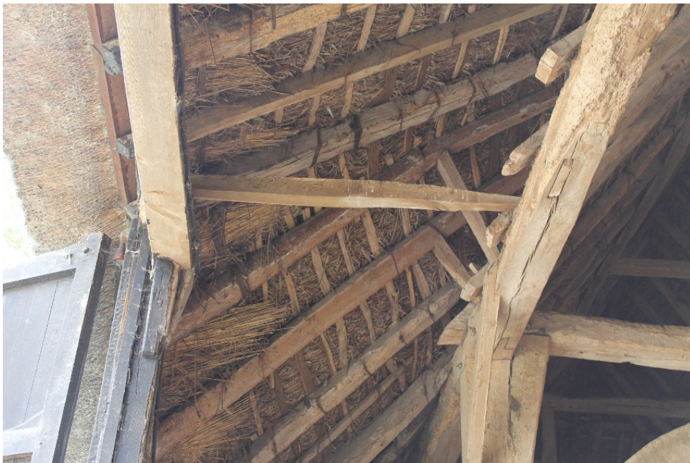
Plate 22 Re-located porch to structure 2 showing rafters ending at the arcade plate and the sawn-off ends of the brace - view east
