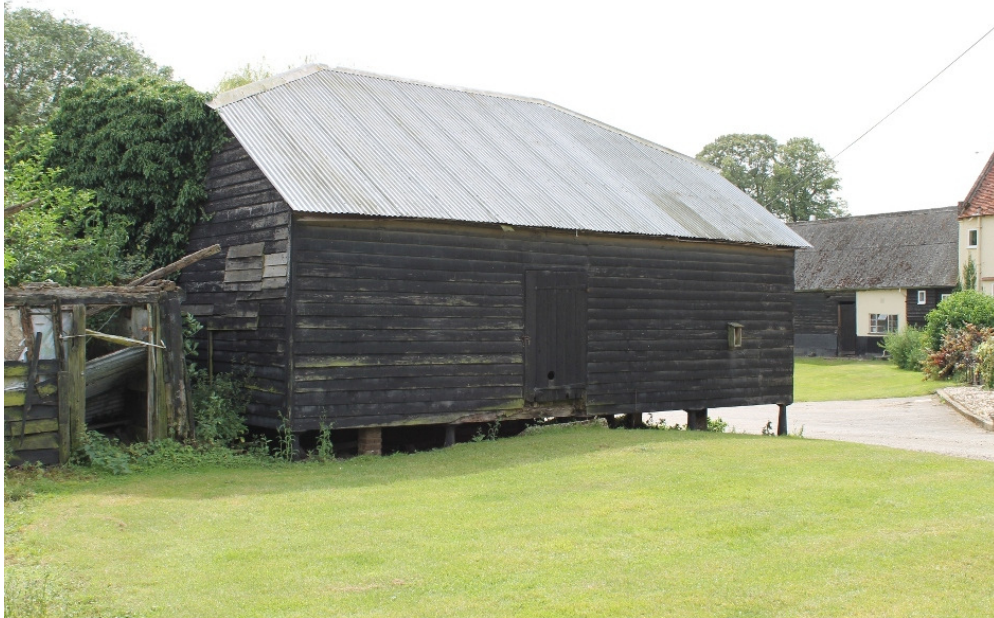
Plate 23 Structure 3, 19th-century granary - view south-west
