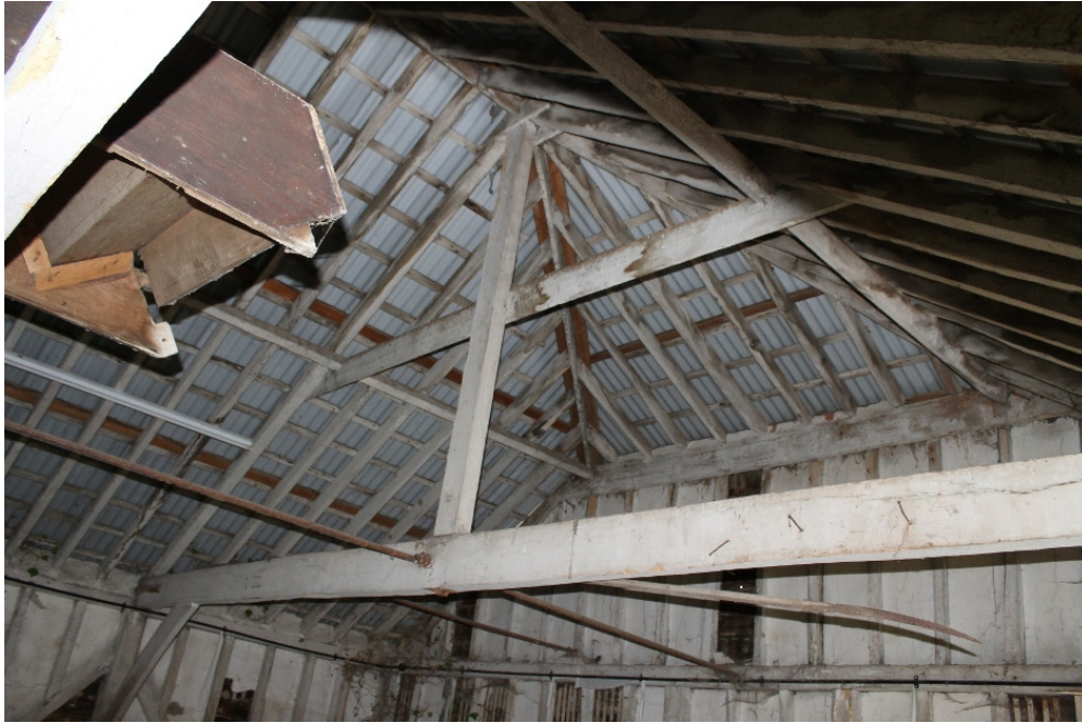
Plate 25 Structure 3, kingpost roof truss showing strengthening tie bolt and collar – view south-west
