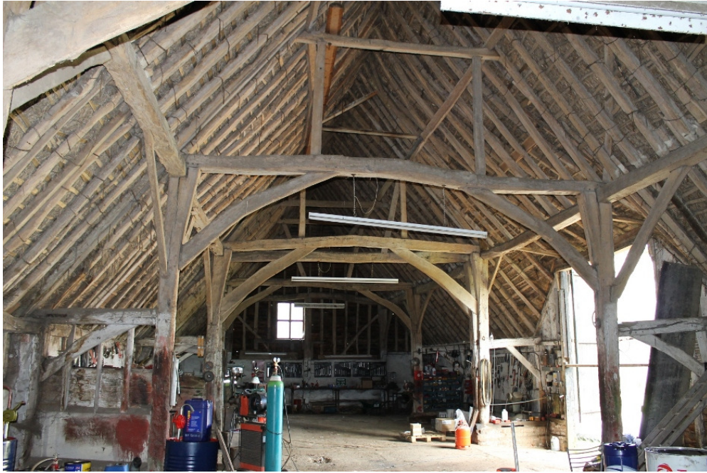
Plate 17 Structure 2, truss D of the early 17th-century barn with straight queen posts – view west
