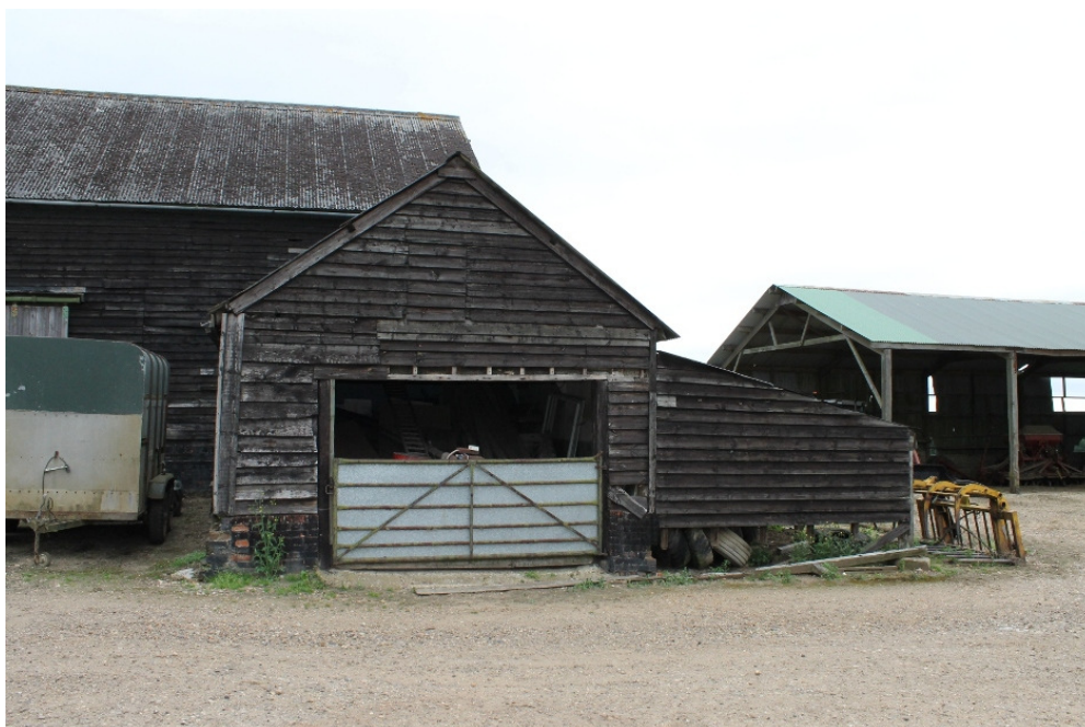
Plate 40 Structure 11, 19th-century loose box – view north-east
