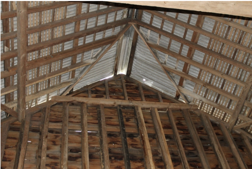
Plate 6 South-east gable of structure 1, showing the earlier half-hipped roof
