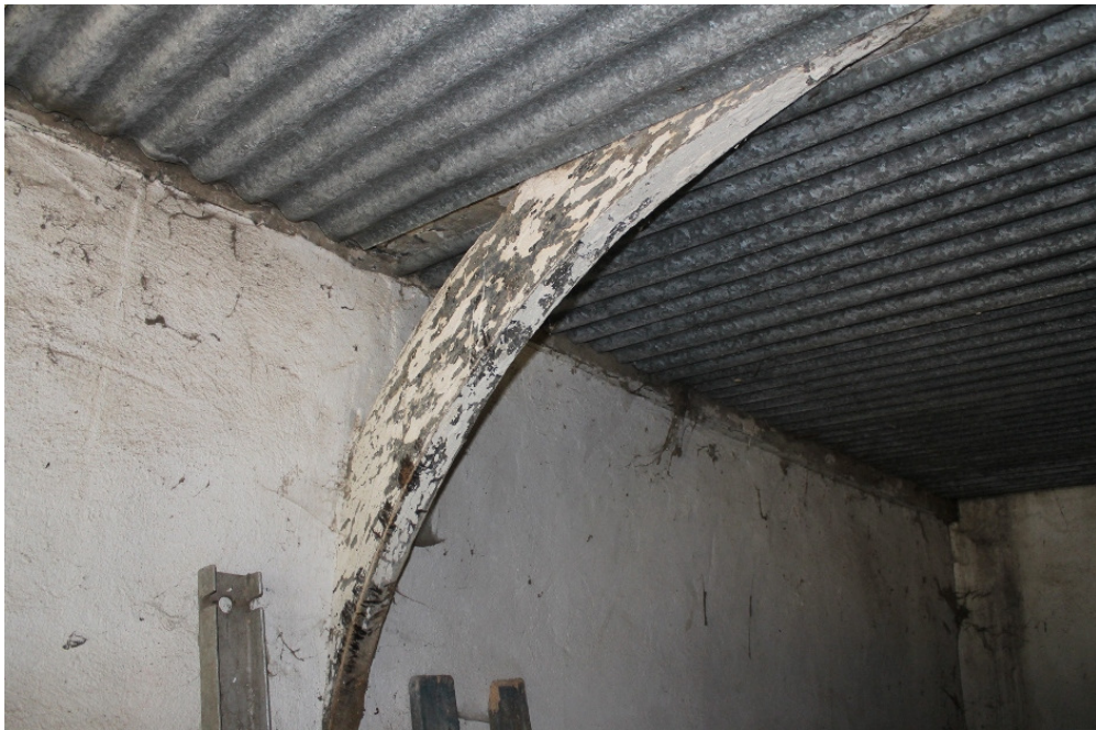
Plate 42 Interior of structure 11 showing a curved brace. The framing has been obscured by modern render and the insertion of a corrugated iron sheet ceiling - view north
