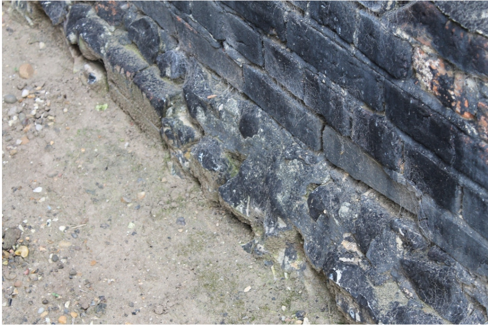
Plate 41 Flint rubble foundation to brick plinth of structure 11 – view north-east
