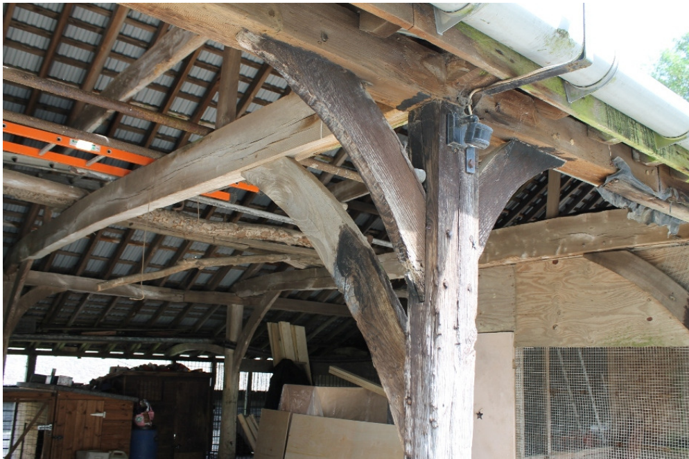
Plate 36 Structure 6, detail of bracing to south post of truss B - view east
