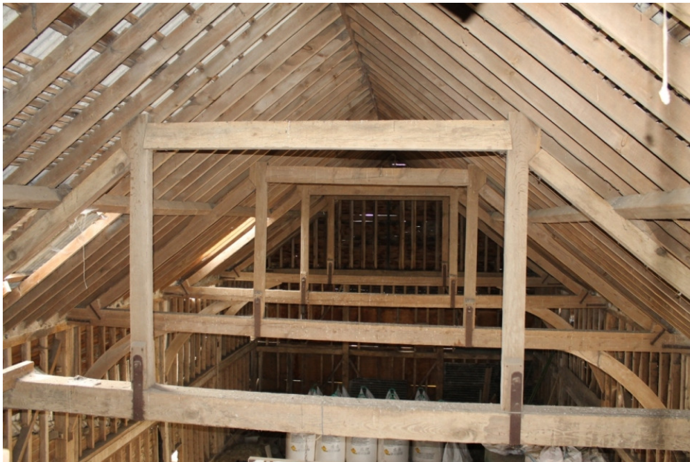
Plate 4 Interior of barn 1a showing queen post roof trusses – view south-east
