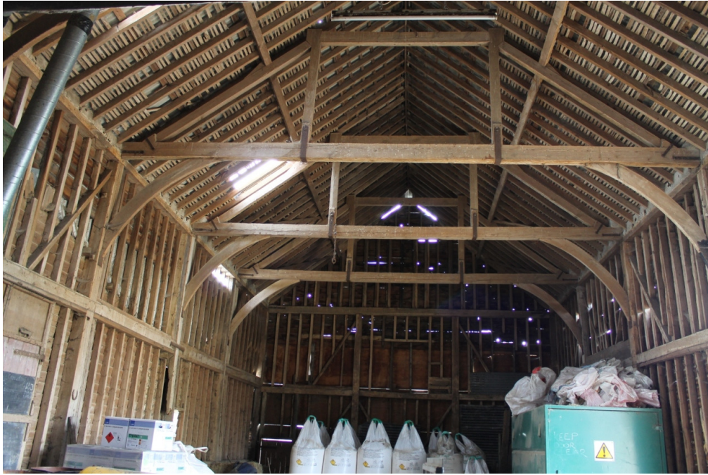
Plate 3 Interior of barn 1 – view south-east
