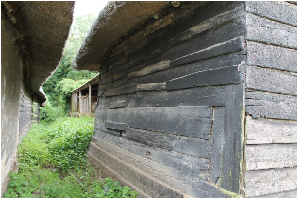
Plate 30 Structure 5, north elevation with possibly original weatherboard – view south-east
