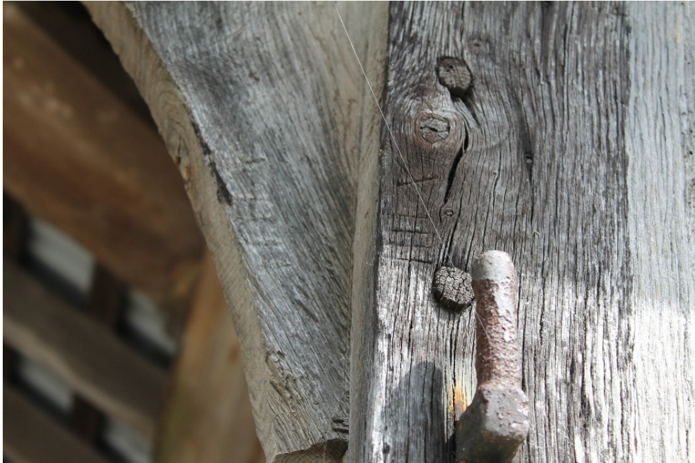
Plate 37 Detail of carpenter's marks (XIII) on the post and brace of the south-east corner – view north-east
