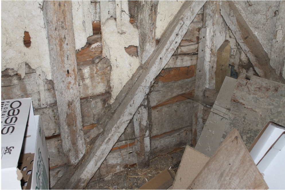
Plate 33 Primary bracing to the frame of structure 5 with the possibly original thick plank cladding attached to the exterior of the frame – view north-east
