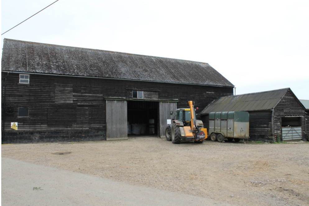
Plate 1 South-west elevation of structure 1 (19th-century barn) with structure 11 (19th-century lean-to) on the right - view north-east
