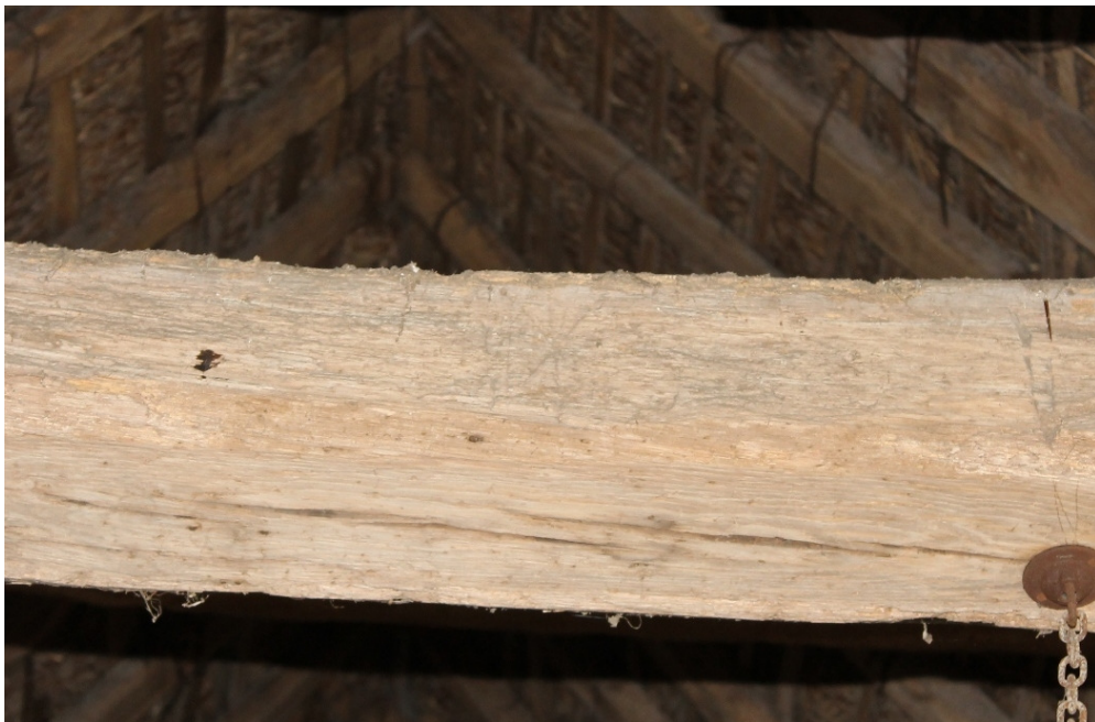
Plate 20 Unusual carpenter's mark on tie beam of truss B – view south-west
