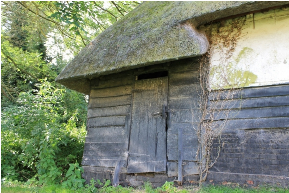
Plate 14 North elevation of the lean-to at the end of structure 2, possibly with the original weatherboard and door - view south-east
