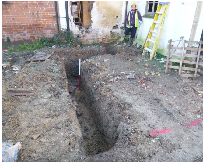
Plate 1 Hall Extension 1 General view of partly completed footing trenches (view southeast)
