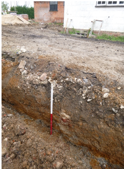
Plate 9 Brick and mortar feature F4 (beside ranging pole) in side of New boundary wall footing trench (view northeast)
