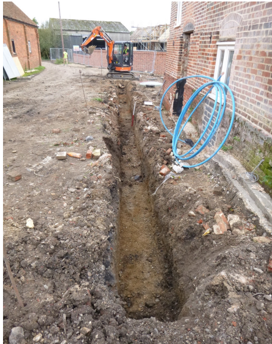
Plate 6 New boundary wall footing trench (view south)
