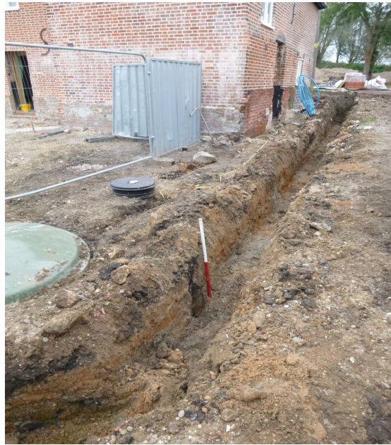
Plate 7 Post F3 showing location of post (by ranging pole) in the New boundary wall footing trench (view northwest)
