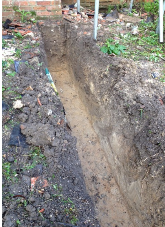
Plate 5 Hall Extension 2 view of open north footing trench (view west)
