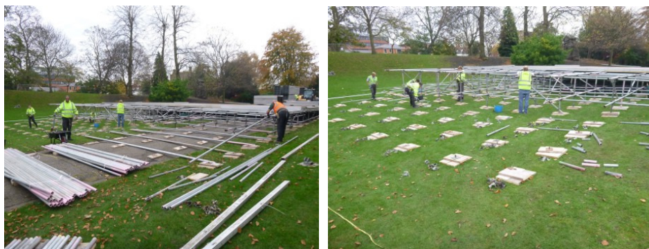
Photographs 9-10 East side of Colchester Castle during construction of raised floor for ice rink, coffee hut and skate exchange, looking SE
