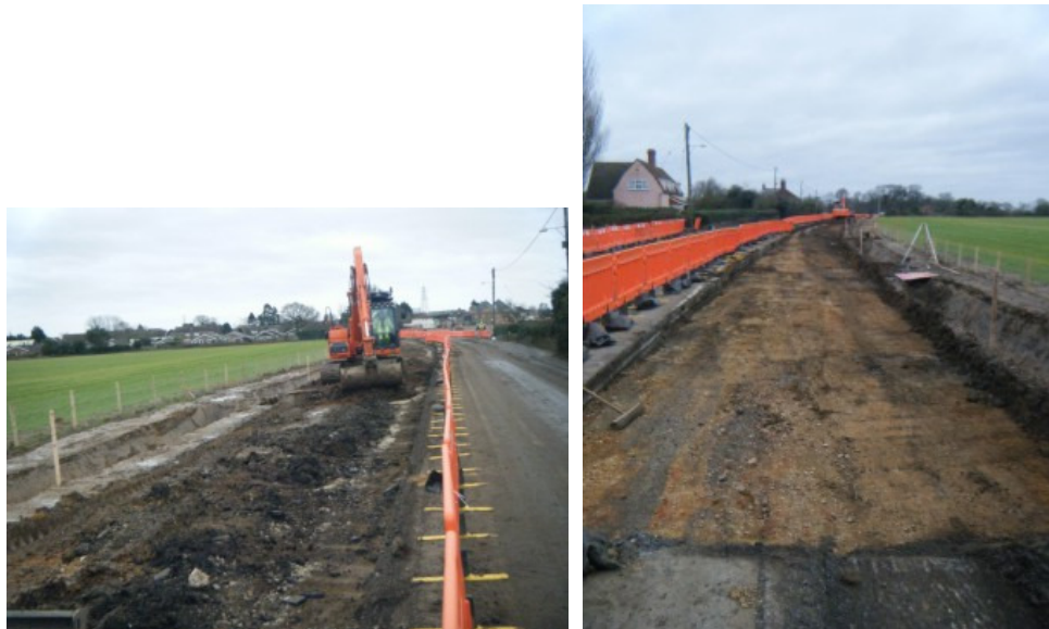
Photographs 5-6 Removal of pre-existing surface, looking S, and stripping to natural, looking N
