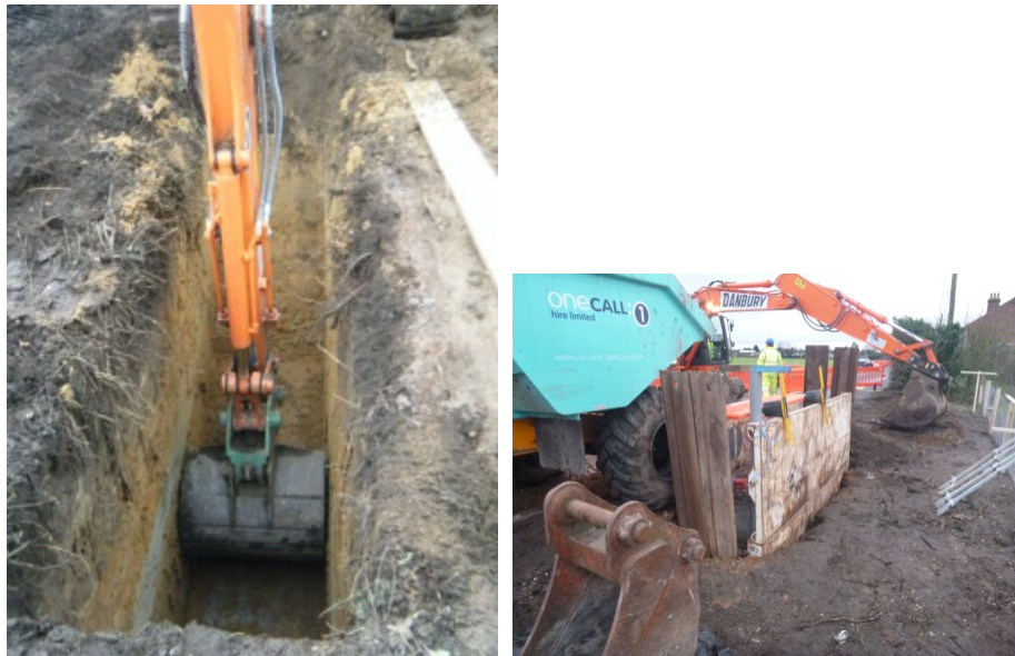
Photographs 9-10 Deep (3.2m) drainage trenches, looking N and S
