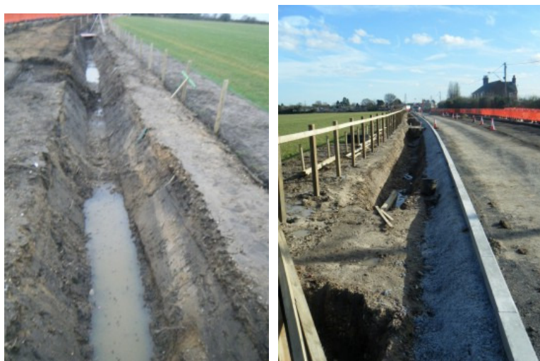
Photographs 13-14 Drainage ditch, looking S
