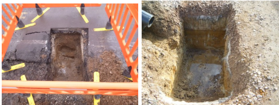
Photographs 11-12 Soakaways associated with the drainage trenches, looking W and E
