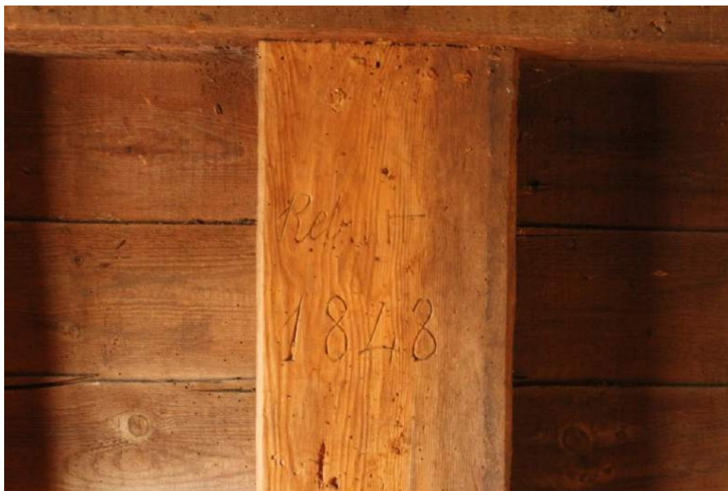
Photograph 19 "Rebuilt 1848" carved into a post of the lucam on the second floor.
