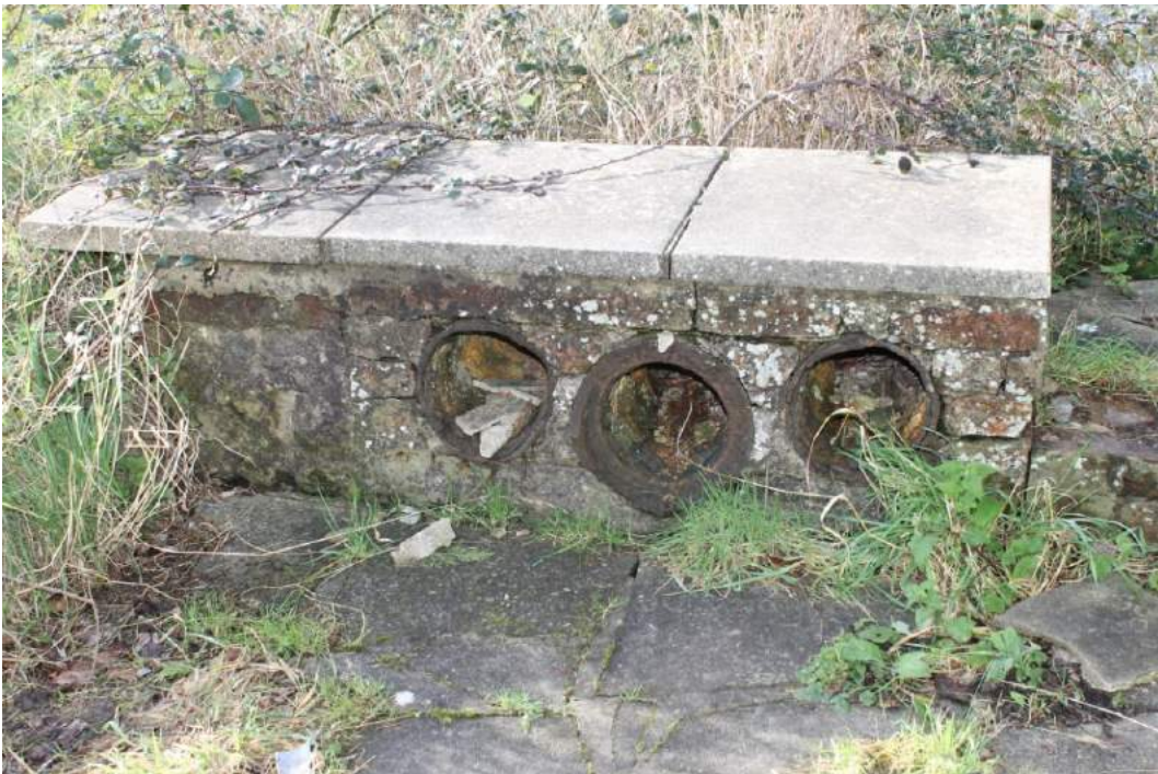
Photograph 6 Detail of iron pipes funnelling water from the mill pond to the overshot wheel - view south-west.
