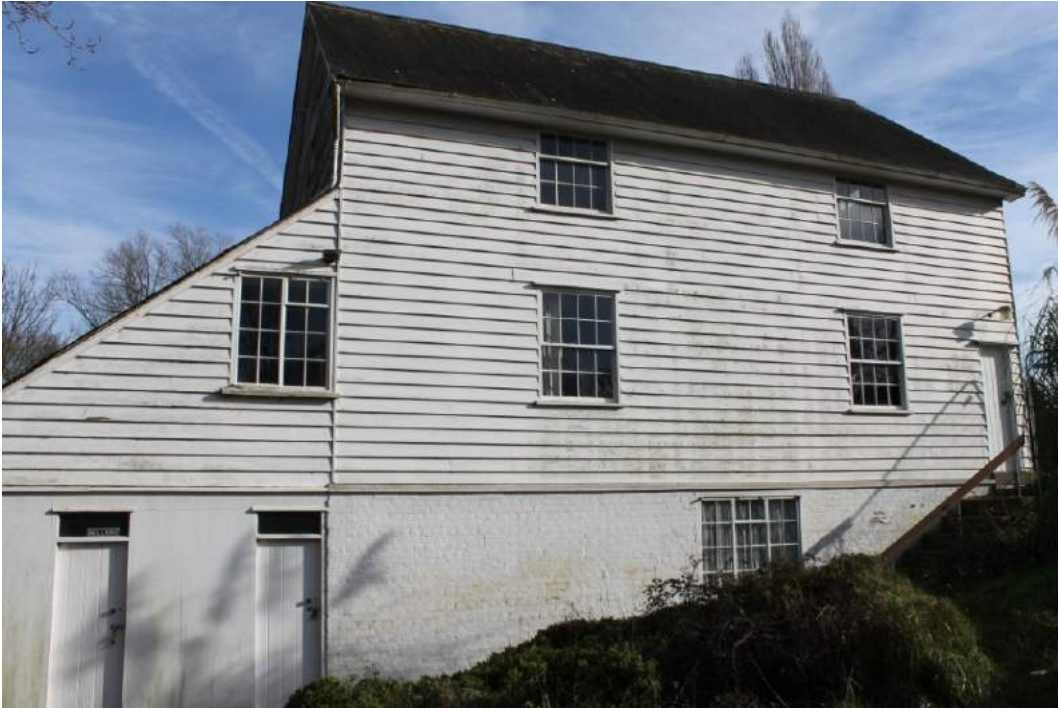
Photograph 3 South-west elevation - view east.
