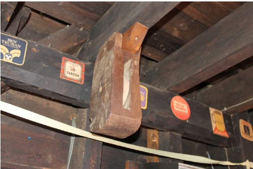
Photograph 10 Original pulley wheel from milling apparatus, relocated to underside of the replacement floor joists in the first floor.
