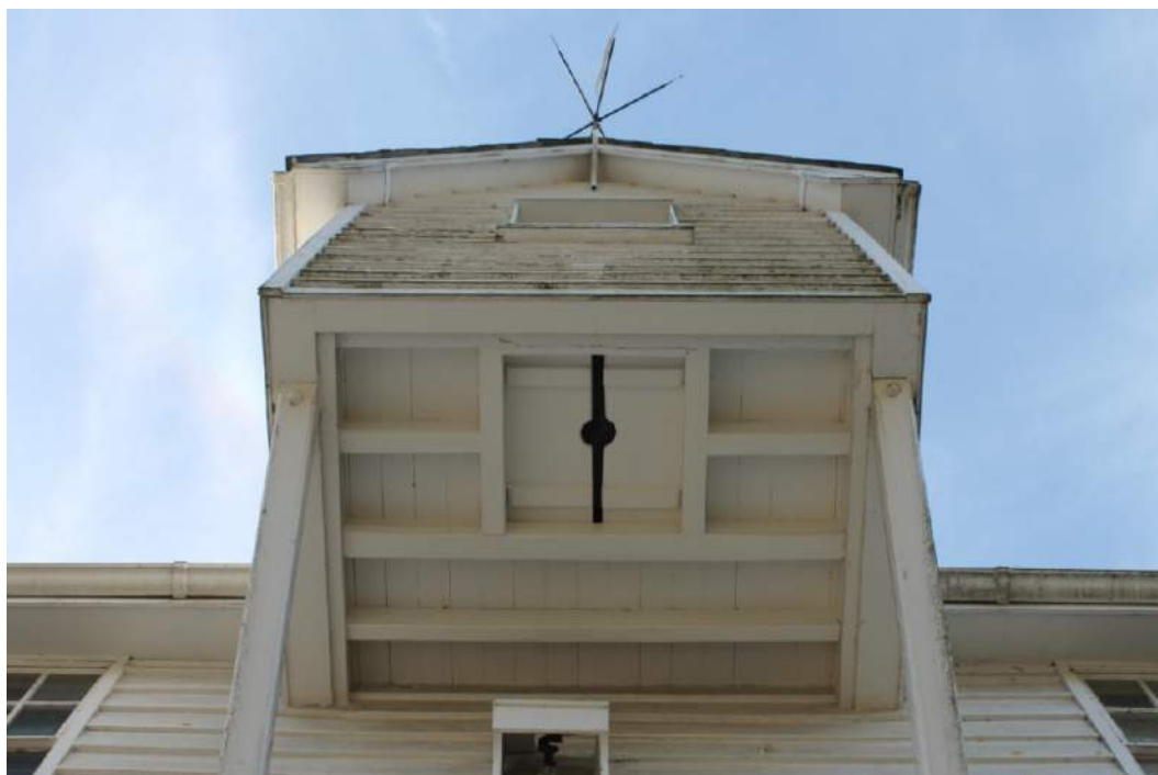
Photograph 15 Underside of the lucam showing the trap doors for the sack hoist.
