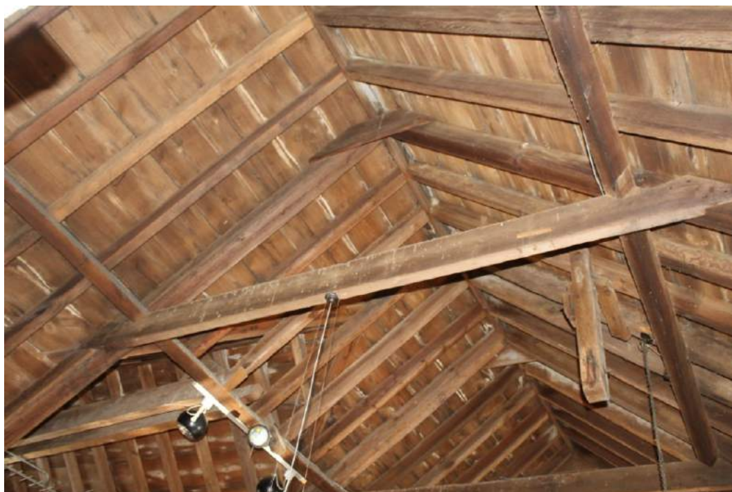
Photograph 17 Roof arrangement showing the single purlin to either pitch and the trenced collar supporting the common rafters on which sarking boards are lain.
