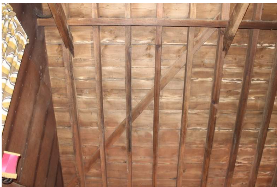
Photograph 18 Wind brace in the outer bay of the roof.
