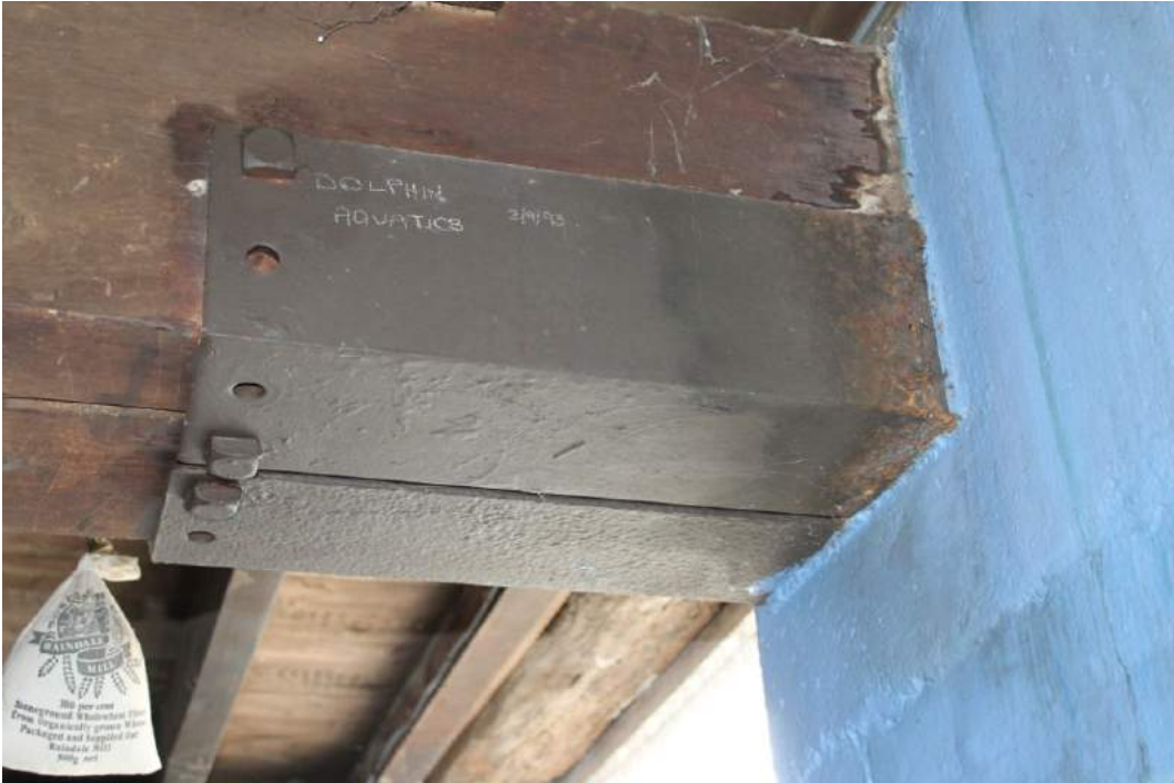
Photograph 5 Chalked date on iron brace at south-west end of bridging beam which suggests a date for the renovation of the mill.
