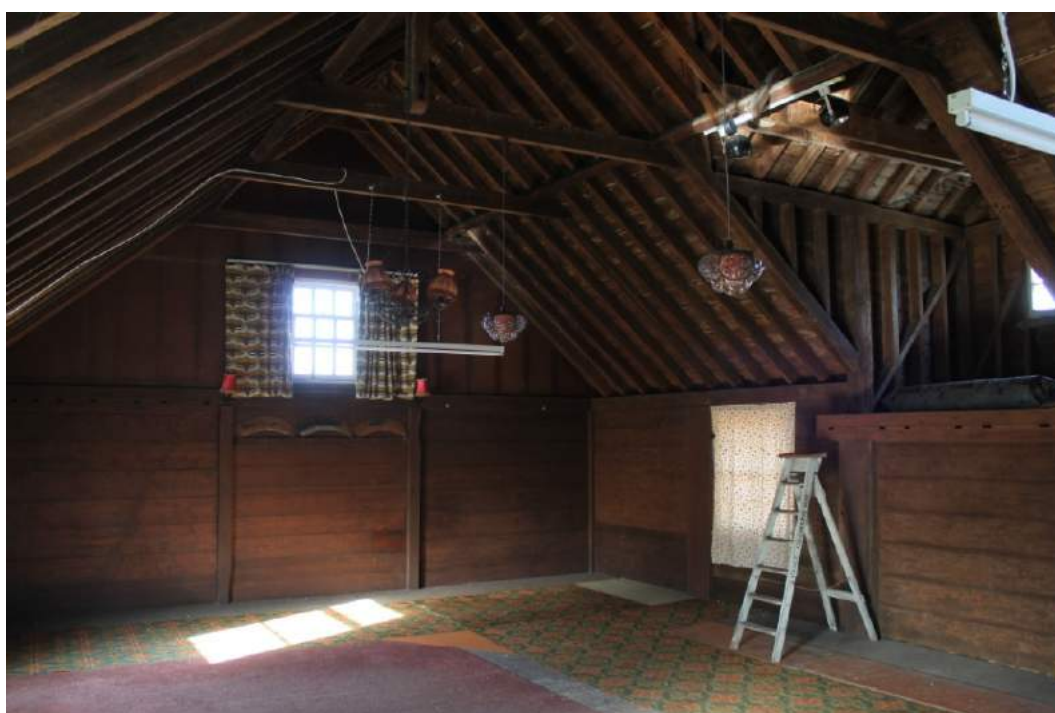
Photograph 16 Interior of the second floor with original horizontal tongue and groove boarding and the lucam to the right – view north.
