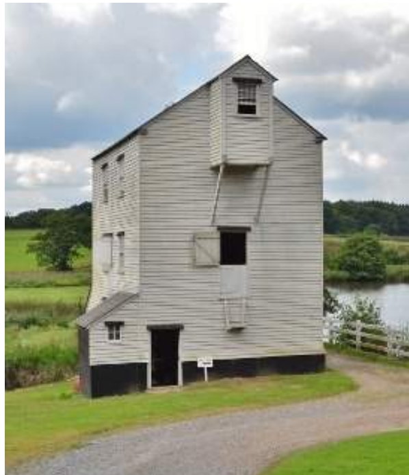
Photograph 26 Thorrington Tide Mill has a brick built ground floor and upper timber-framed storeys clad in weatherboard, a lucam, outward-opening first floor loading door and similar sized sash windows (photograph by Ashley Dace).
