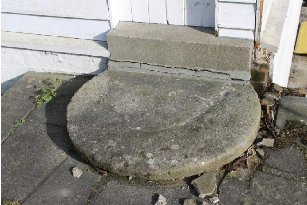
Photograph 7 Mill stone re-used as door step for inserted entrance in first floor of south-west elevation – view north-east.
