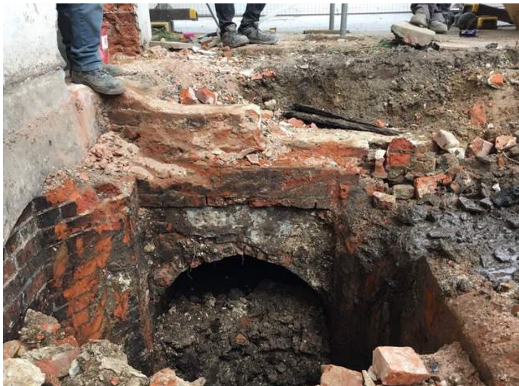
Photograph 29 Wheel pit exposed by contractor during groundworks, showing the culvert taking water below Old heath Road to Distillery Pond – view north-east.
