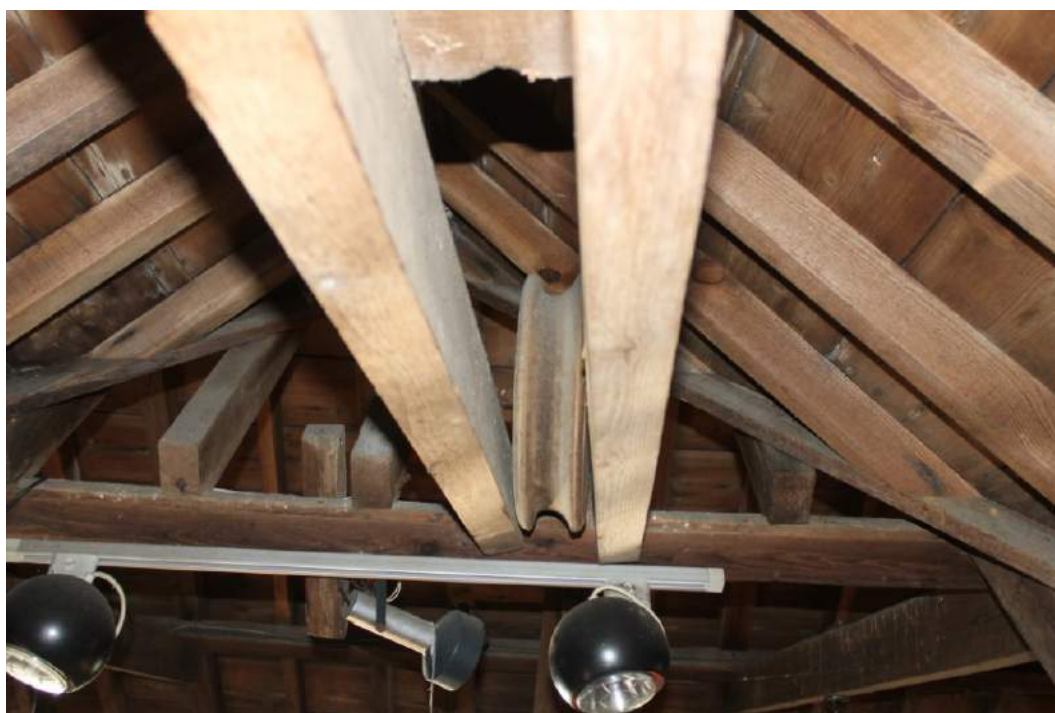
Photograph 20 Mechanism for grain sack hoist in lucam of second floor.
