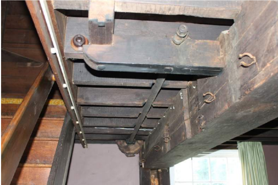
Photograph 11 Original fly wheel and drive shaft, possibly in original location but more likely positioned after 20th-century renovations - view south-west.
