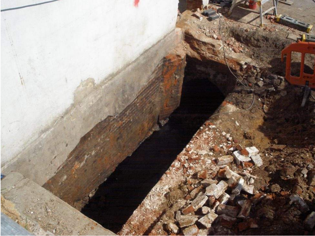
Photograph 27 Wheel pit fully excavated by contractor during groundworks – view north.
