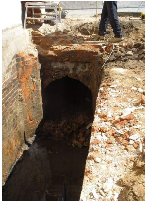
Photograph 28 Wheel pit fully excavated, with culvert taking water below Old Heath Road to Distillery Pond – view north-east.
