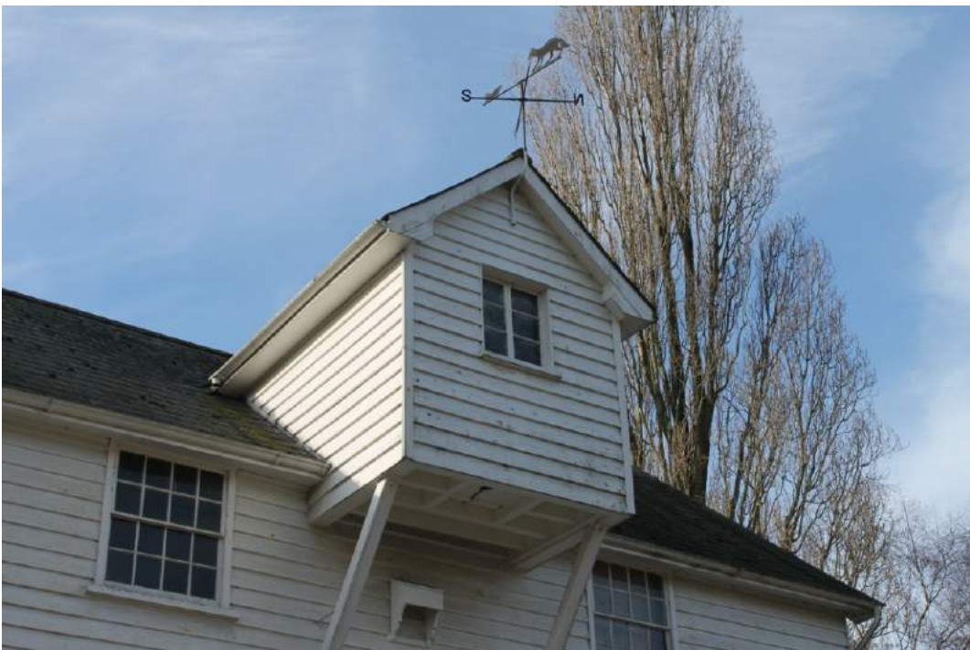
Photograph 14 Lucam for hoisting grain sacks into the second floor – view west.
