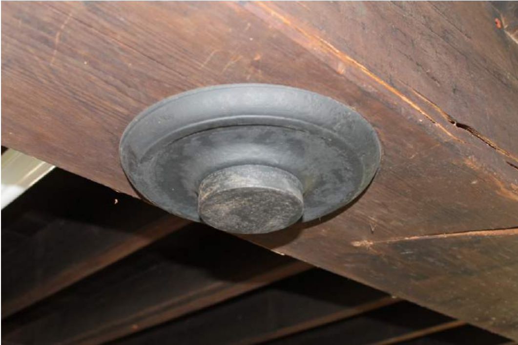
Photograph 13 Iron boss in the underside of the centre of the bridging beams to the second floor.
