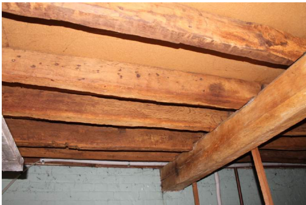
Photograph 21 Re-used timbers supporting the first floor of the 20th-century extension.
