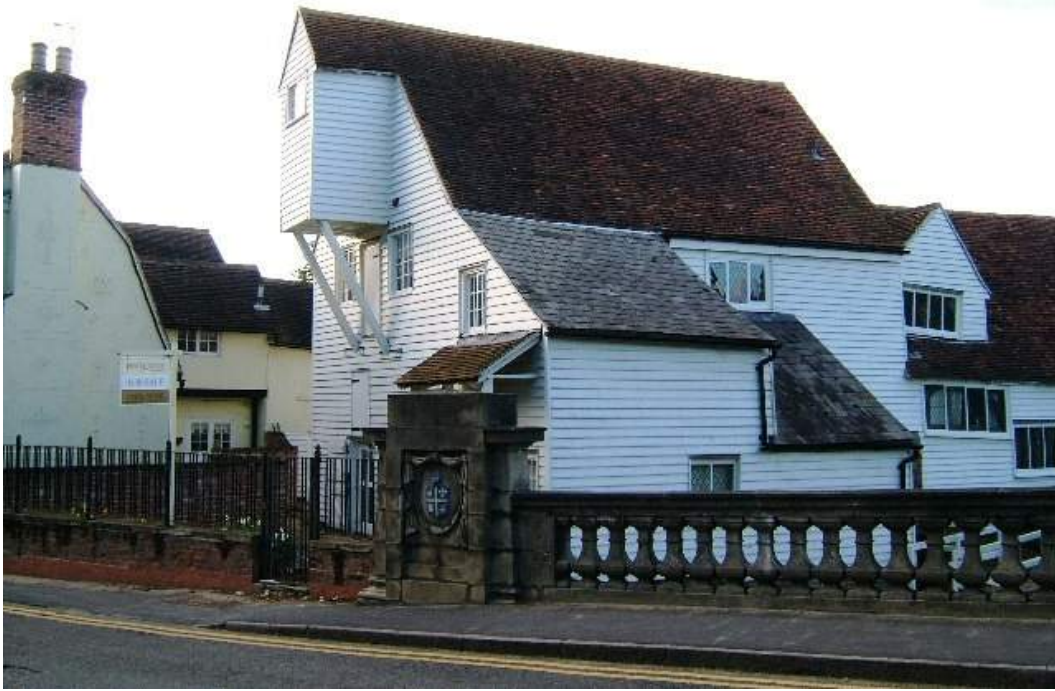
Photograph 25 Bradfordstreet mill, Bocking also has a weatherboarded timber frame with lucam, outward-opening first floor loading door and small sash windows (photograph by Brenda Howard).
