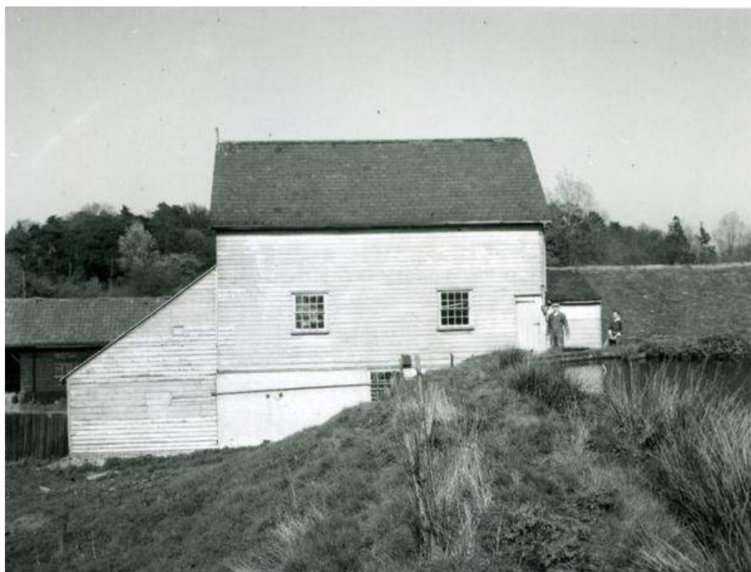
Plate 1 Photograph of the south-west (rear) elevation of Cannock Mill taken by E M Gardner in 1952
