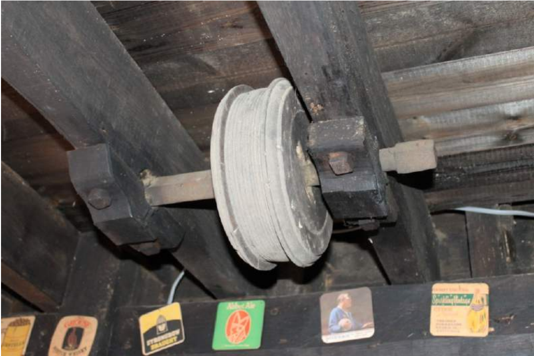
Photograph 9 Original fly wheel from milling apparatus, relocated to underside of the replacement floor joists in the first floor.
