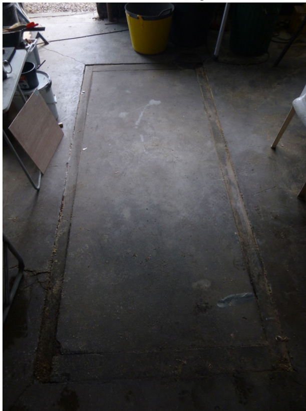
Photograph 12 Backfilled and concreted over inspection pit in main building – shot taken facing east.
