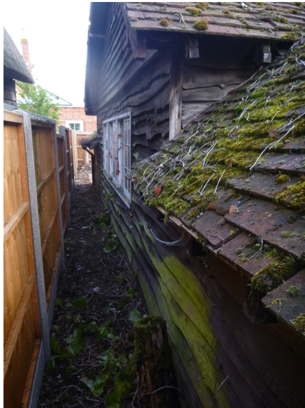
Photograph 4 West elevation – shot taken facing north.
