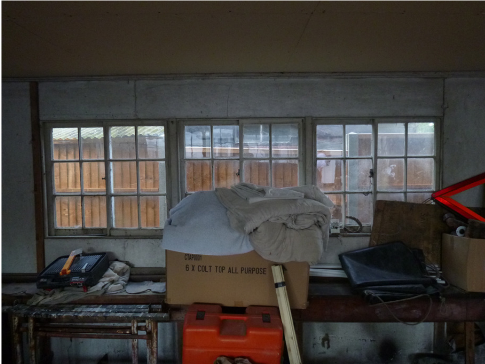
Photograph 7 Interior shot of three sliding casement windows on west elevation – shot taken facing west.
