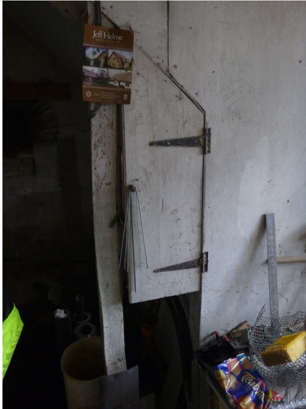
Photograph 11 Hatch in-between wall and supporting post in north wing – shot taken facing north.
