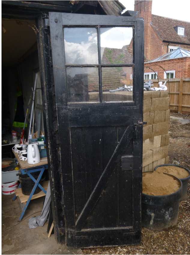
Photograph 13 Detail of single width door on east elevation – shot taken facing north-west.
