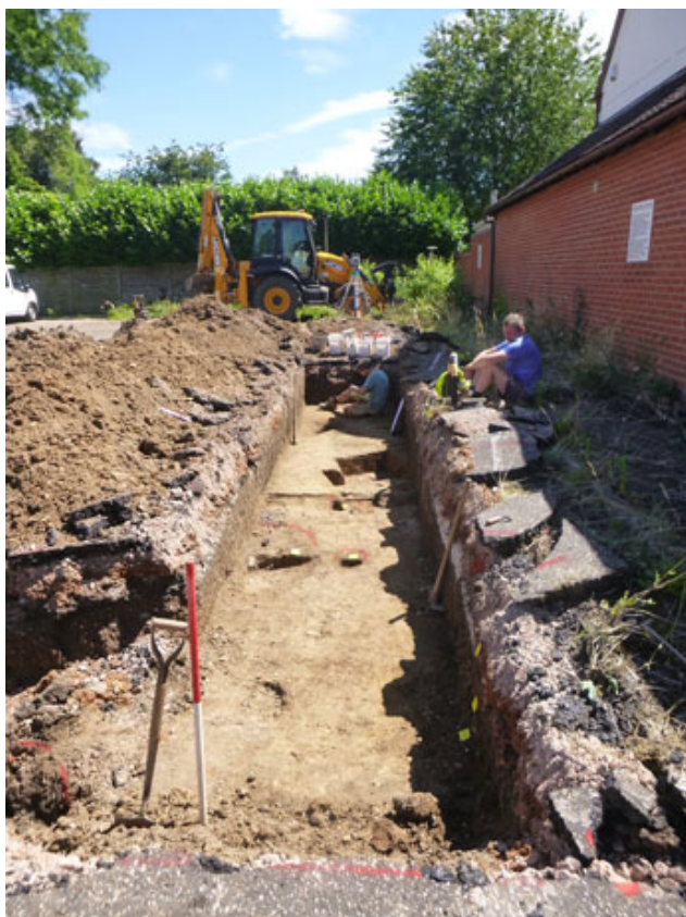
Photograph 1 Trench shot, looking SE
