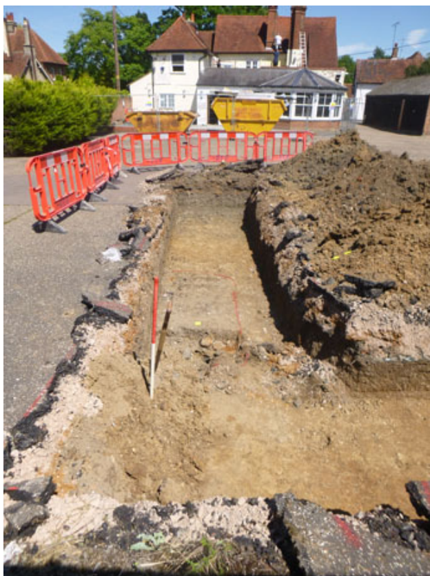
Photograph 2 Trench shot, looking NE
