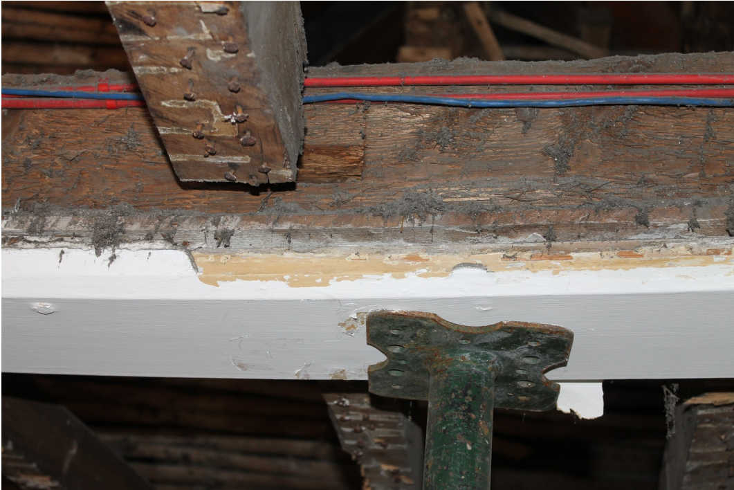
Photograph 7 Staggered mortises for the 19th-century ceiling joists in the bridging beam – view west
