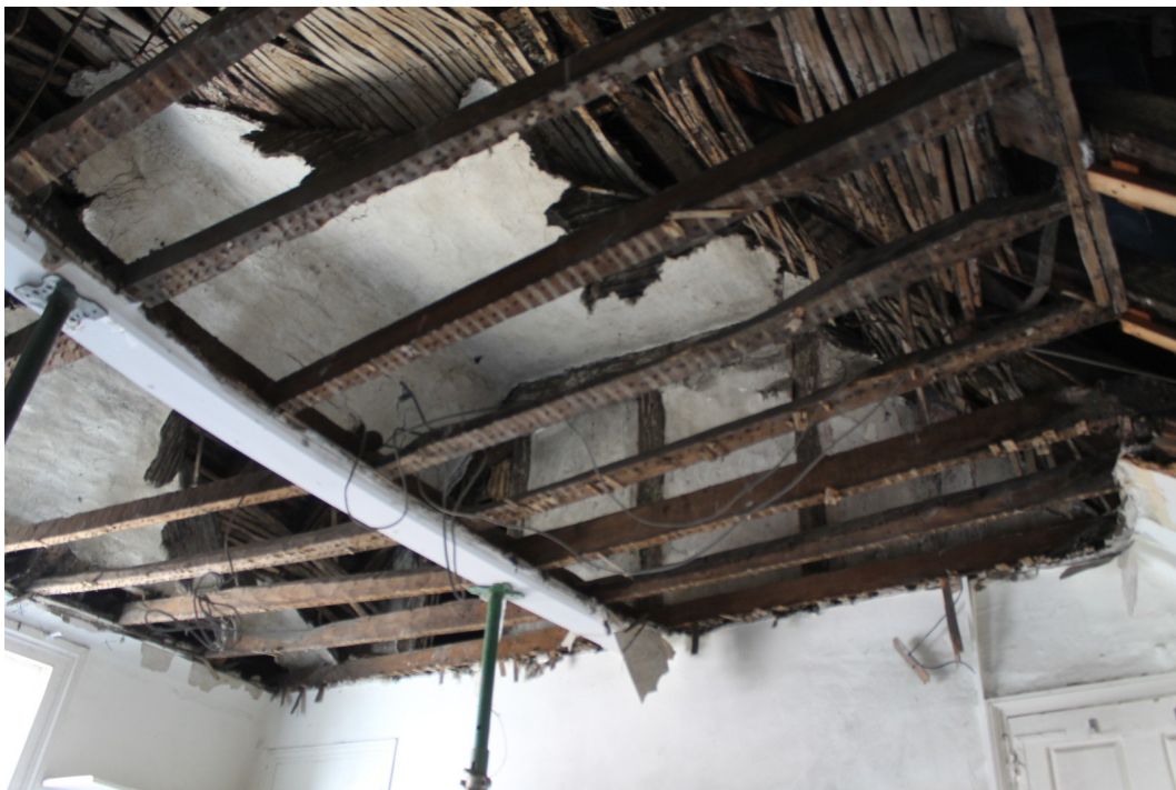
Photograph 6 Exposed ceiling joists with earlier lath and plaster ceiling above – view south-east
