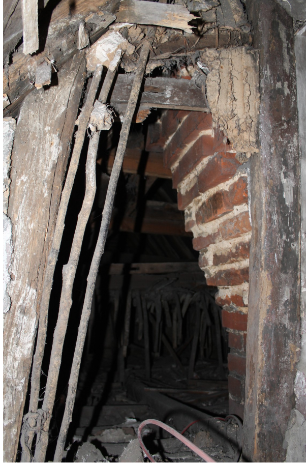
Photograph 12 Cross frame with the remains of one of the original wattle and daub infill panels – view south
