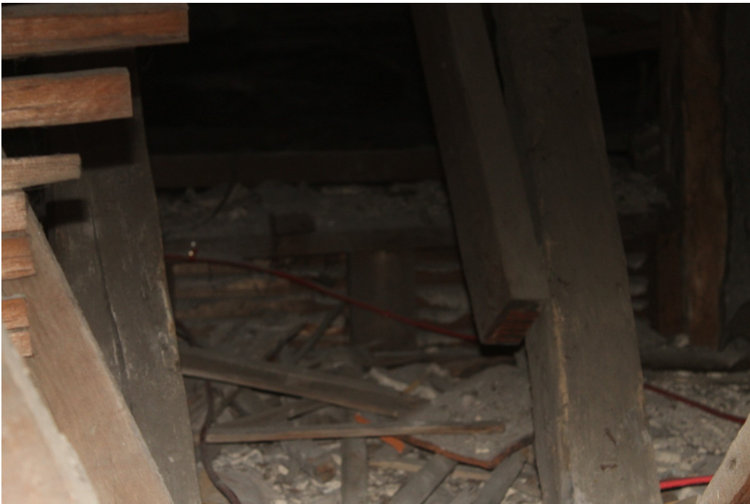
Photograph 5 Interior of roof space showing debris from earlier ceiling on top of existing ceiling – view east
