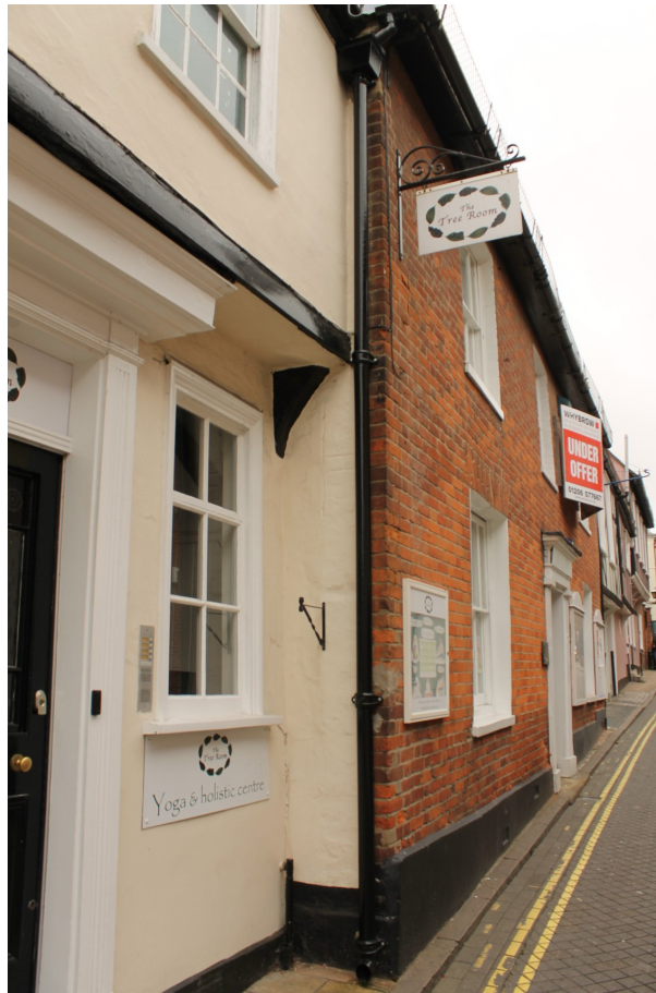
Photograph 2 Brick facing to No. 11 with the jettied first floor of No. 12 showing what is concealed by the brick facing – view north-west
