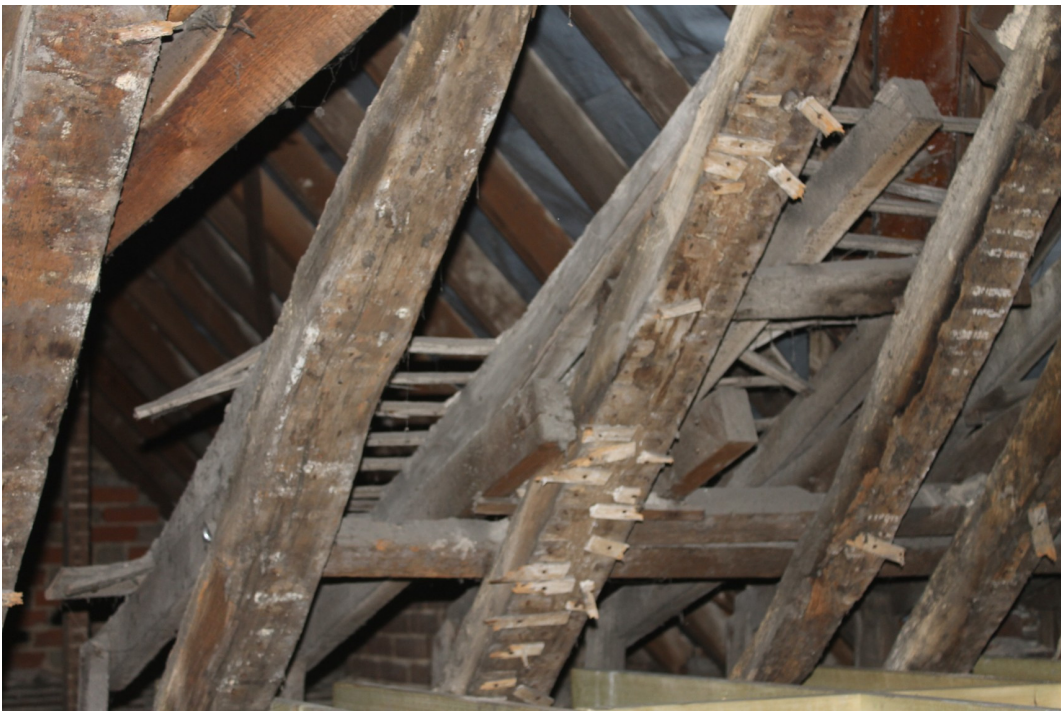
Photograph 16 Longer sprockets at the feet of the rear side rafters, allowing the roof to flare out over the possible earlier 19th-century extension, with the machine-cut timbers of the 19th-century extension behind – view north-west
