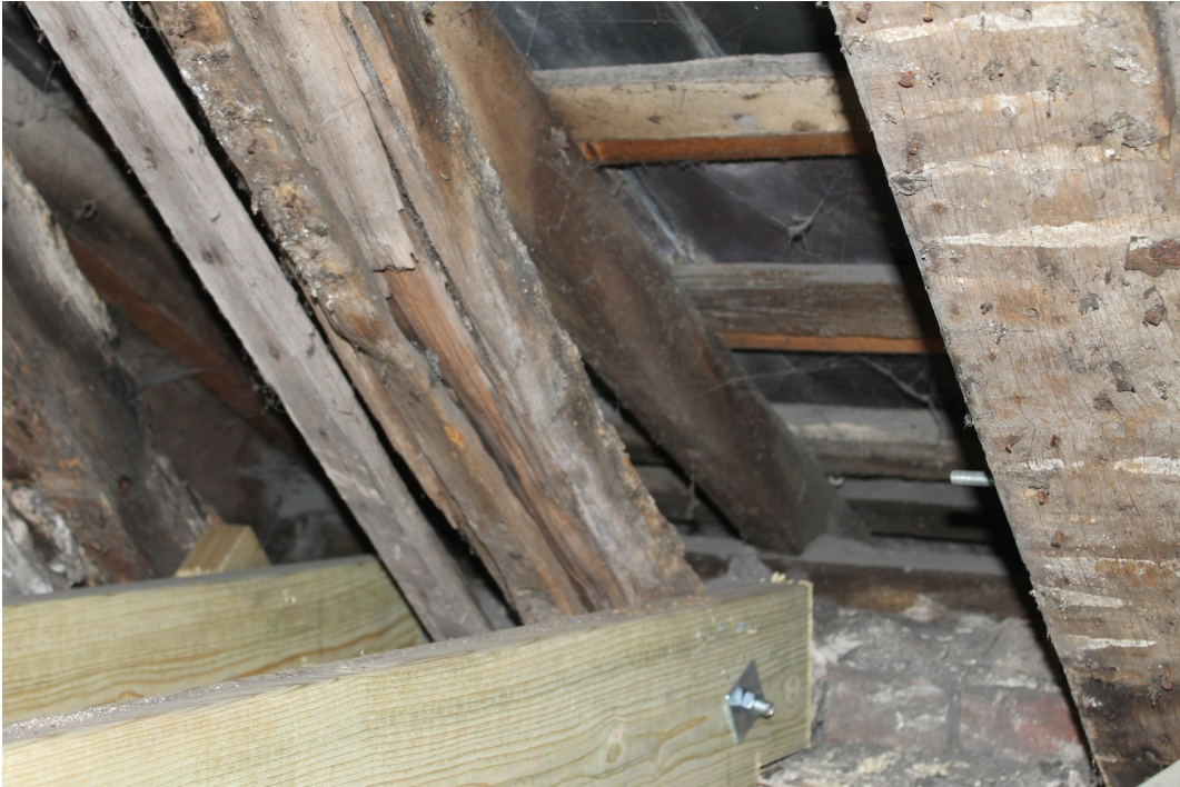
Photograph 15 Sprockets at the feet of the street side rafters, allowing the roof to flare out over the brick facing – note the slate roof covering above the battens – view north-east
