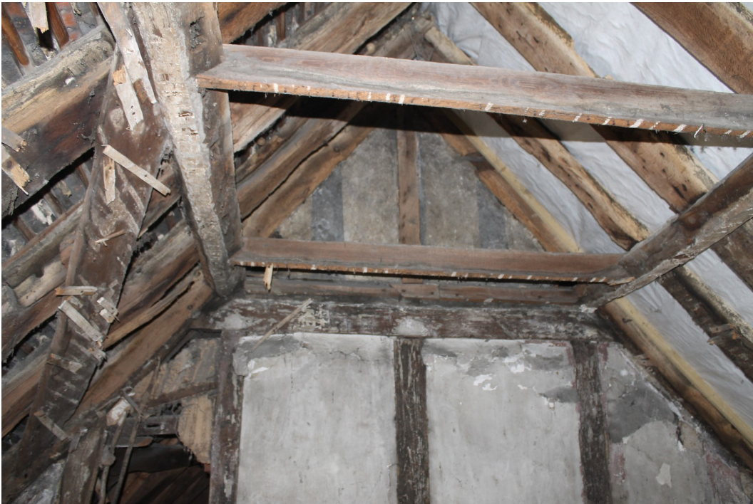
Photograph 9 Interior of the roof space looking towards the central cross frame with the original wattle and daub infill panels. The wind brace can be seen on the left, below the street side purlin which displays toolmarks on its underside and empty mortises, indicating it is a re-used timber – view south
