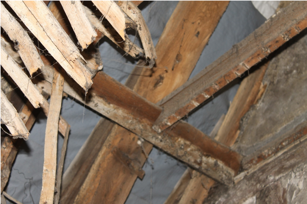
Photograph 8 Machine-cut collar with birdsmouth scarf joint to the purlin, to which the earlier lath and horsehair plaster ceiling was nailed – view south-east
