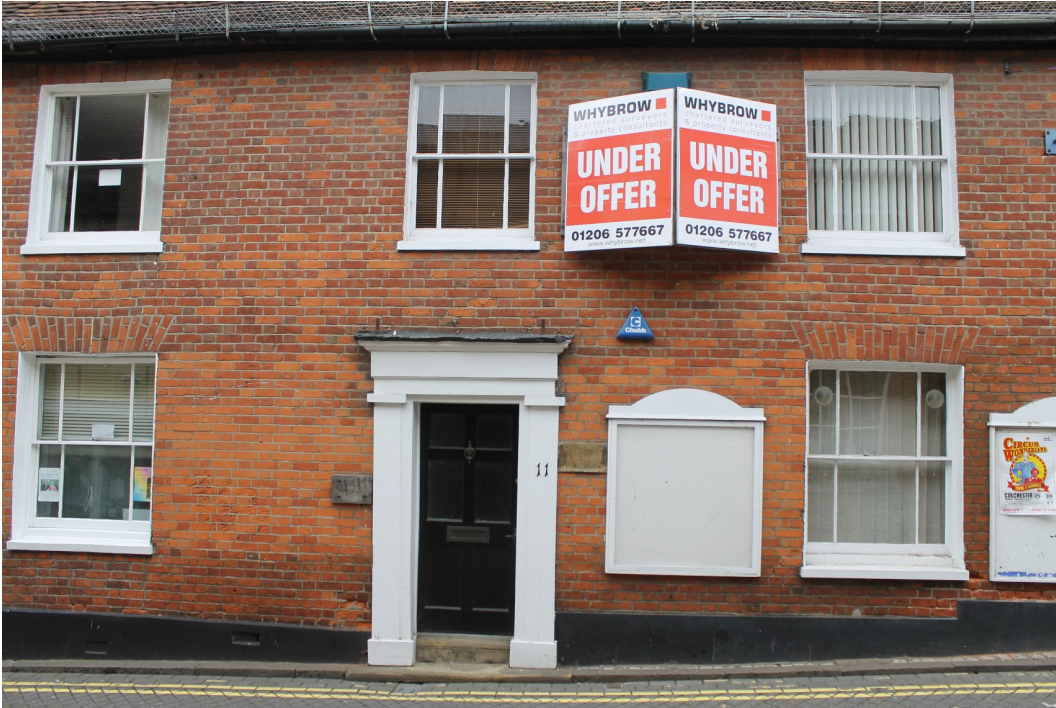
Photograph 1 Street frontage of No. 11 showing the symmetry of the probable 19th-century brick facing – view west
