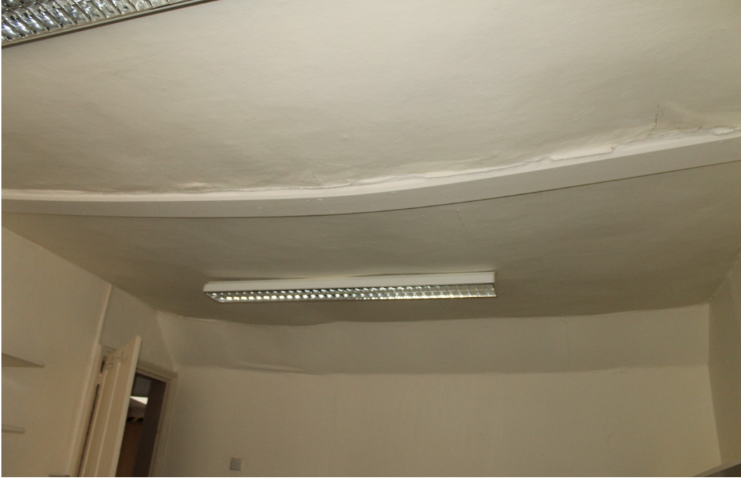
Photograph 4 Sagging ceiling, with bowed bridging beam in first floor room – view west
