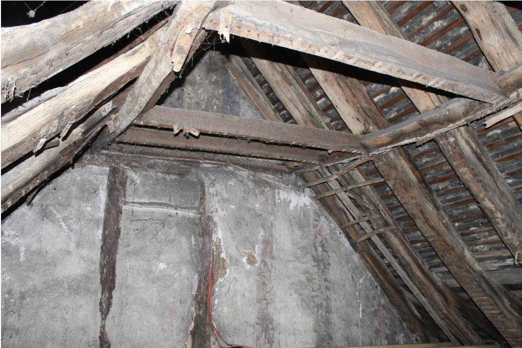
Photograph 10 Interior of the roof space looking towards the gable frame with the original wattle and daub infill panels – view north
