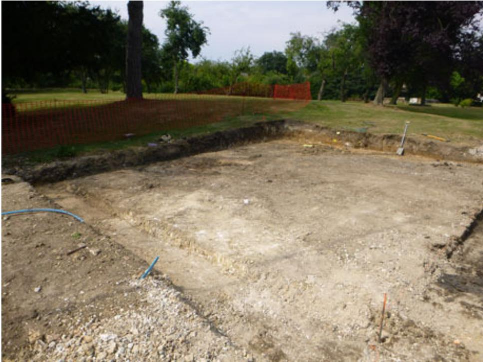
**Photograph 1** Ground reduction within footprint of new pool building, looking NW
