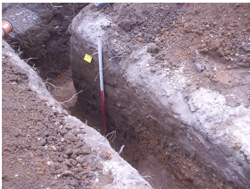
Photo 2 Pit F1 excavated within the footings of the excavation
