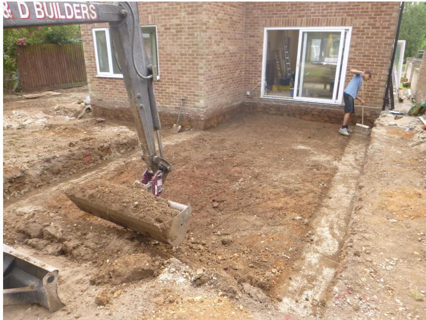
Photo 1 Shot of southern part of the site during excavation
