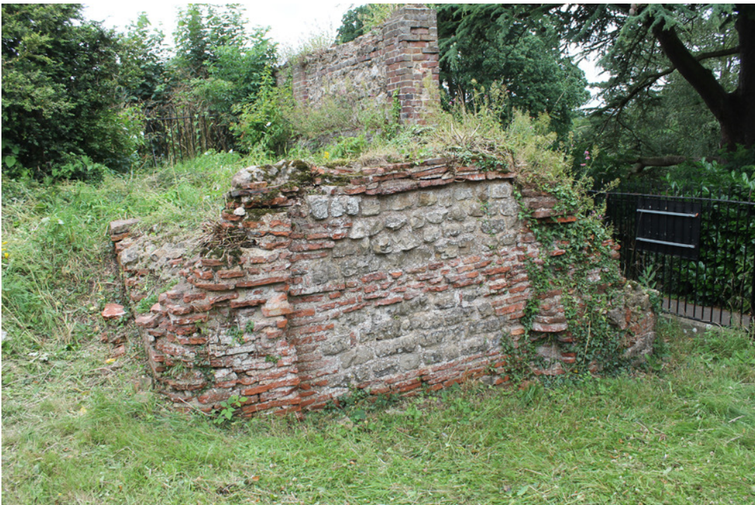
Photograph 8 Western pier of Duncan's Gate Photograph taken facing north-west.
