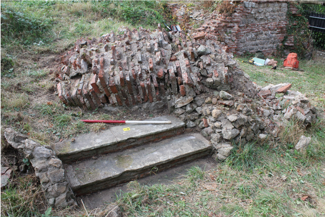
Photograph 15 Collapsed masonry, showing tile courses repaired with modern concrete. Also visible is the modern steps added to the collapse in the early 20th-century. Photograph taken facing north-west.
