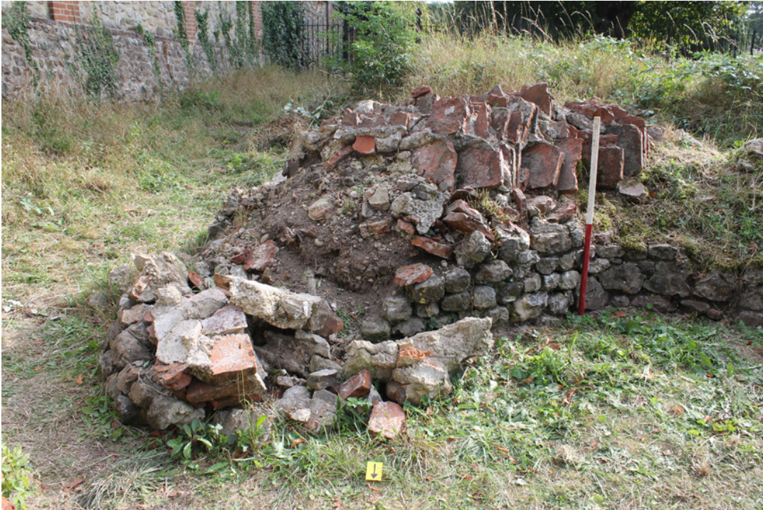
Photograph 17 Recent collapse to east of masonry. Lime mortar exposed behind concrete render and retaining wall. Photograph taken facing south.
