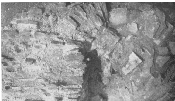
Photograph 2 Detailed photo of window arch visible in collapsed masonry (reproduced from Roman Colchester, 1958, plate IVb).
