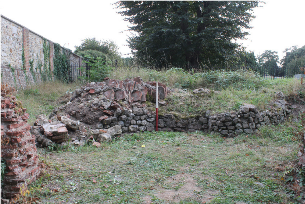
Photograph 13 Collapsed masonry after the removal of overgrowth. Photograph taken facing south.
