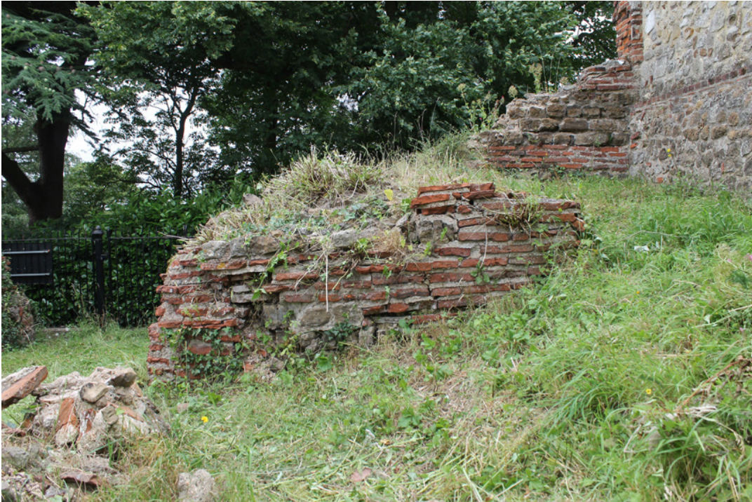
Photograph 11 Southern face of eastern pier. Visible is the decayed concrete used to consolidate the wall in the 1920s. Photograph taken facing north.
