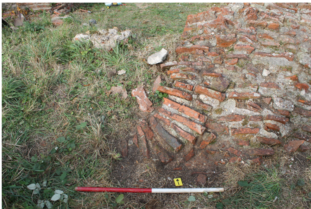
Photograph 19 Arch of window in collapsed masonry. Photograph taken facing north.
