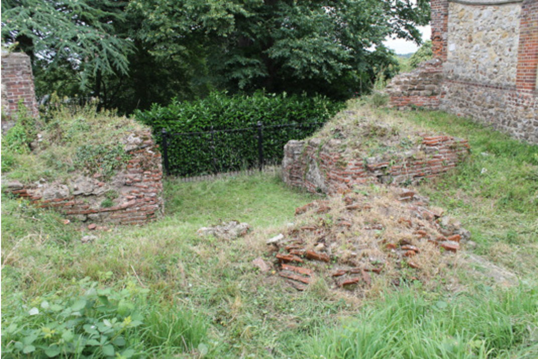
Photograph 7 General shot of Duncan's Gate. Collapsed masonry visible in foreground. Photograph taken facing north-east.
