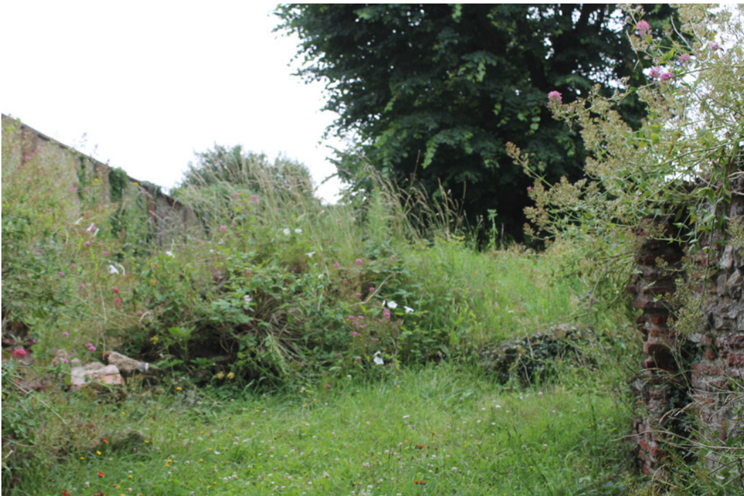
Photograph 12 Collapsed masonry prior to the removal of overgrowth. Photograph taken facing south.
