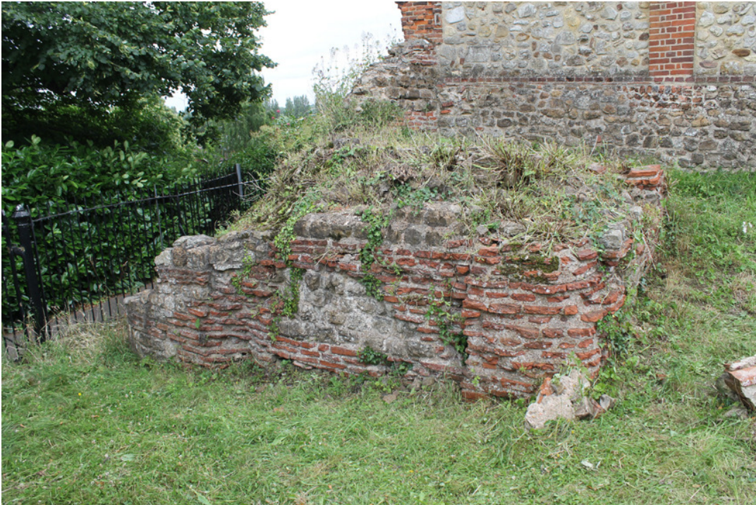
Photograph 9 Eastern pier of Duncan's Gate. Photograph taken facing north-east.
