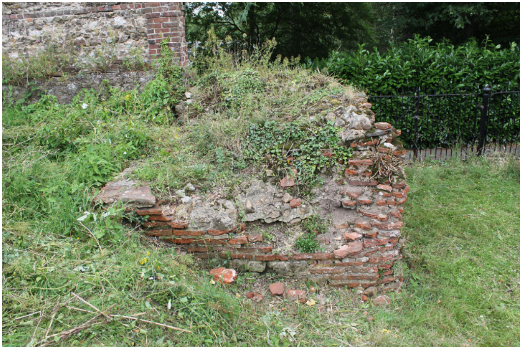
Photograph 10 Southern face of western pier. Visible is the decayed concrete used to consolidate the wall in the 1920s. Photograph taken facing north.
