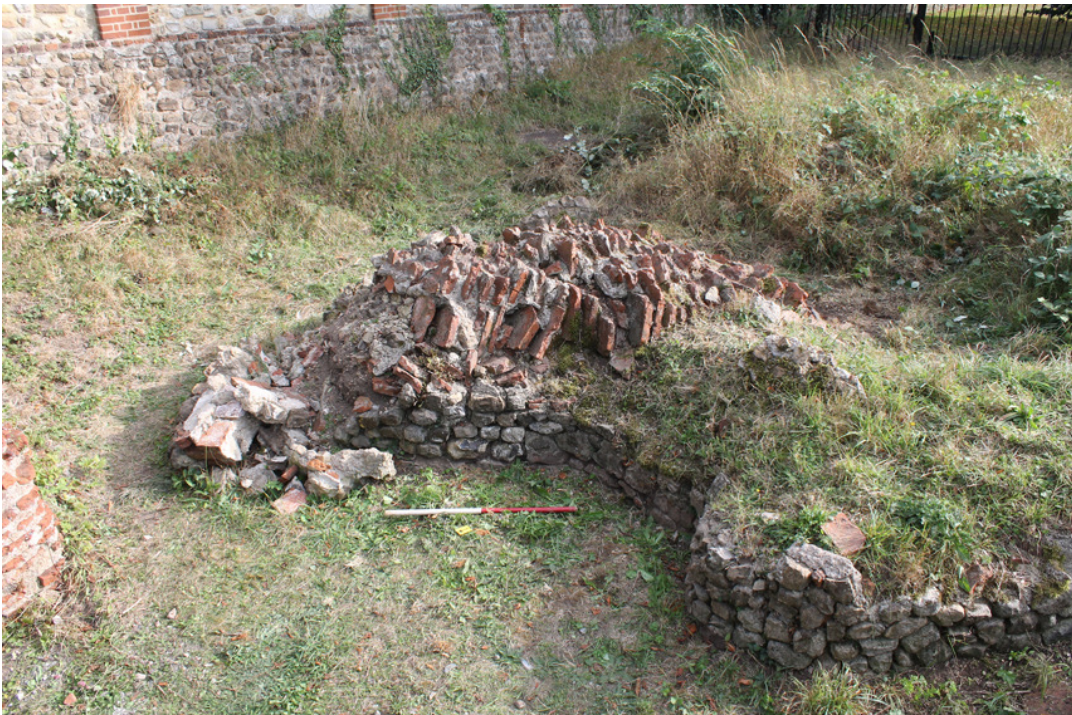
Photograph 14 Collapsed masonry after the removal of overgrowth. Photograph taken facing south-east.
