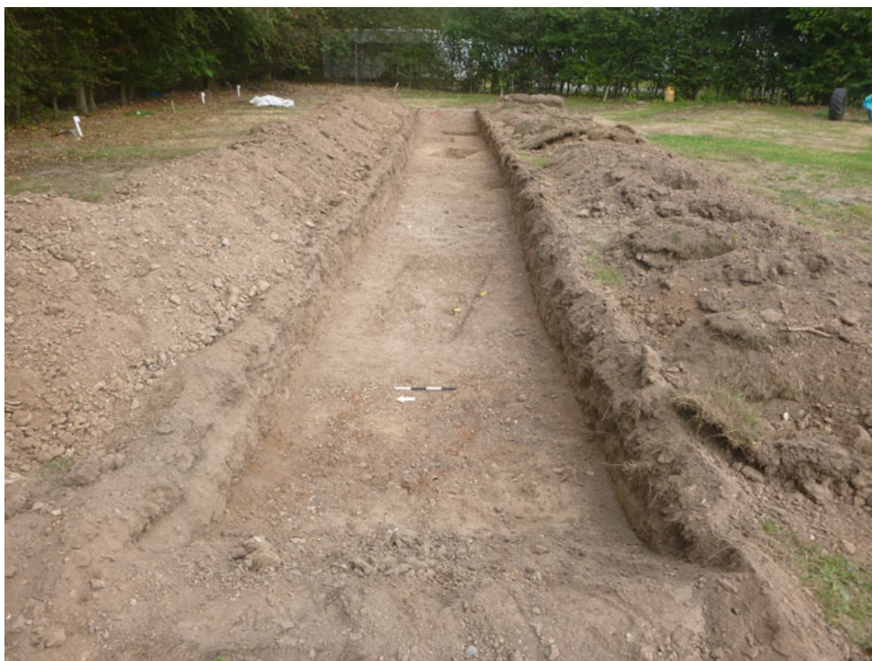
Photograph 1 T2, looking E
