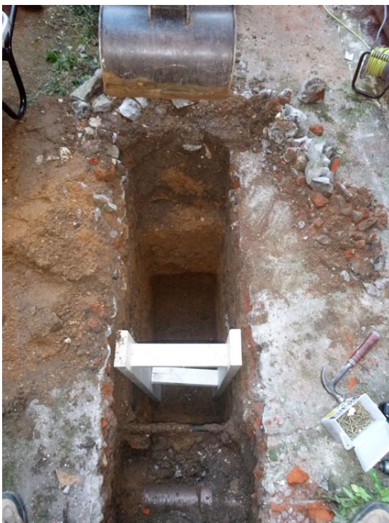
Photograph 2 Foundation trench, looking NE
