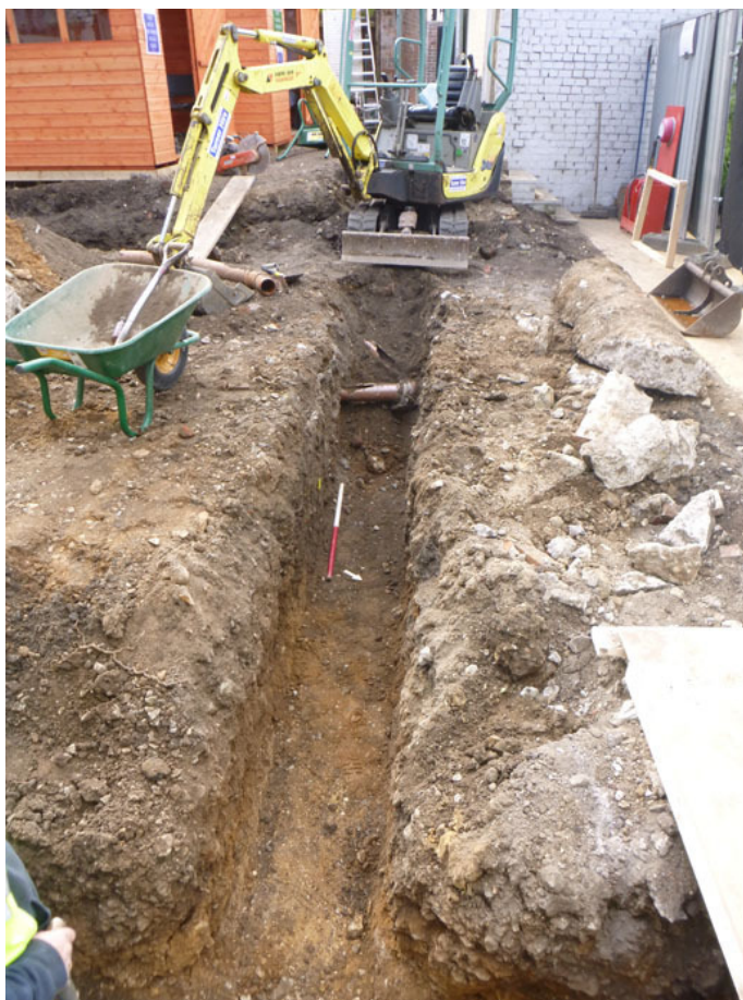
Photograph 2 F2 and foundation trench, looking SW
