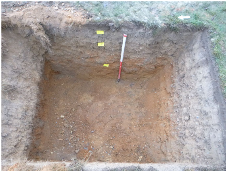
Photograph 2 Soakaway, looking E
