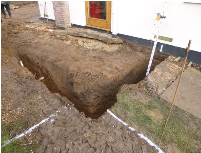
Photograph 1 Groundworks for the side extension, looking NE
