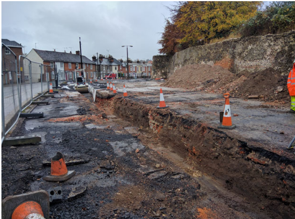
Photograph 2 Groundworks for the French drain, looking SW
