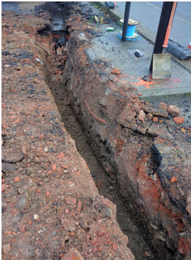
Photograph 3 Groundworks for the street light cabling, looking NE
