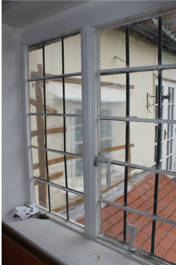
Photograph 29 16th-century casement window in south-east wall of FF5 – view east.
