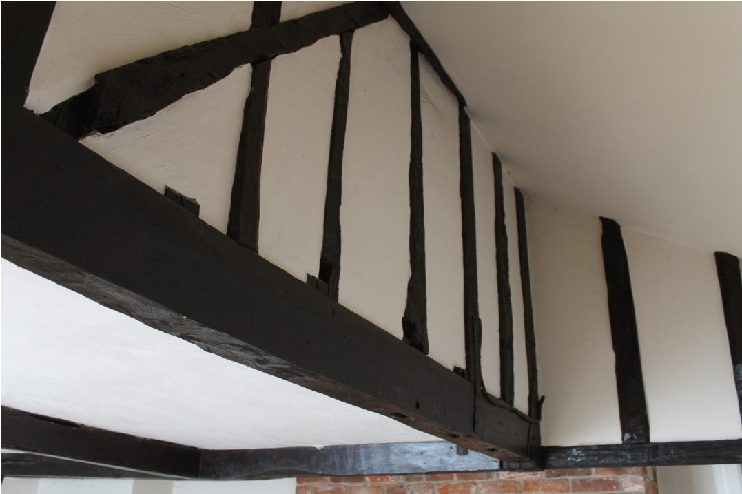
Photograph 17 External studwork of the first floor to the 18th-century extension to the 16th-century cross-wing concealed by the 19th-century single-storey extension on the north-west elevation (GF2) – view north.
