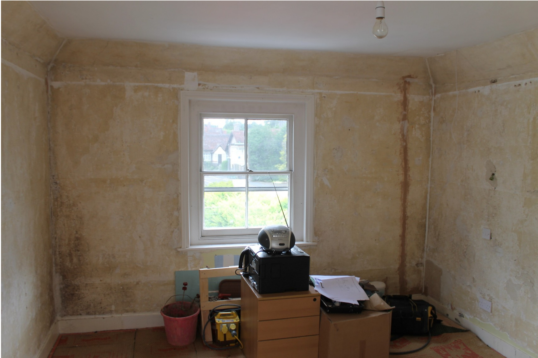
Photograph 31 Interior of FF8 with inserted 19th-century sash window – view south-west.
