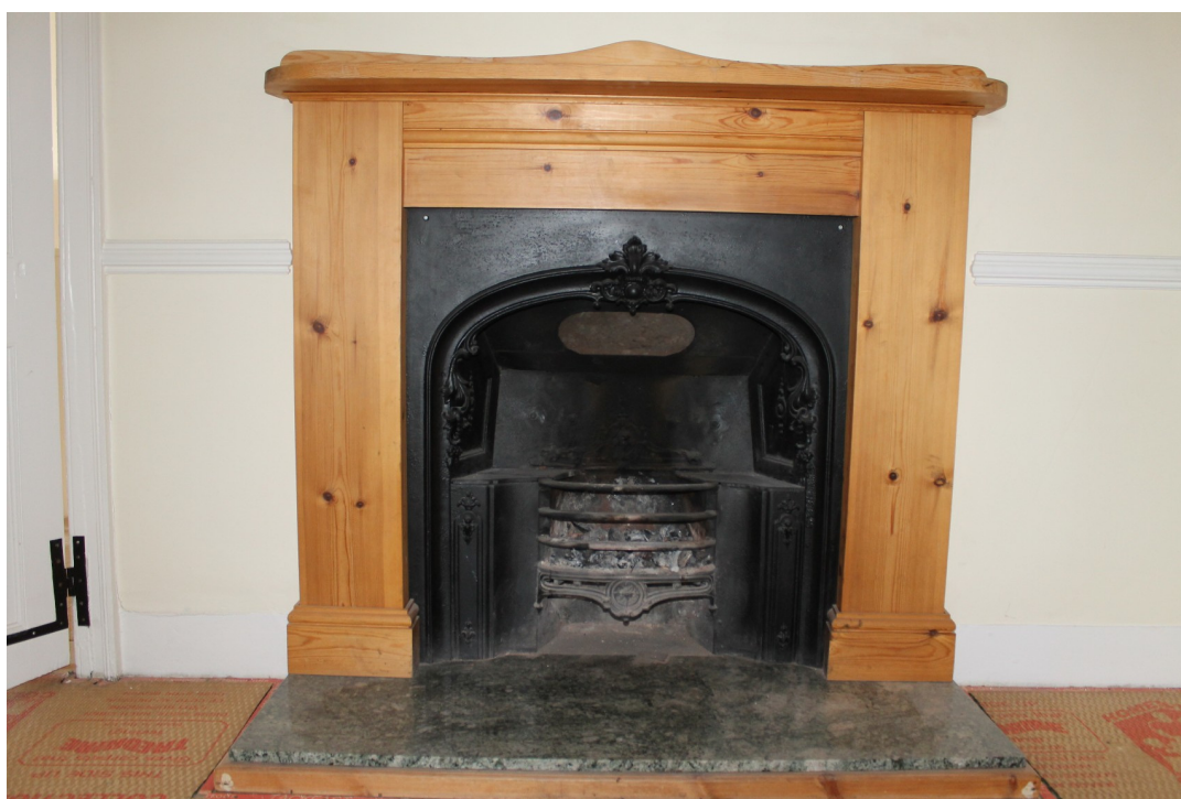
Photograph 22 FF1, 18th-century cast-iron register grate with modern fire surround – view south-west.
