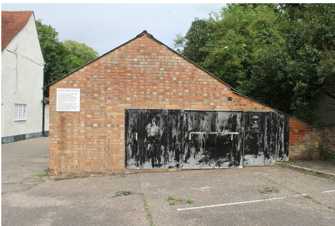
Photograph 36 South-west elevation of outbuilding – view north-east.
