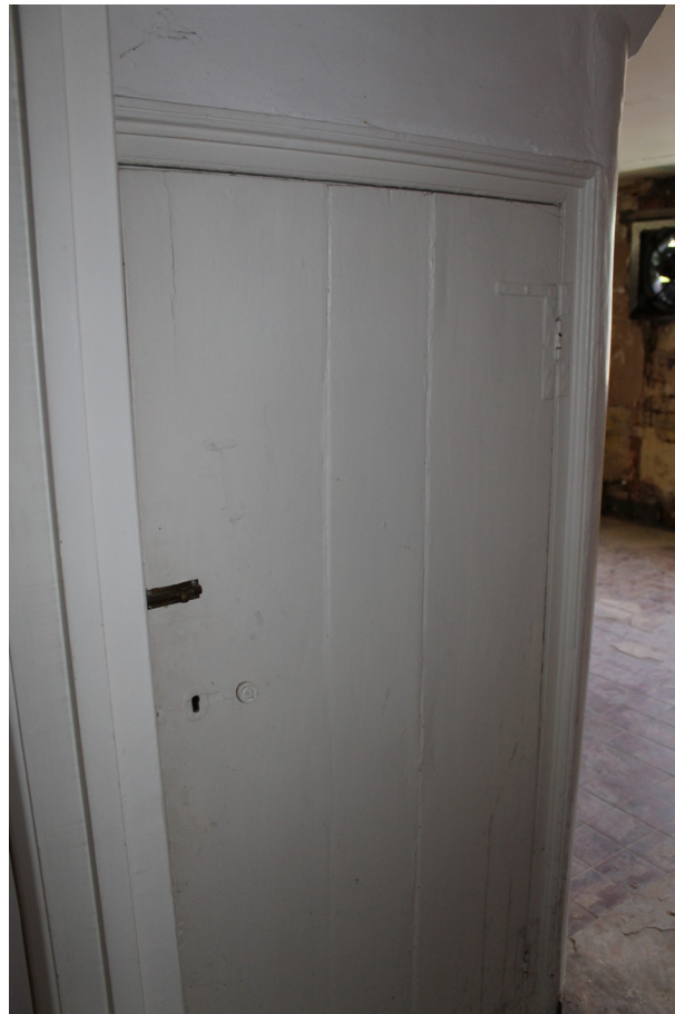
Photograph 20 18th-century under stairs cupboard between GF1 and GF3 – view south-west.
