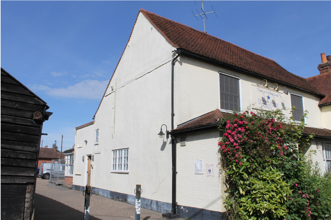
Photograph 5 South-east elevation - view west.
