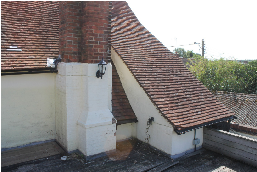
Photograph 4 South-west elevation of the 15th-century main range with the 18th-century chimney stack and the flared roof covering the probable 18th-century external staircase - view east.
