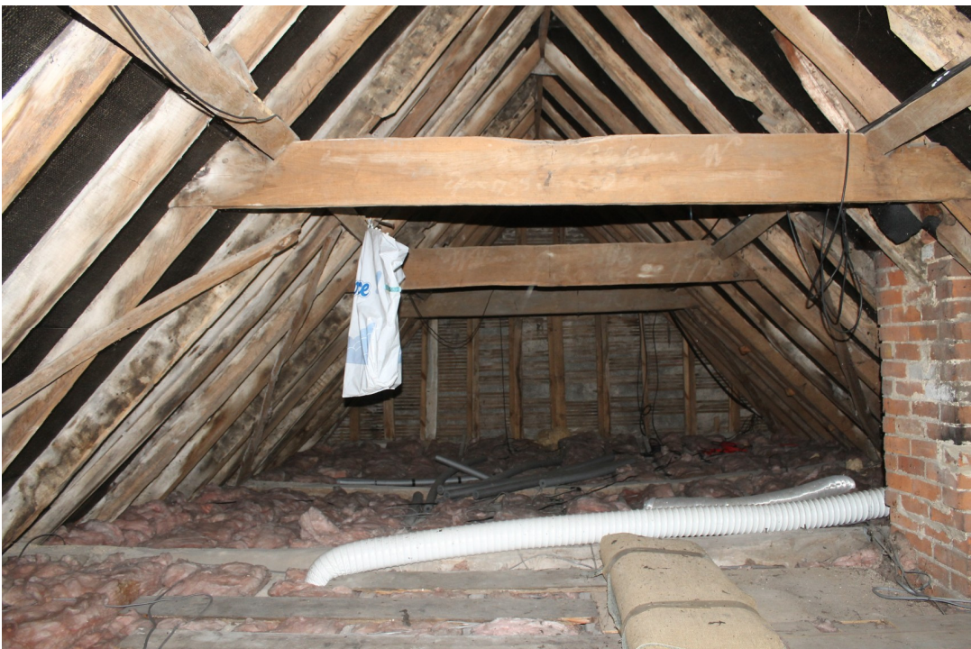
Photograph 32 Roof timbers above 15th-century main range (FF1-3) – view south-east.
