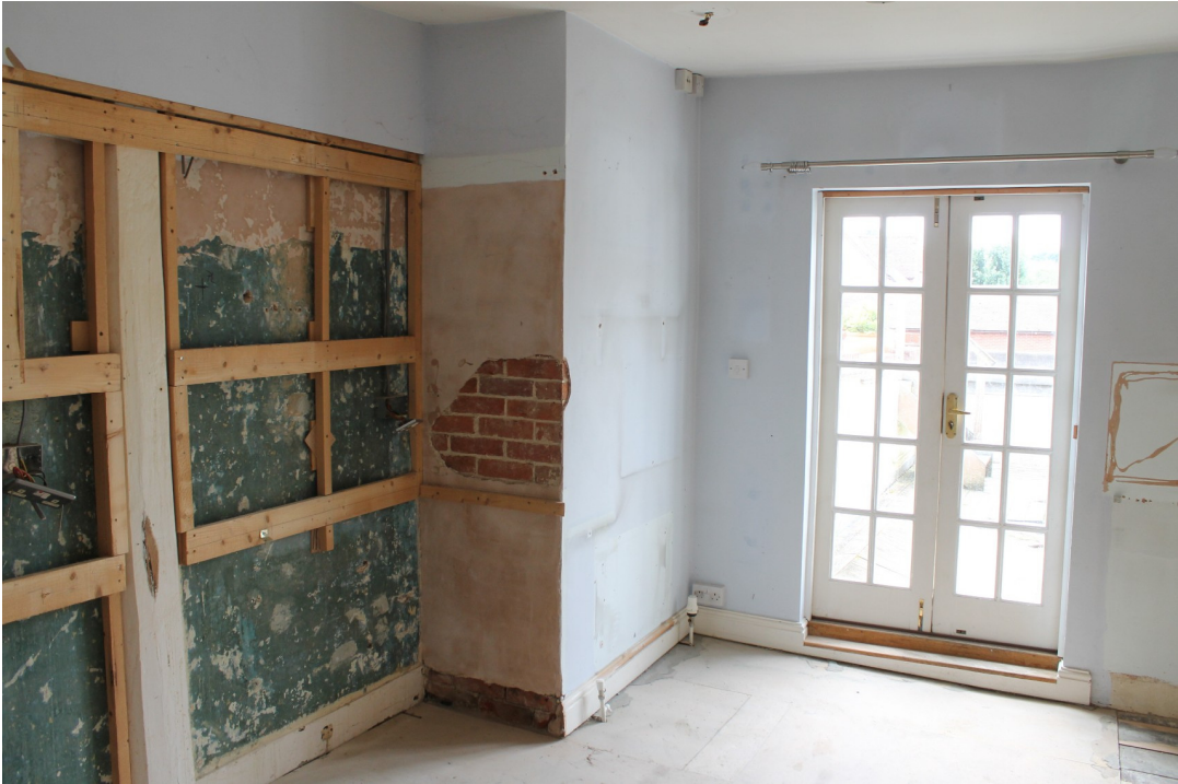
Photograph 25 18th-century dividing wall between FF1 and FF2, built around 15th-century storey post and with 20th-century chimney stack and French doors to roof – view south-east.
