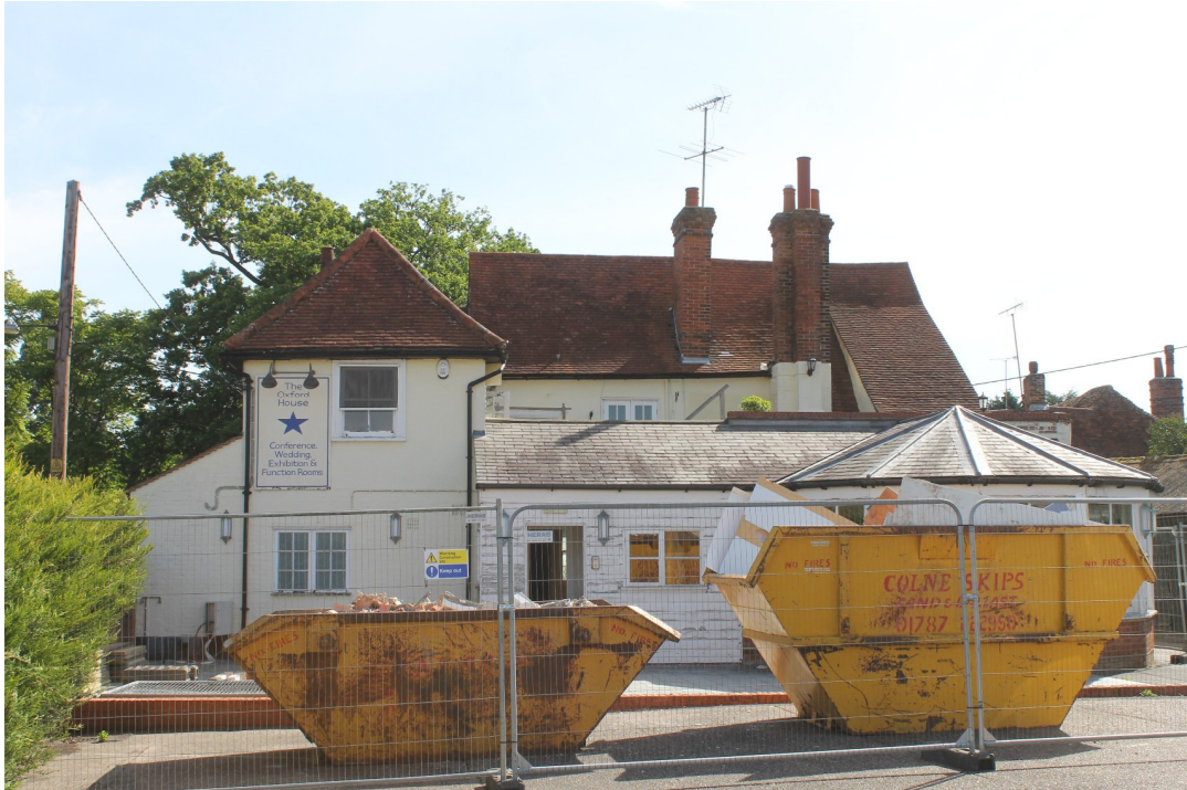
Photograph 3 South-west elevation - view north-east.
