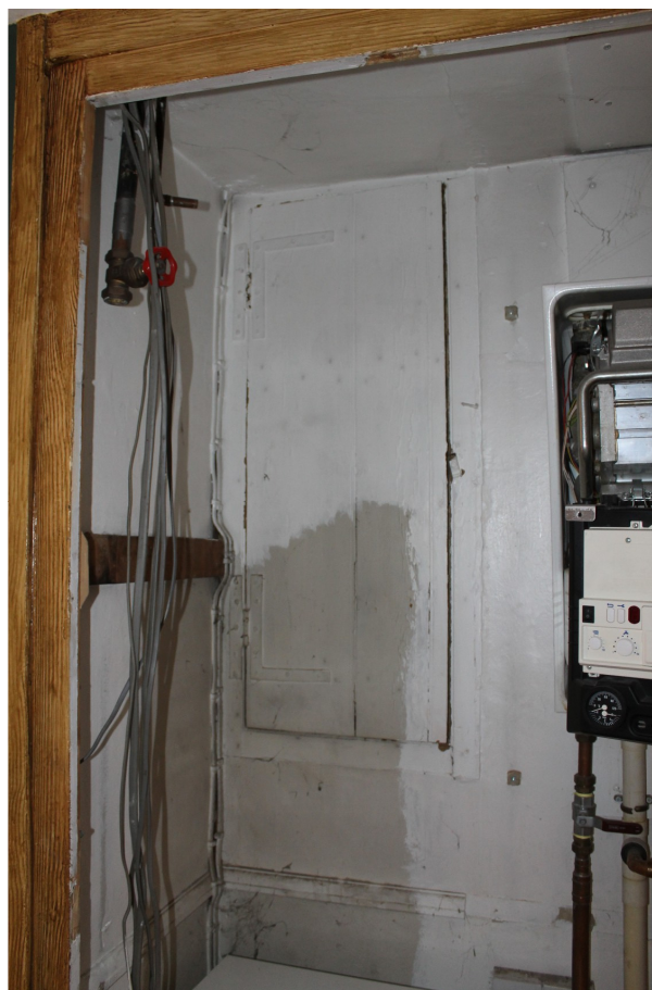
Photograph 28 Cupboard built against chimney stack off FF5 – view north-west.
