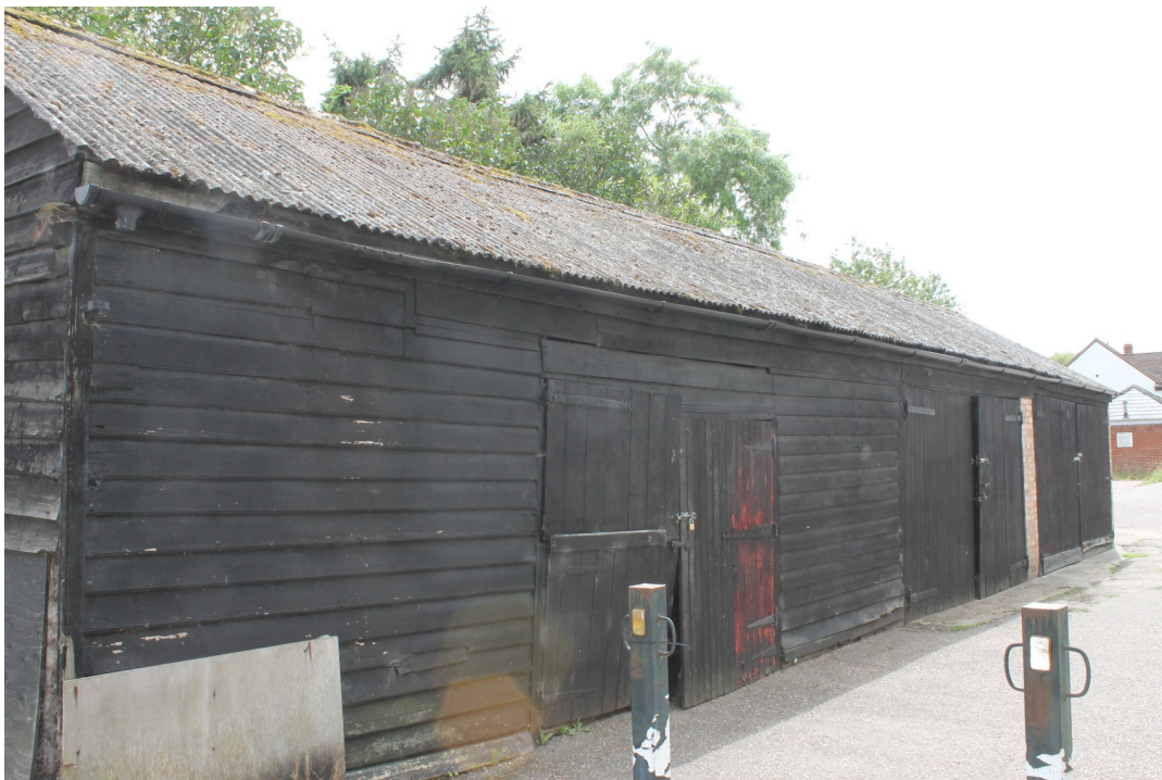
Photograph 35 North-west elevation of outbuilding – view south.
