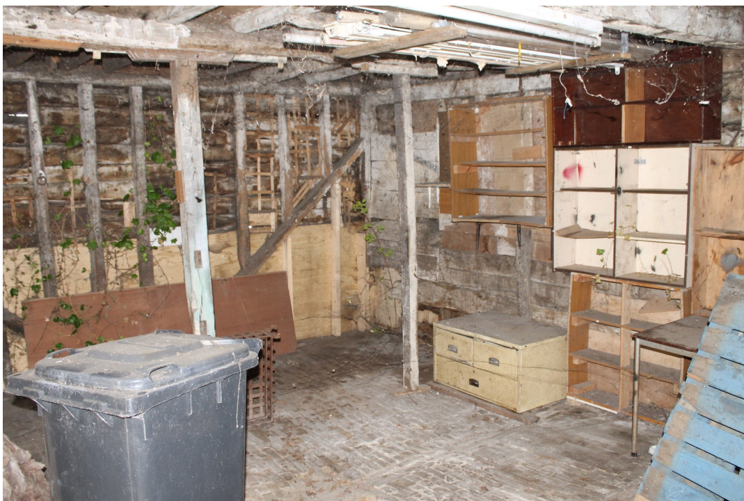
Photograph 37 Interior of OB1 – view east.
