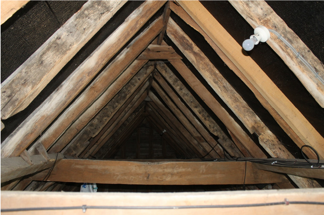
Photograph 33 Intermediate high collars and ridge board above 15th-century main range (FF1-3) – view south-east.
