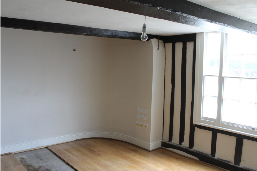
Photograph 15 Interior of GF2 showing the curved brickwork of the 19th-century single-storey extension on the north-west elevation – view north.
