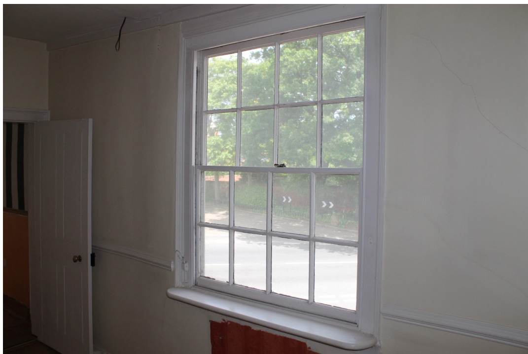
Photograph 23 18th-century sash window in north-east wall of FF1 – view north.
