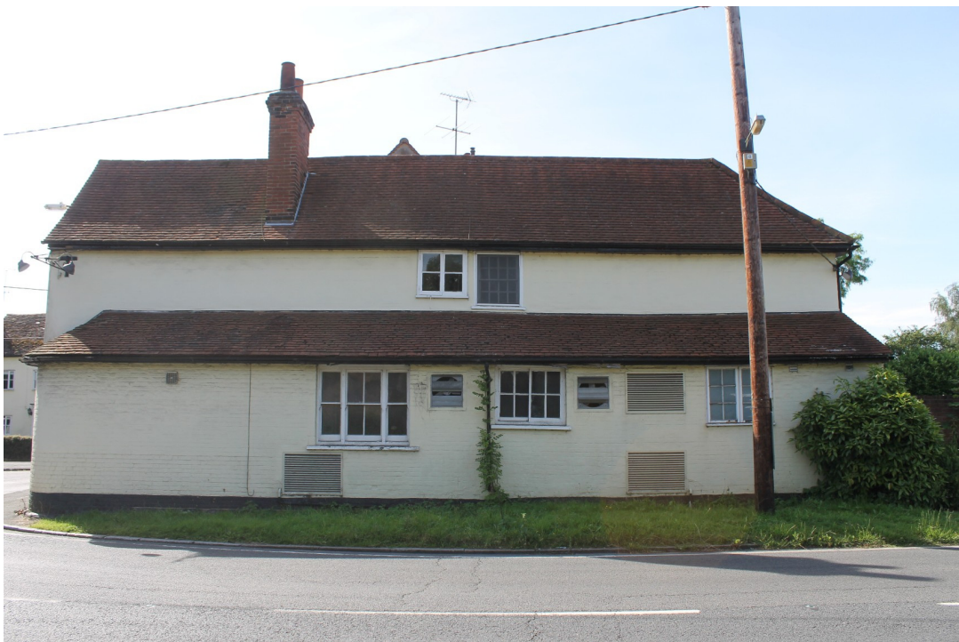
Photograph 2 North-west elevation - view south-east.
