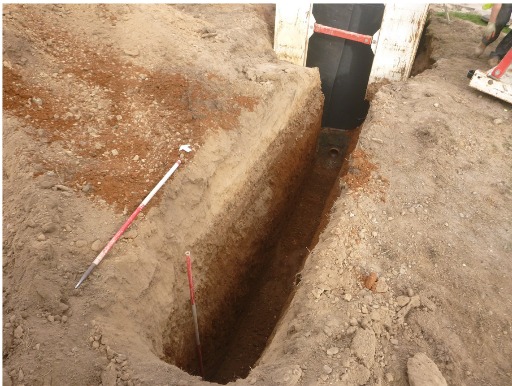
Photograph 1 Drainage trench, looking NNE
