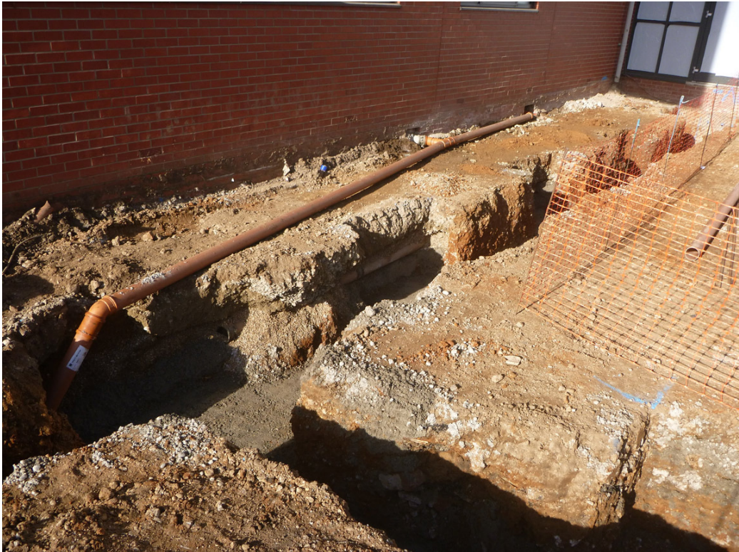
Photograph 3 Foundation trenches, looking NNW
