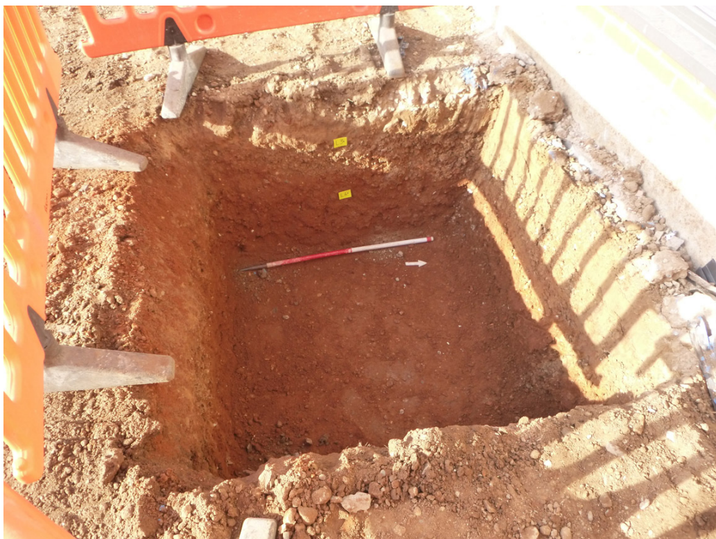
Photograph 2 Foundation pad, looking W
