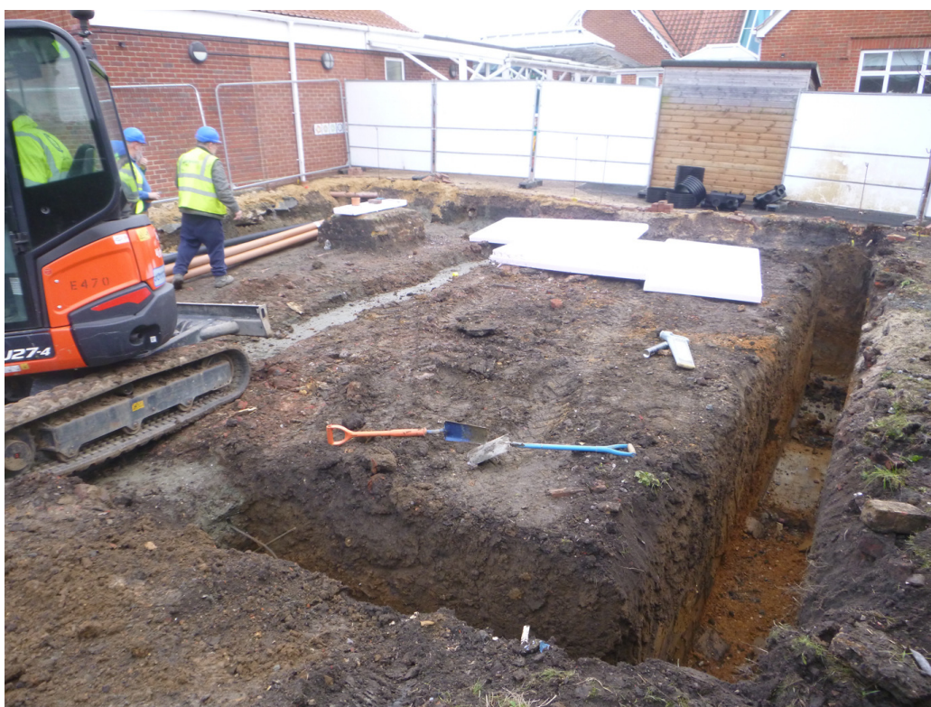
Photograph 2 Excavation of footings, looking NE
