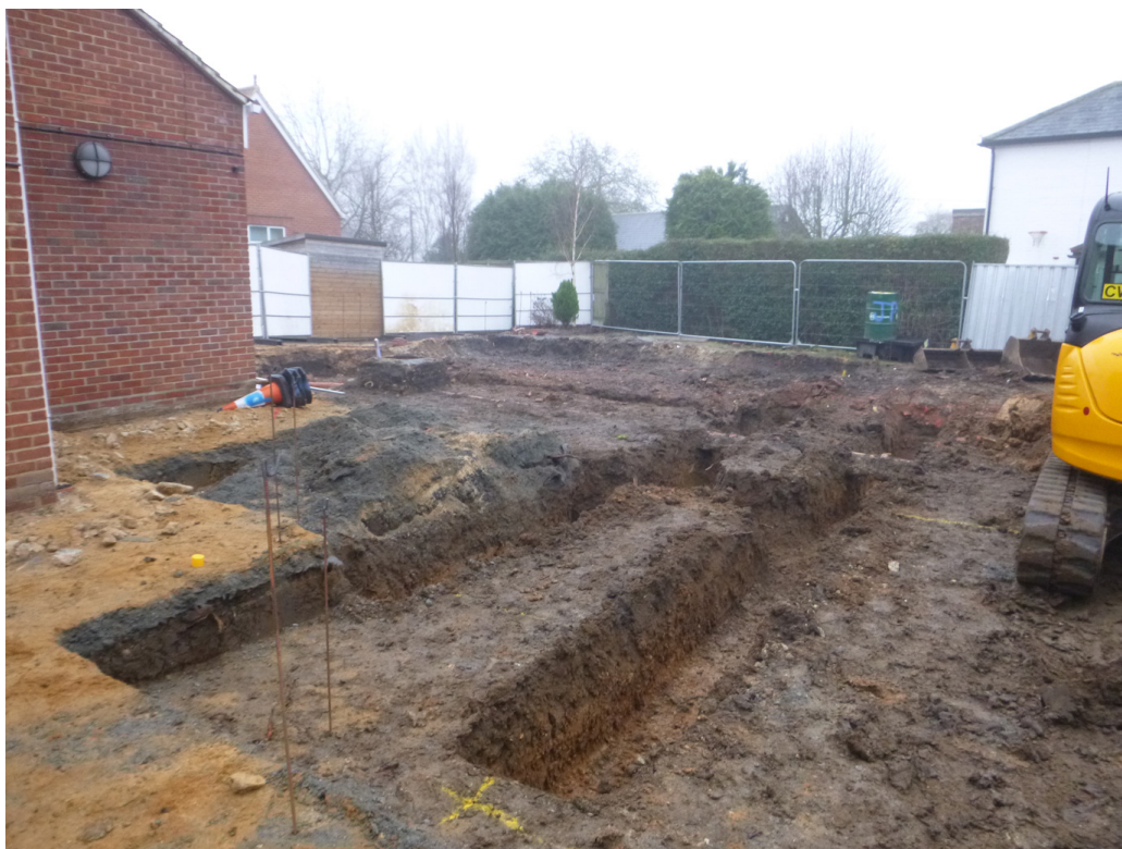
Photograph 1 Excavation of footings, looking SE
