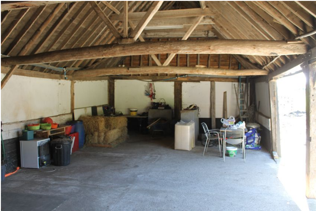
Photograph 18 Interior of extension of Building B. Photograph taken facing south.
