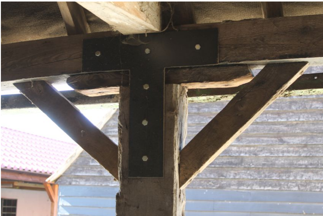
Photograph 19 Steel bracing supporting primary-post in entrance to Building B extension. Photograph taken facing west.
