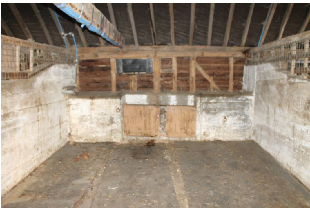
Photograph 6 Central stall in Building A, with concrete feeding troughs and hay racks. Photograph taken facing south.
