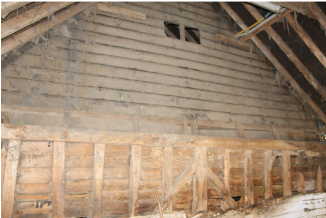
Photograph 4 Original eastern gable end of Building A, showing missing gable and beginning of extension (A2). Photograph taken facing south-east.
