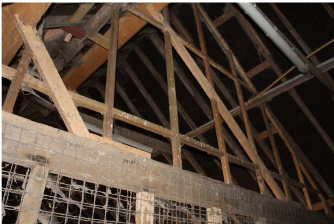
Photograph 5 Building A, showing modern timbers used to support the roof in the absence of a tie-beam. Photograph taken facing south-east.
