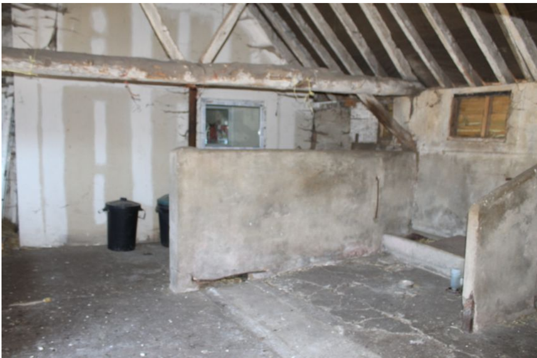
Photograph 13 Building B interior. Photograph taken facing north.
