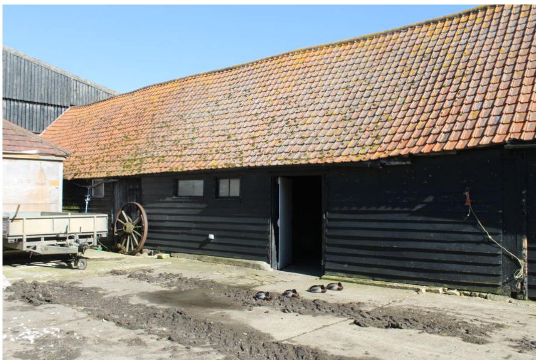
Photograph 10 Western elevation of Building B. Photograph taken facing north-east.
