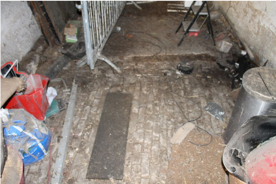
Photograph 3 Building A westernmost stall, showing pavior brick flooring. Photograph taken facing south.
