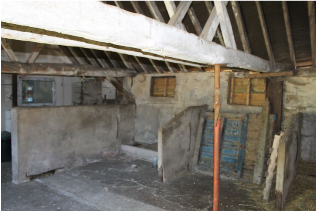
Photograph 14 Building B interior. Photograph taken facing north-east.
