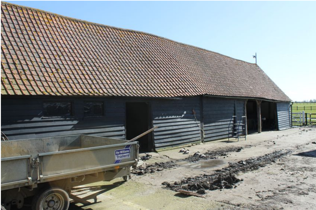
Photograph 17 Western elevation of Building B and its extension. Photograph taken facing south-east.
