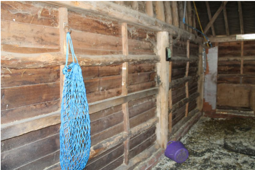
Photograph 7 Detail of wall construction in the extension to Building A, showing rails and separate studs jointed between them. Photograph taken facing south-west.
