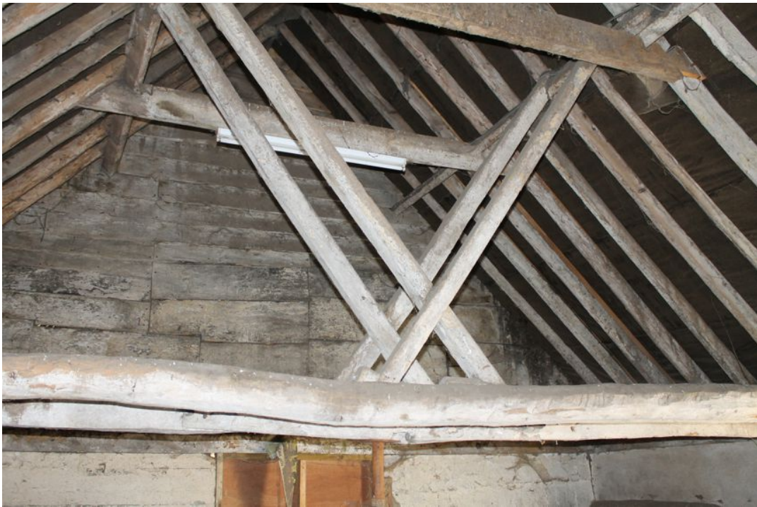
Photograph 15 Replacement scissor brace trusses in Building B. Photograph taken facing south.
