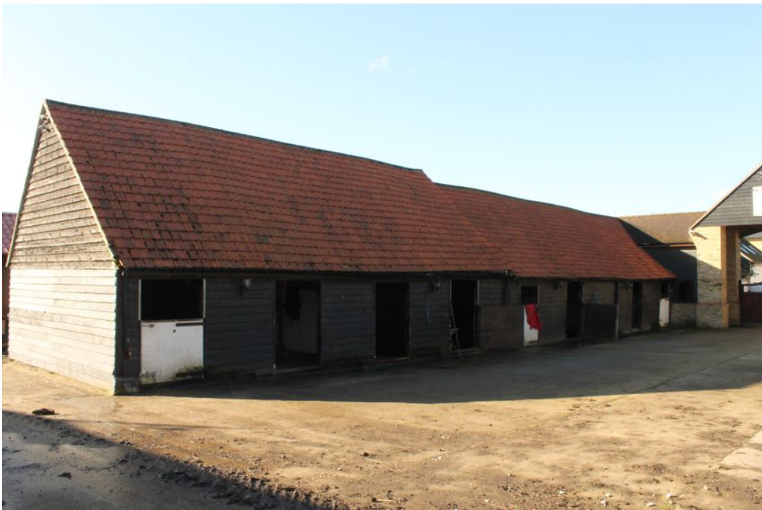
Photograph 1 Building A northern elevation. Photograph taken facing south-west.
