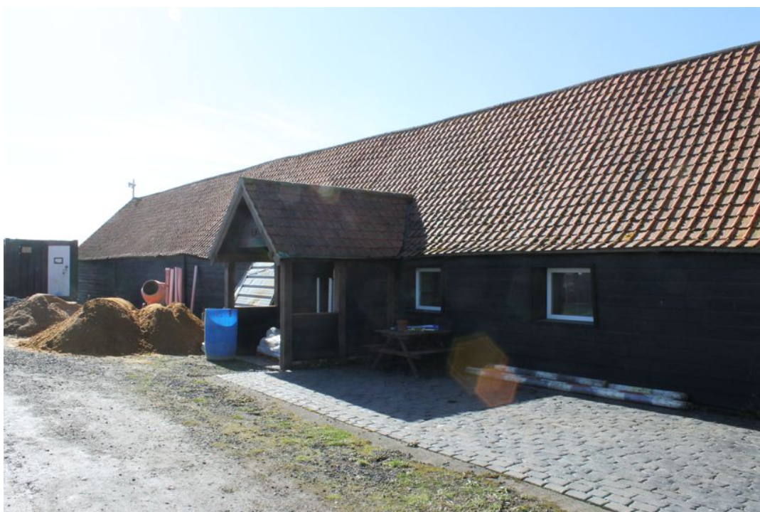
Photograph 11 Eastern elevation of Building B. Photograph taken facing south-west.
