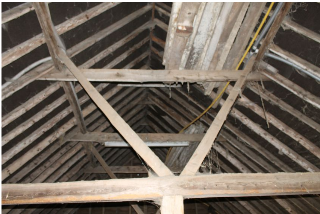
Photograph 9 Truss in extension to Building A. Photograph taken facing east.
