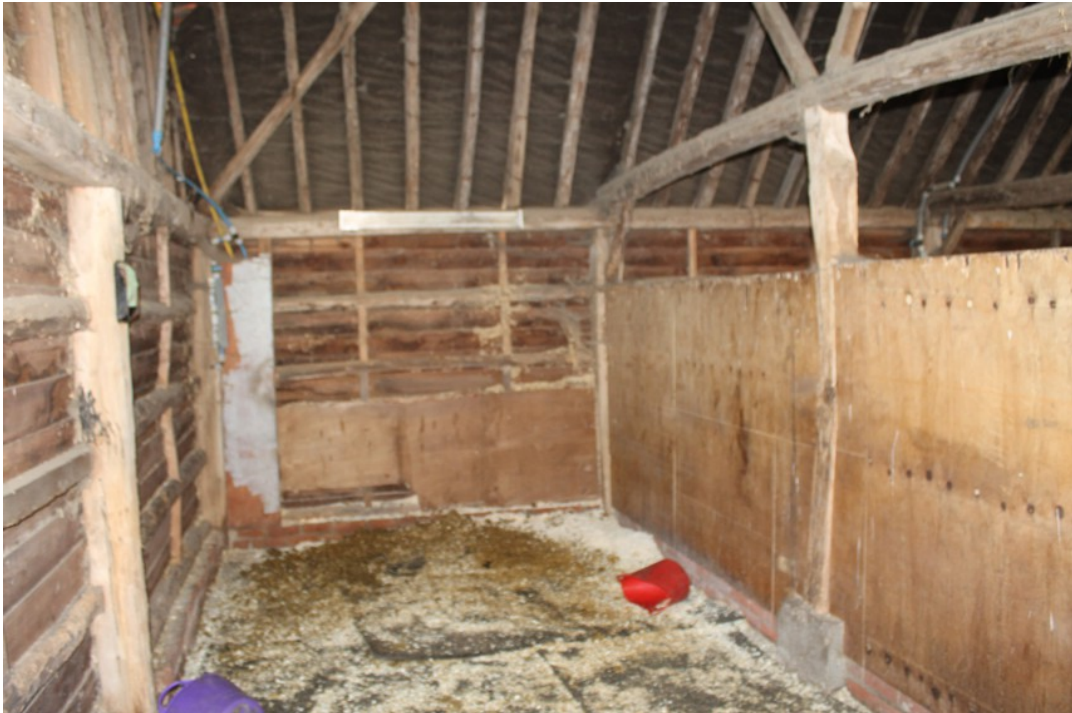
Photograph 8 Westernmost stall in the extension to Building A. Photograph taken facing south.
