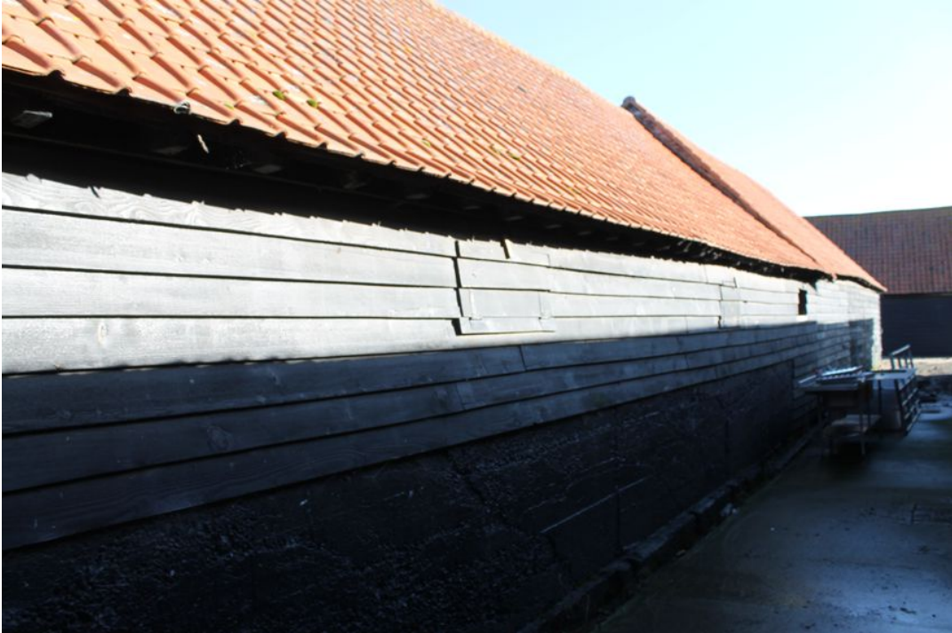
Photograph 2 Building A southern elevation, showing wooden awning shutters. Photograph taken facing north-east.
