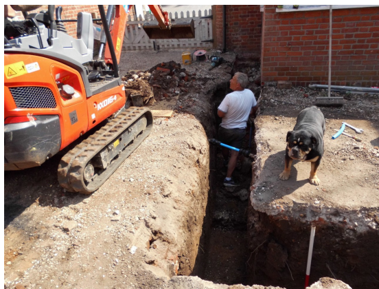
Photograph 2 N-S foundation - looking south
