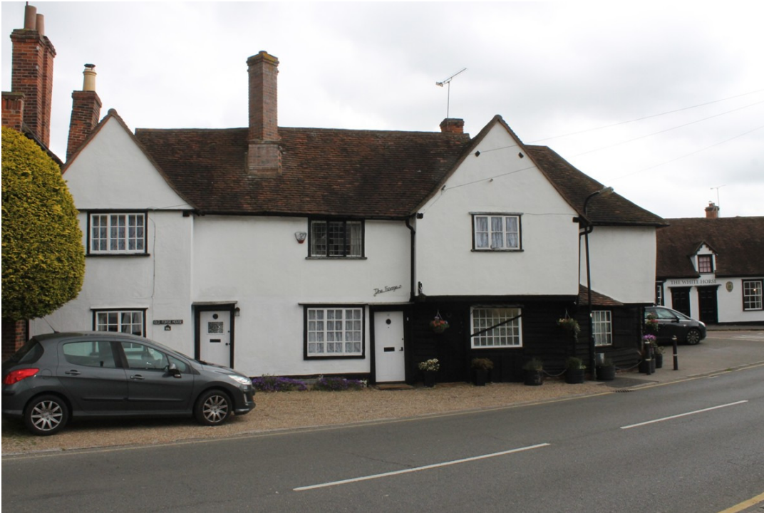
Photograph 1 South-west elevation of the medieval building with the 1425 cross-wing to the left (18a Chipping Hill), the 1375 hall house in the centre (mainly 18 Chipping Hill) and the 1500 cross-wing to the right (18 Chipping Hill to the upper floor, The Forge to the ground floor). The 17th-century extensions are to the right of the 1500 cross-wing - view north-east.
