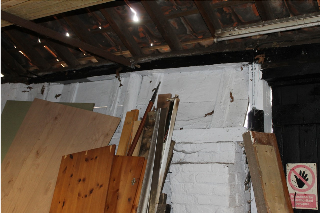
Photograph 30 Original top-hung shutters in the south-east wall of the farrier's shop - view south-east.
