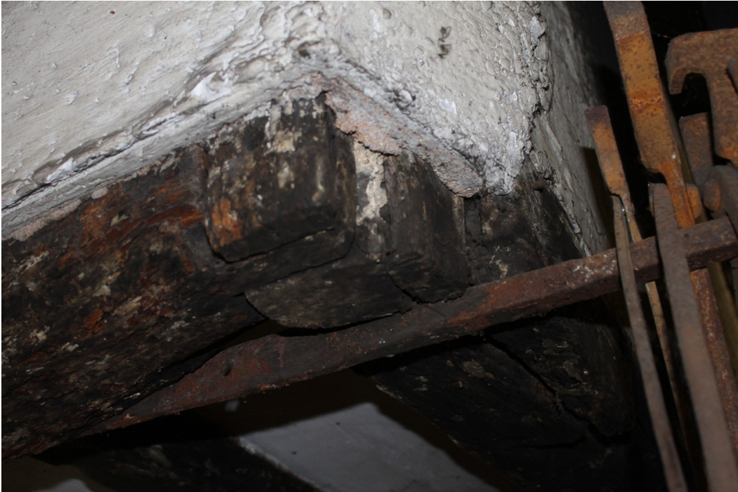
Photograph 21 The north-east corner of extension A viewed from extension B where the corner post of the timber frame has been sawn off, exposing the joints with the adjoining wall plates.
