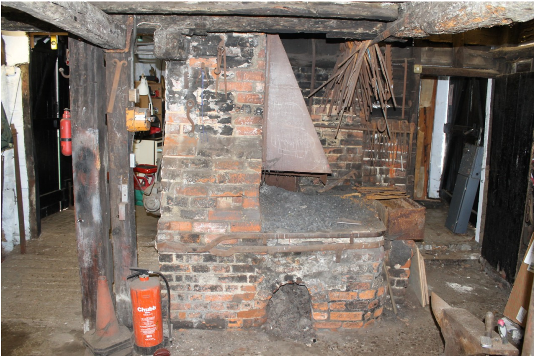
Photograph 24 Extension B behind extension A, housing the second forge with a doorway to the right originally providing access to the yard but now to the farrier's shop. The brickwork behind the forge appears to be a remnant of a yard wall - view north-east.
