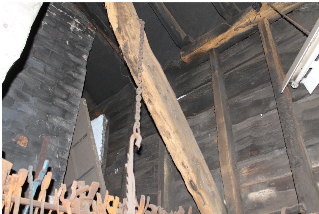
Photograph 25 Extension B behind the second forge with the wide-section weatherboard on top of the earlier yard wall and the straight brace rising to the corner of extension A - view north.
