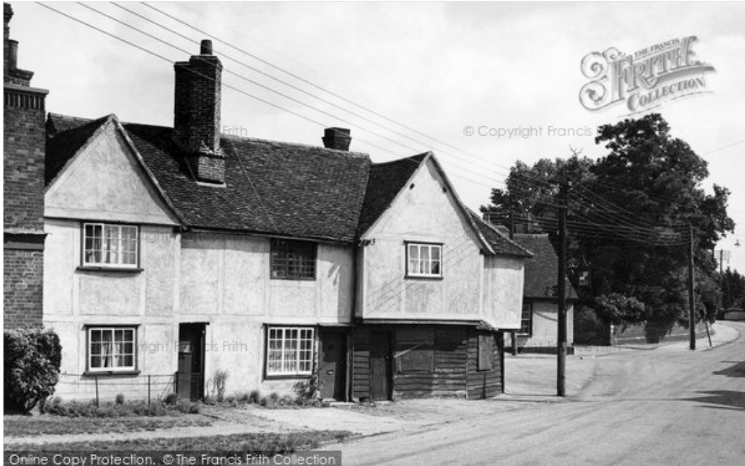
Historic Photograph 5 The Forge, Chipping Hill 1950
