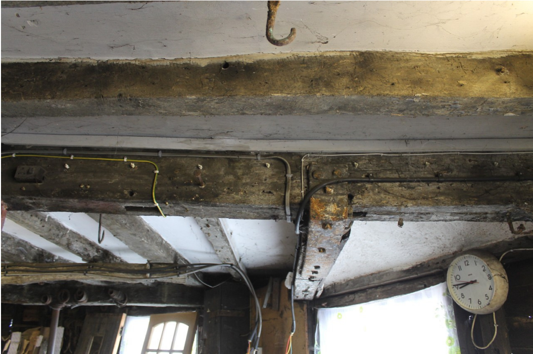
Photograph 15 South-east wall plate to the front bay of the cross-wing with two widely-spaced mortices, perhaps indicating windows were once located here. The 17th-century extensions are behind the wall plate, with extension A's wall plate tied into the wall plate of the cross-wing - view south-east.
