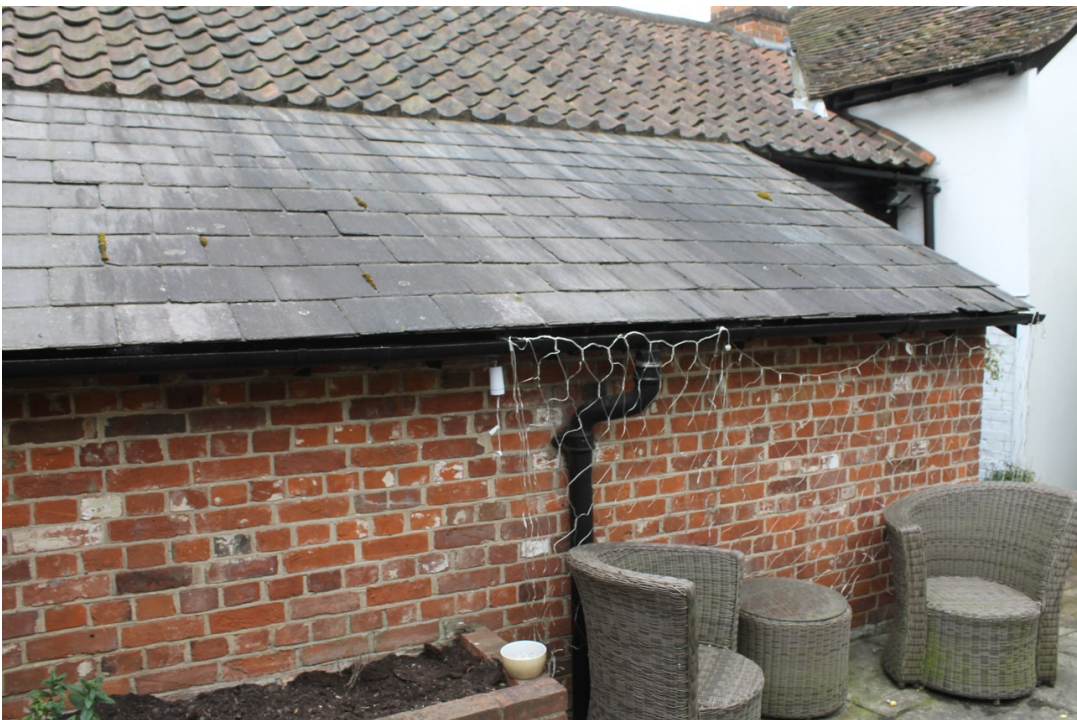
Photograph 32 Slate-roofed lean-to on the north-west side of the farrier's shop - view south-west.
