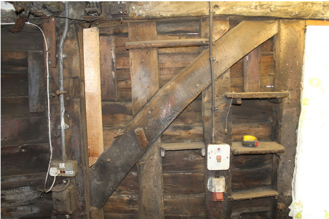
Photograph 14 Internal brace and studs to the front frame of the cross-wing - view south-west.
