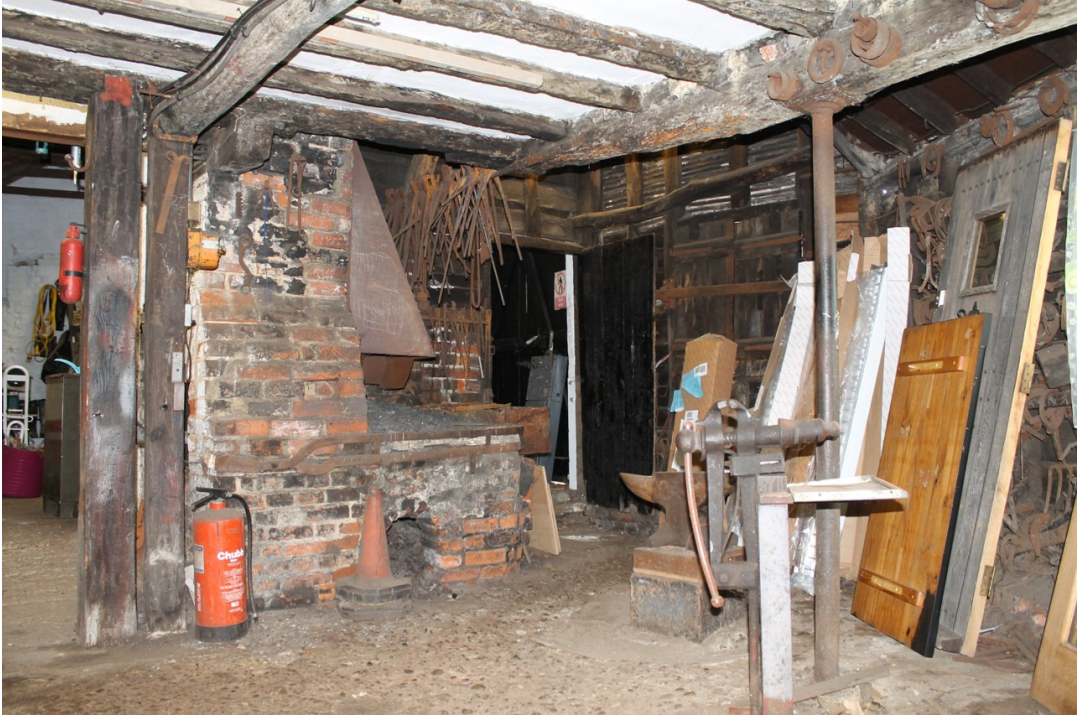
Photograph 19 Extension A with forge located in extension B behind. The wall plates of extension A are supported on iron columns and the replacement timber posts to the left of the forge chimney stack. The corner post of the timber frame has been removed to allow the forge to be worked - view north-east.
