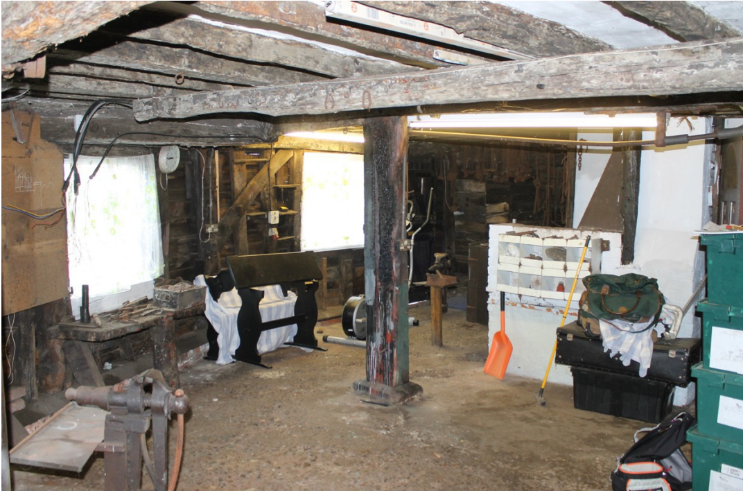
Photograph 17 Extension A built against the south-east wall of the cross-wing - view west.
