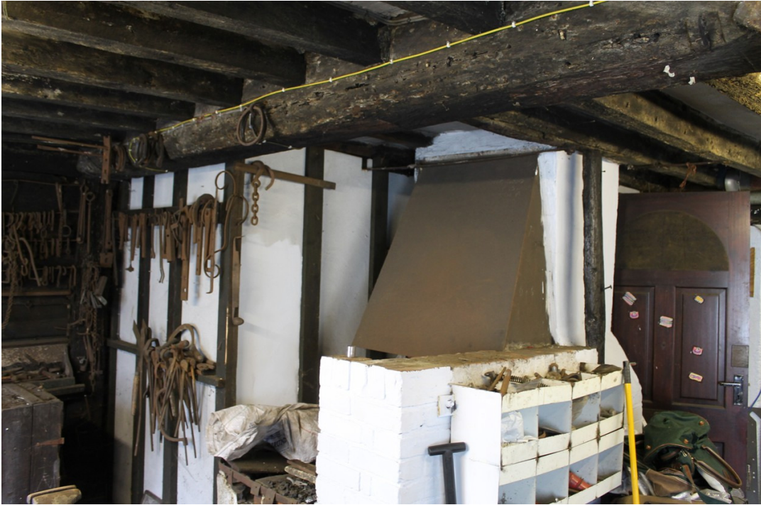
Photograph 11 Rear bay of the cross-wing with one of the two forges and the inserted stud walls behind. The bridging beam has chamfered edges and stepped stops - view north.
