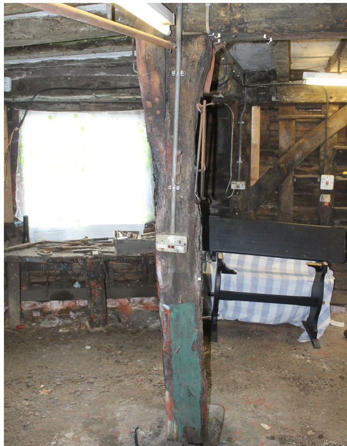
Photograph 12 Intermediate post with jowled head carrying the bridging beam between the front and rear bays of the cross-wing - view south.
