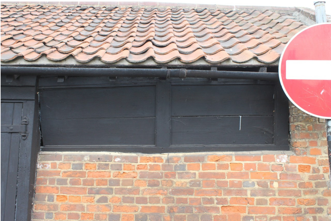
Photograph 8 Window openings below the eaves of the farrier's shop with internal top-hung shutters. These openings have been inserted into an earlier wall, either the boundary wall to the yard and garden or part of the free-standing structure shown on the 1838 Tithe map - view north-west.
