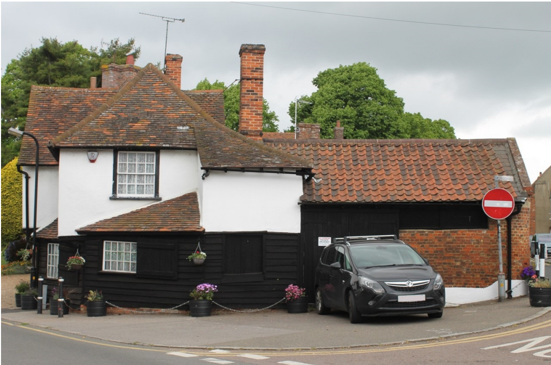
Photograph 3 South-east facing elevations of The Forge with extension A projecting from the cross-wing and the single-storey components of extension B wrapped around its base. The farrier's shop is to the right of the main range - view north-west.
