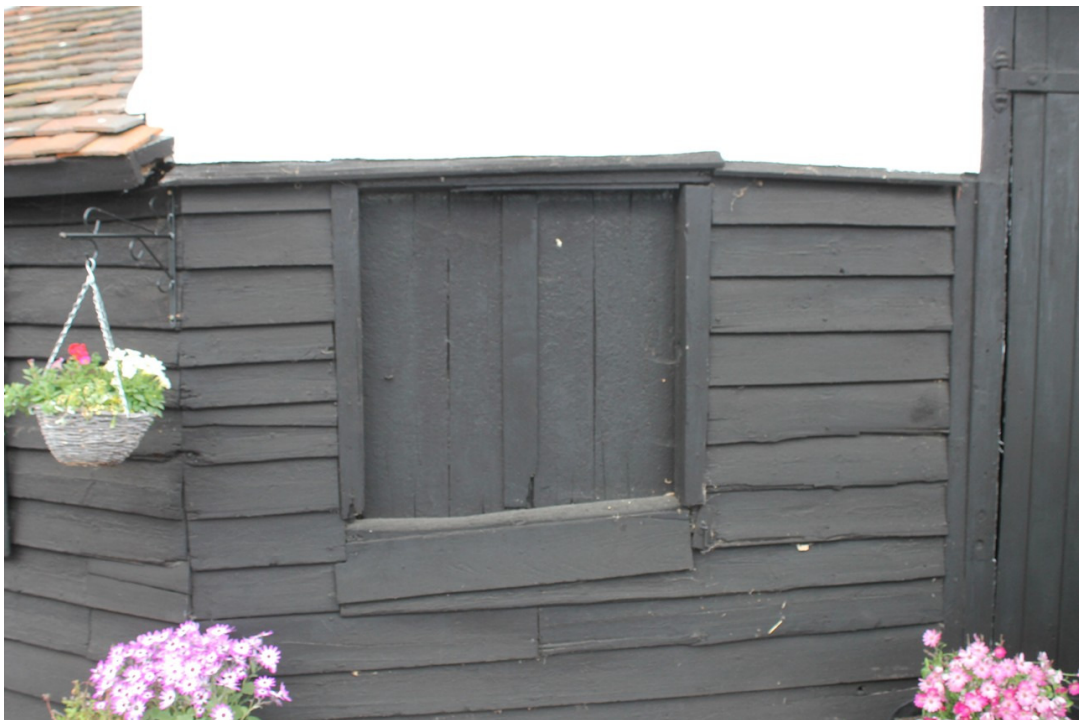
Photograph 6 The glassless window opening in extension B with internal side-hung shutters. The farrier's shop is to the right - view north-west.
