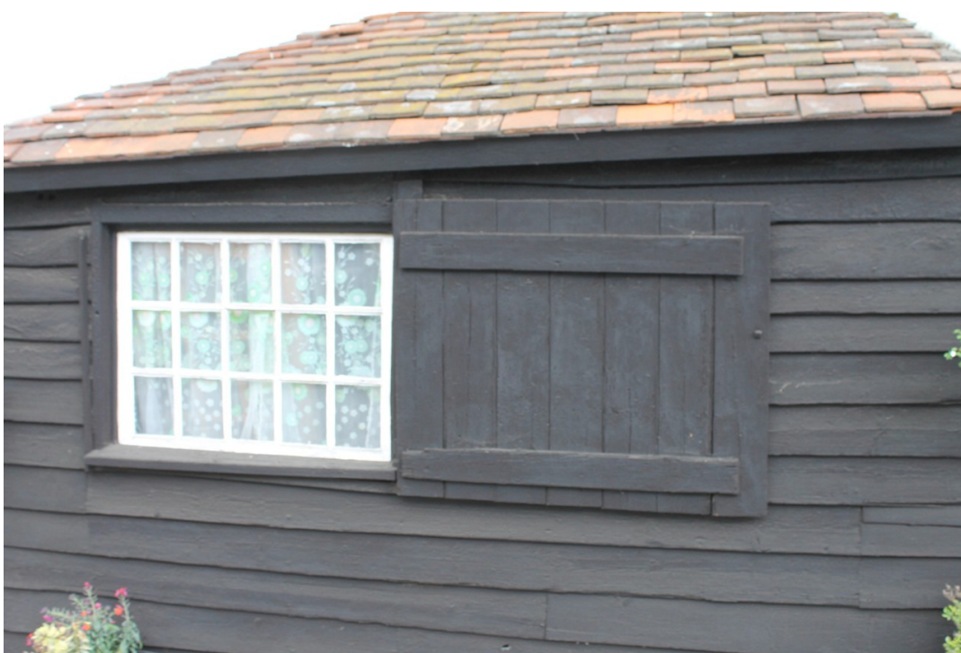
Photograph 5 One of the two window openings in extension B with a side-hung shutter - view north.
