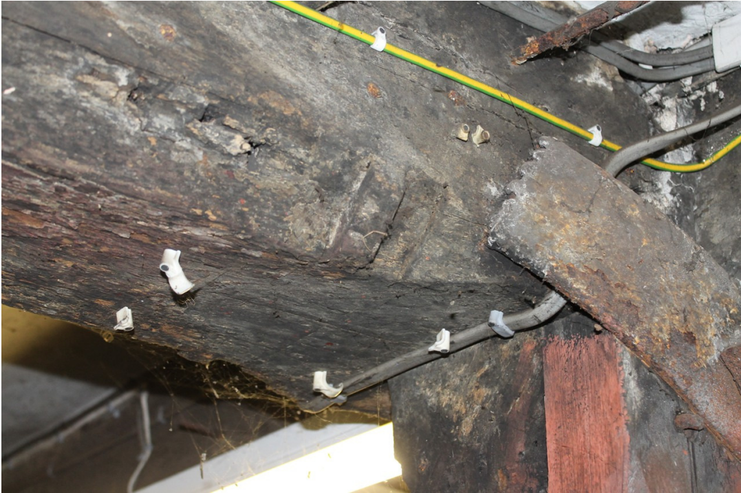
Photograph 13 Detail of the bridging beam between the front and rear bays of the cross-wing, showing the chamfered edges and stepped stops - view east.
