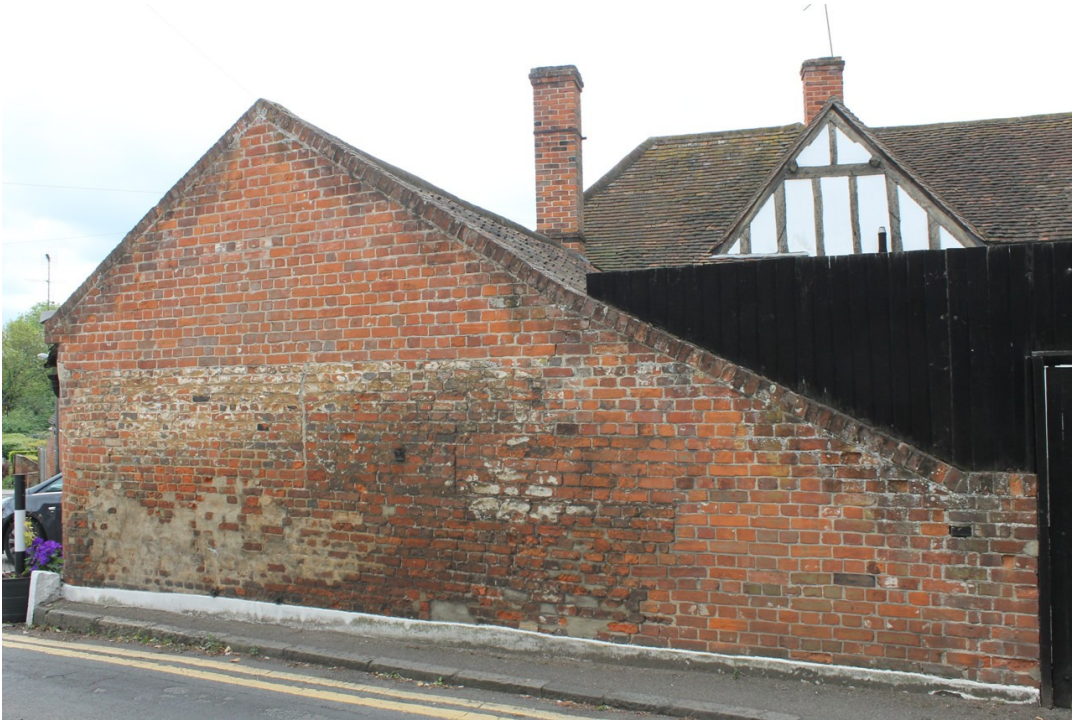
Photograph 9 North-east wall of the farrier's shop and the lean-to. Changes in the brickwork clearly indicate that the gable is constructed upon an earlier wall, either the boundary wall to the old yard and garden or part of the free-standing structure shown on the 1838 Tithe map - view west.
