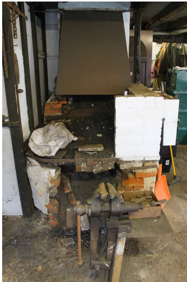
Photograph 16 Forge in cross-wing - view north-east.
