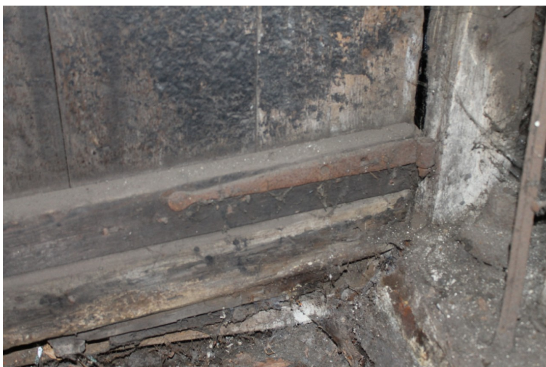
Photograph 26 Detail of simple strap hinge to door in extension B, likely to have been forged on the premises.
