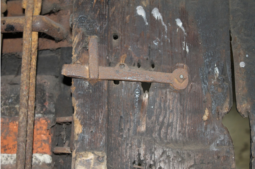
Photograph 27 Detail of simple latch to door in extension B, likely to have been forged on the premises.
