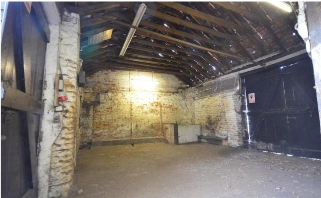
Photograph 29 Interior of the farrier's shop viewed from the smithy showing the gable constructed upon the earlier yard wall - view east. (Copyright Fenn Wright)
