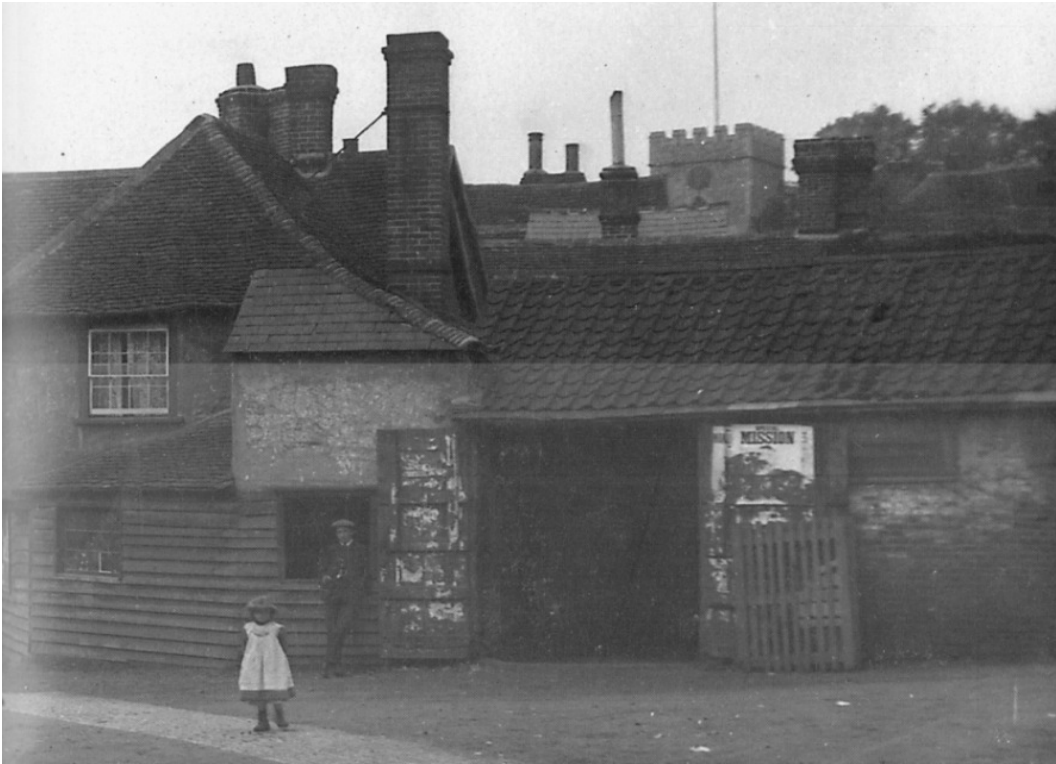
Historic Photograph 3 The Forge, Chipping Hill, c 1910 (Marriage, 1995).
