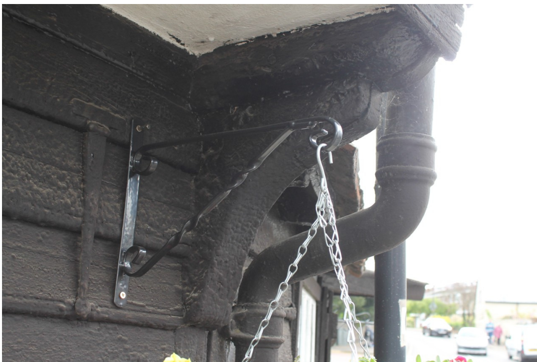
Photograph 4 Original bracket supporting the jetty of the cross-wing above The Forge - view south-east.
