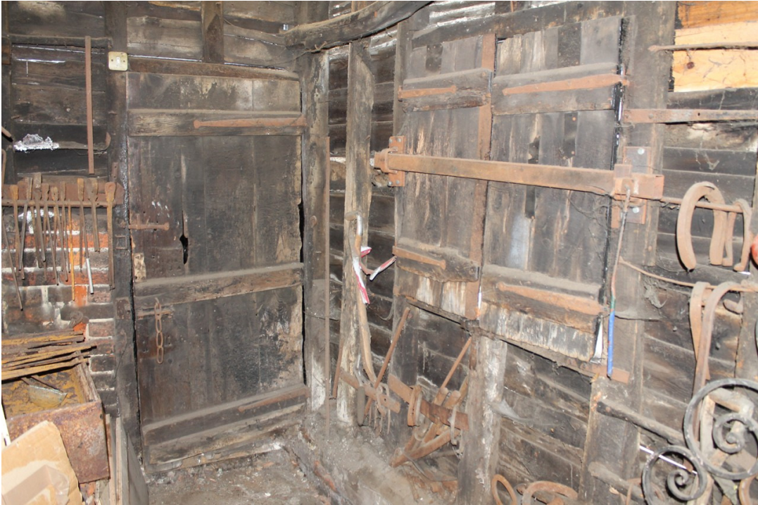
Photograph 23 The third section of the exterior wall to extension B showing the original timber shutters to the right and the door to the farrier's shop - view east.
