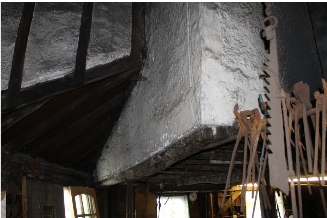
Photograph 20 The north-east corner of extension A viewed from extension B where the corner post of the timber frame has been removed to allow the forge to be worked. The original render of simple panels with textured decoration to extension A has been hidden and preserved by extension B - view west.
