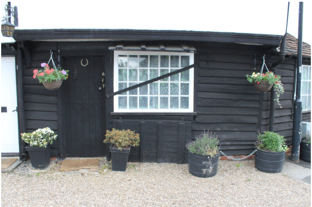
Photograph 7 The window opening in the cross-wing with top- and bottom-hung shutters that would have formed a counter from which the blacksmith sold items made at the smithy - view north-east.
