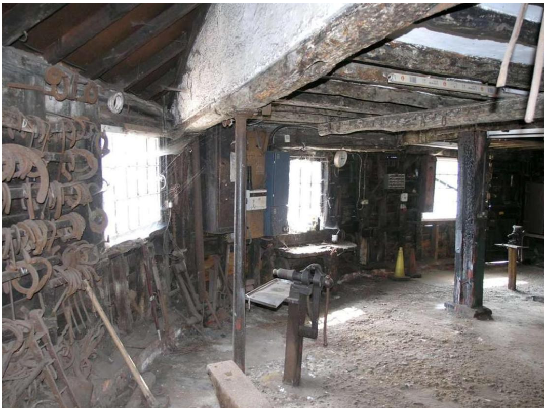
Photograph 22 The first and second sections of the exterior wall to extension B with extension A to the right - view south-west (Copyright John D Wood).
