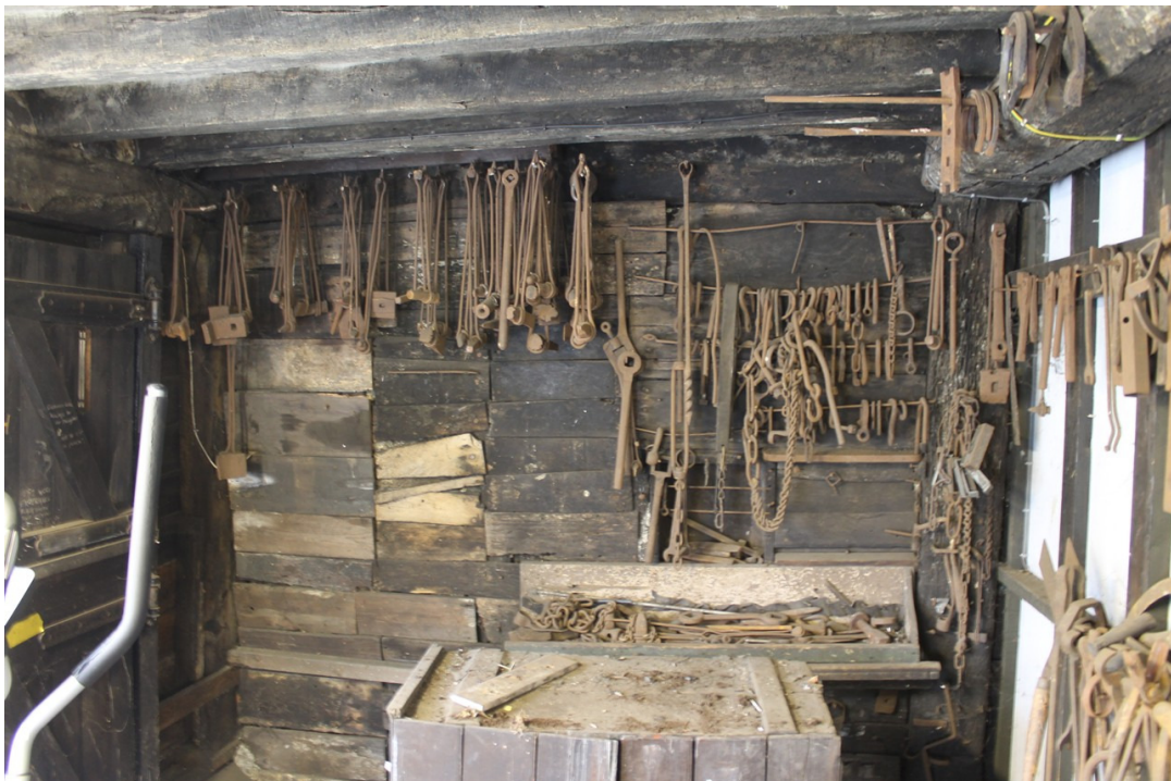
Photograph 10 North-west wall of the front bay to the cross-wing with the original doorway to the left and the inserted stud wall to the right. The studs of the wall frame are concealed behind the plank covering - view north-west.
