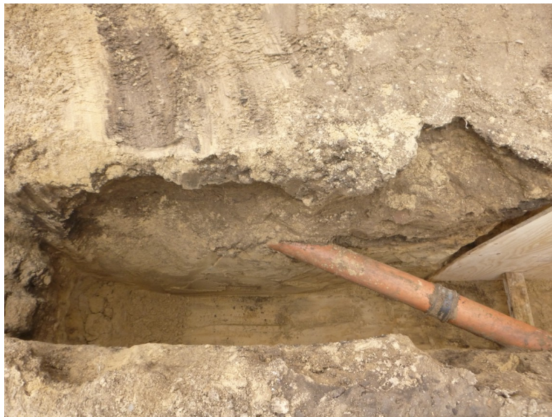
Photograph 1 Trench shot showing modern services
