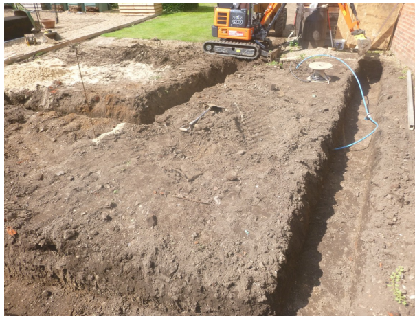
Photograph 1 Site shot – looking west southwest
