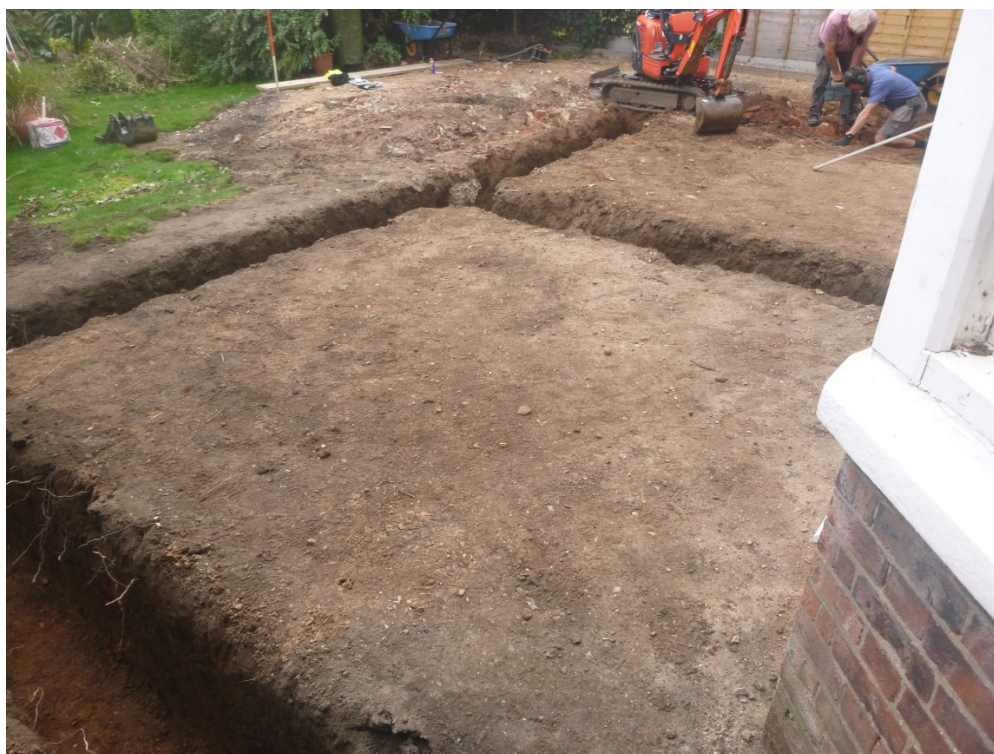
Photograph 1 Context shot showing trenching – looking southwest
