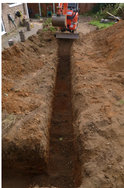
Photograph 1 Southern branch of foundation trench – looking east
