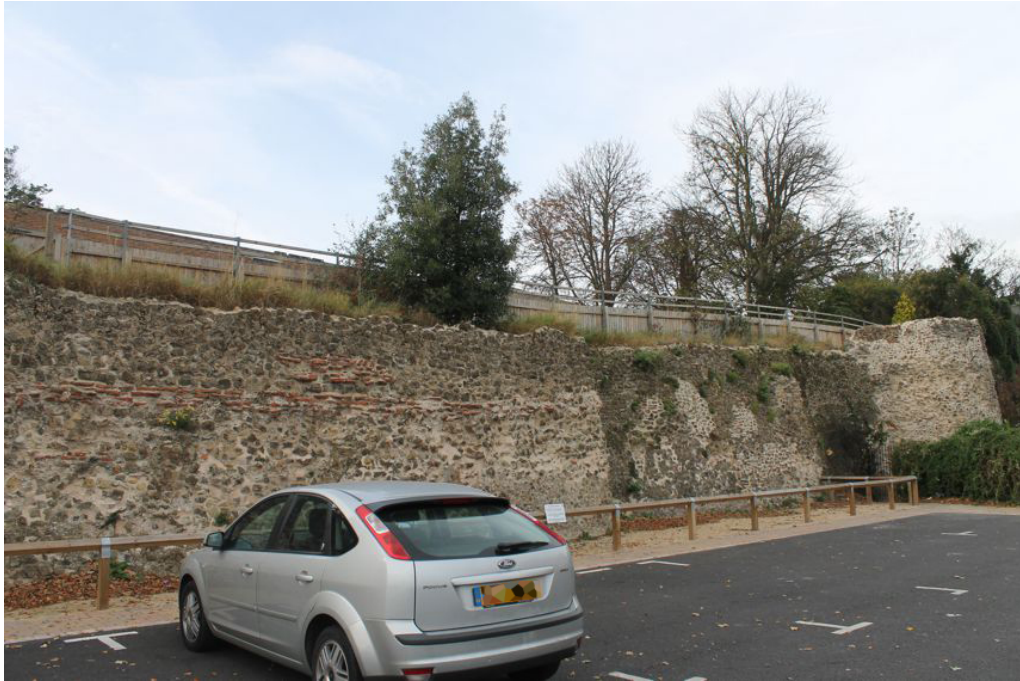
Photograph 13 Section 11 (to right of frame) and part of Section 10 (drawn in Figs 5 and 6). All after conservation. Photograph taken facing north-west.
