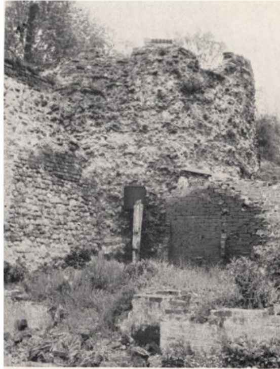
Photograph 2 Photograph of Bastion 1 from Roman Colchester (Hull 1958, pl XI D). Note the remains of later foundations on top of the bastion. Photograph taken facing north-west.
