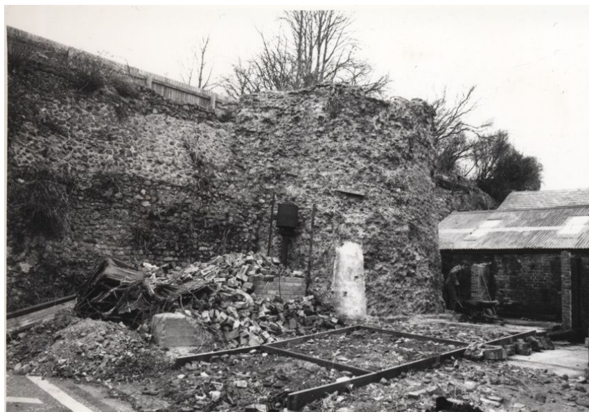
Photograph 3 Section 11 and Bastion 1, taken in 1986 after demolition of a nearby building. Photograph taken facing north-west.
