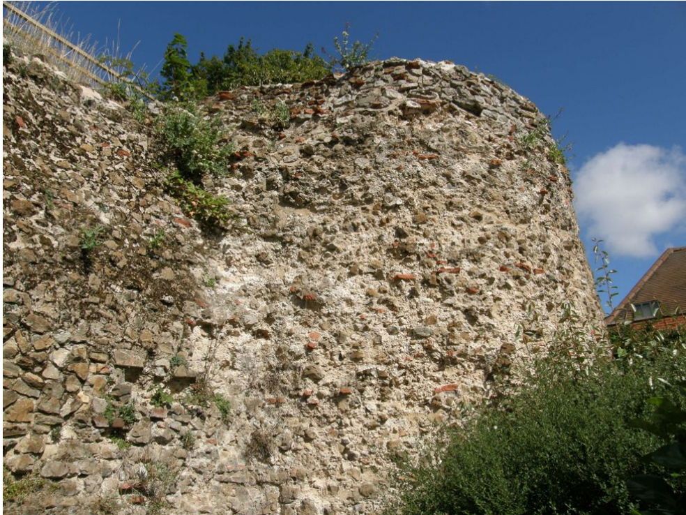
Photograph 6 Section 11 of the town wall, including Bastion 1, prior to removal of overgrowth. Photograph taken facing north-west.
