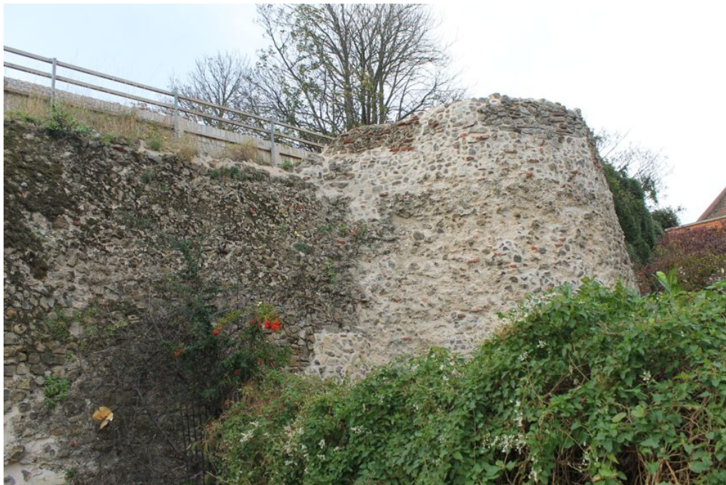
Photograph 12 Section 11 and Bastion 1 after conservation. Photograph taken facing north-west.
