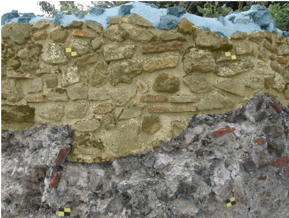
Photograph 7 Section of the top of the bastion photographed during survey (for location see Fig 4). Three phases highlighted; at the top, the modern lime mortar capping, in the middle, stones and re-used Roman tile bound in concrete, and at the bottom, the original bastion material of re-used Roman tile and septaria. Photograph taken facing west.
