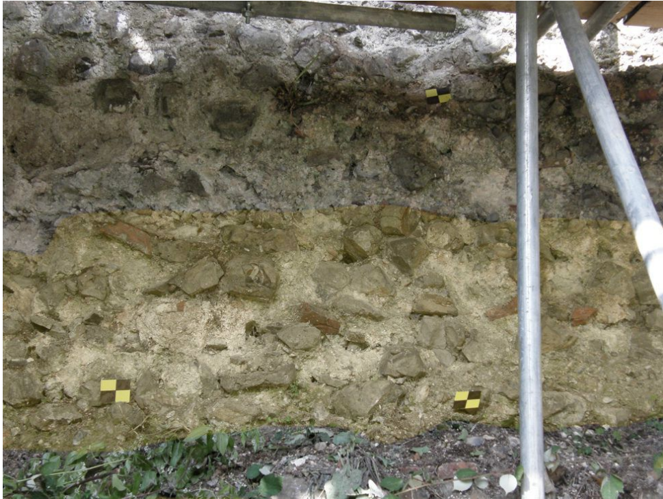
Photograph 8 Section of the base of the wall photographed during survey (for location see Fig 4). Highlighted section shows possible underpinning of wall below foundation. Photograph taken facing west.
