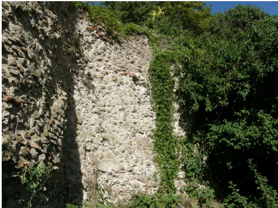
Photograph 11 Section of wall to the north of Bastion 1 prior to removal of overgrowth. Remains of tile courses visible towards the top of the wall. Photograph taken facing west.
