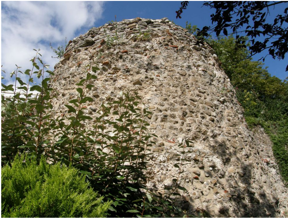
Photograph 10 Bastion 1 prior to removal of overgrowth. Photograph taken facing west.
