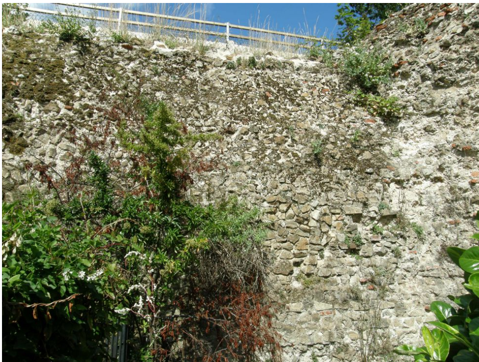
Photograph 9 Wall to the south of Bastion 1 prior to removal of overgrowth. Photograph taken facing west.
