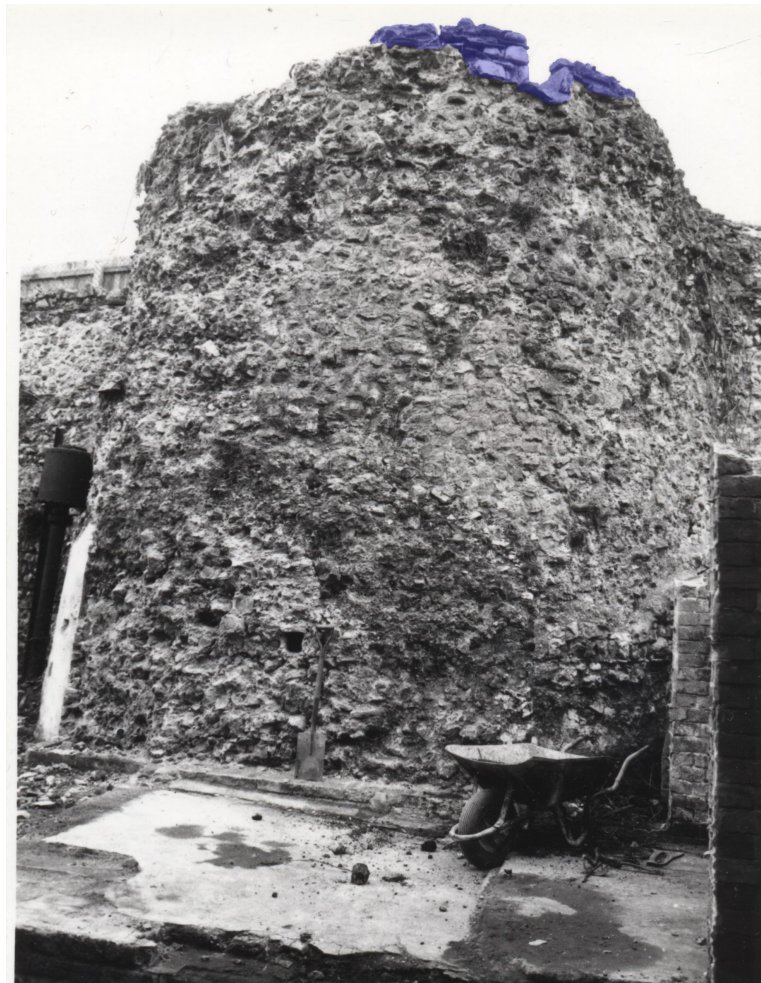
Photograph 5 Detailed shot of Bastion 1, taken in 1986 after demolition of a nearby building. Highlighted in blue at the top of the bastion is the remains of a structure seen on mapping in 1848 and 1896. Photograph taken facing south-west.
