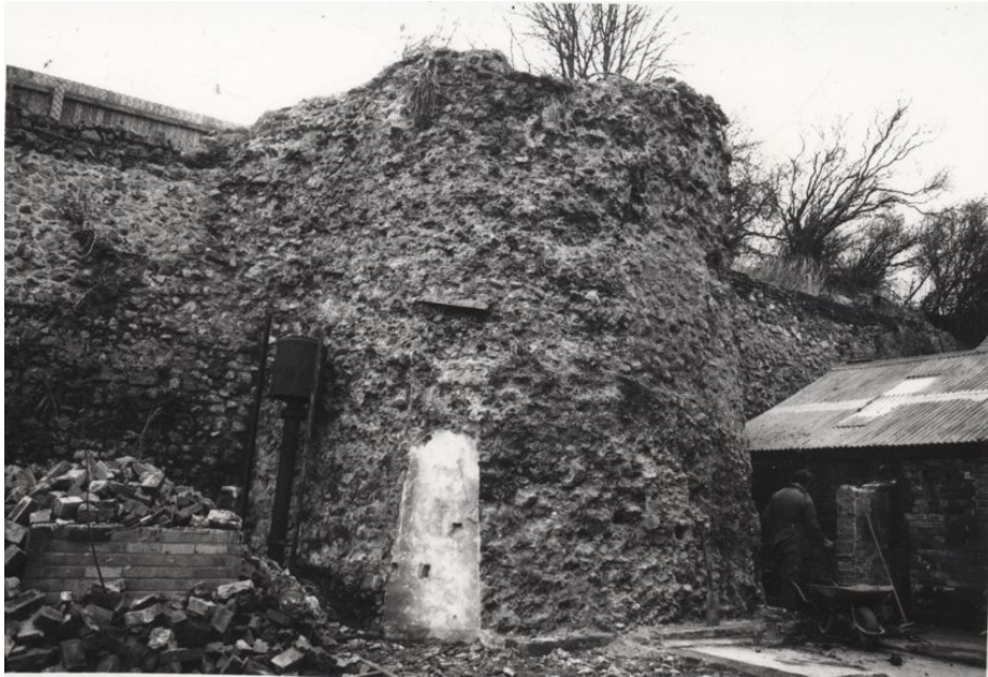
Photograph 4 Detailed shot of Bastion 1, taken in 1986 after demolition of a nearby building. Photograph taken facing north-west.
