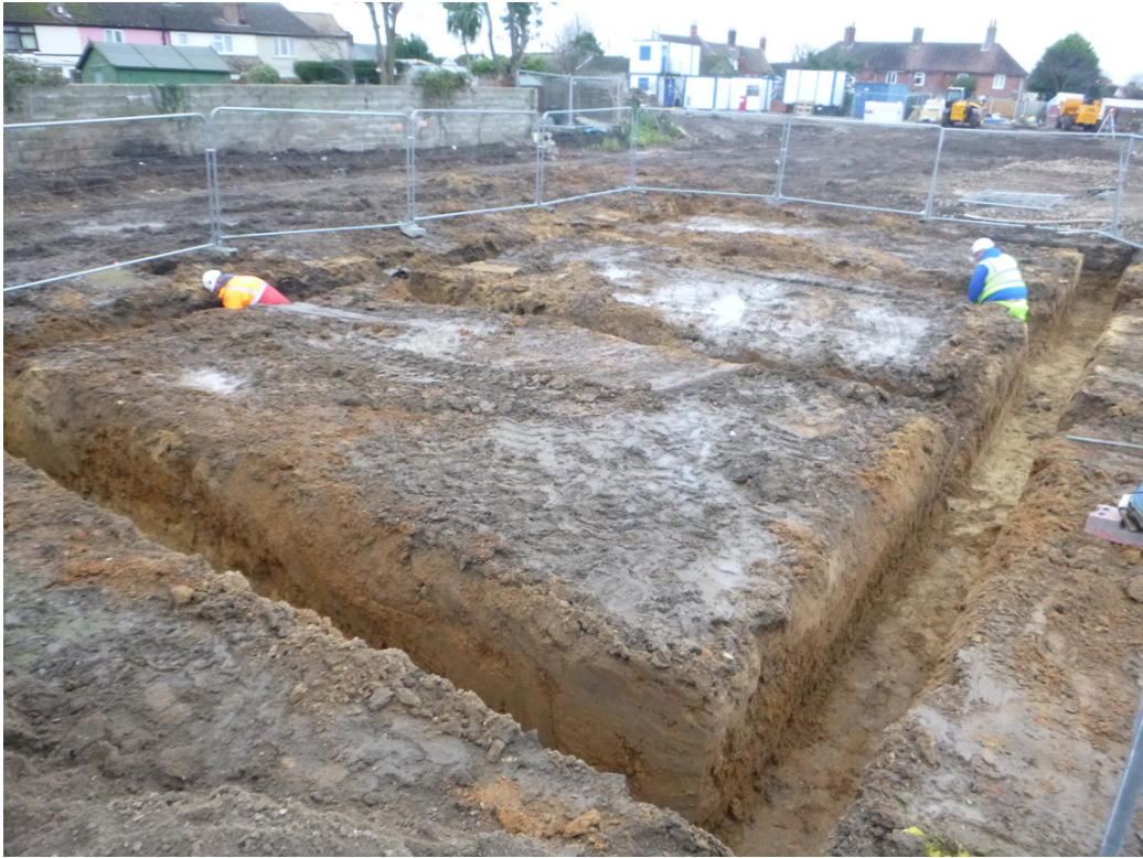
Photograph 6 Foundation trenches in the eastern corner of the development site, looking south
