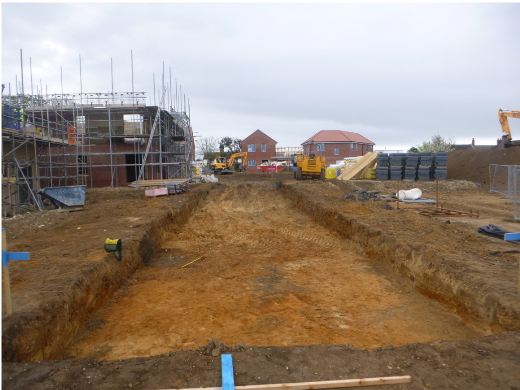
Photograph 7 Access road strip with F90 of the left-hand site, looking south
