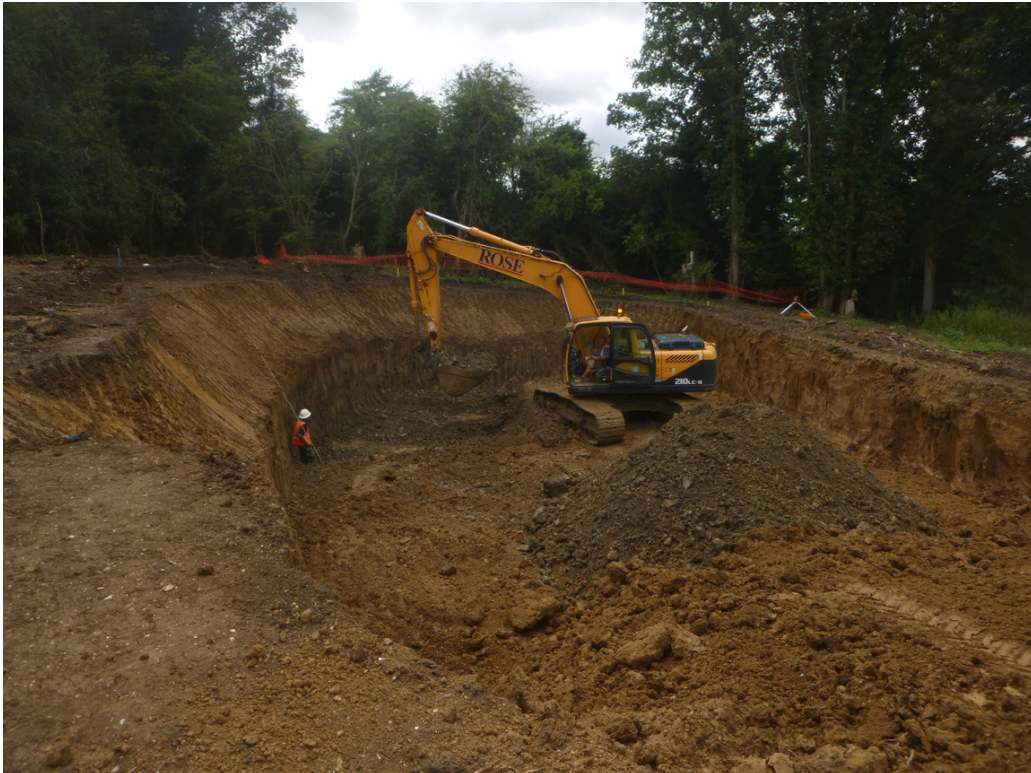
Photograph 8 Groundworks for the attenuation tank, looking northwest.
