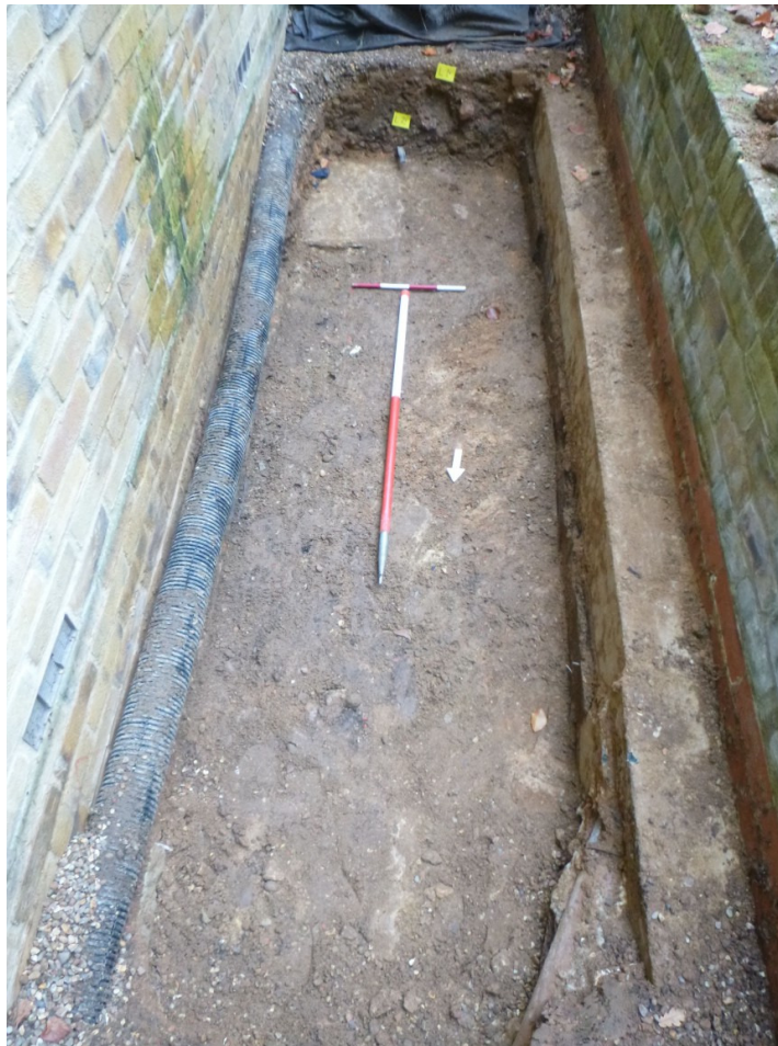
Photograph 1 Level reduction – looking south
