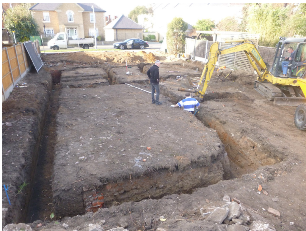
Photograph 1 Excavation of the foundation trenches, looking NW
