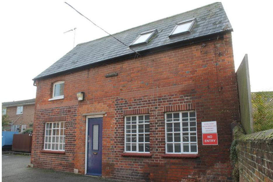
**Photograph 12** North-west elevation of outbuilding. Bricked in openings visible on either side of the door. Photograph taken facing east.
