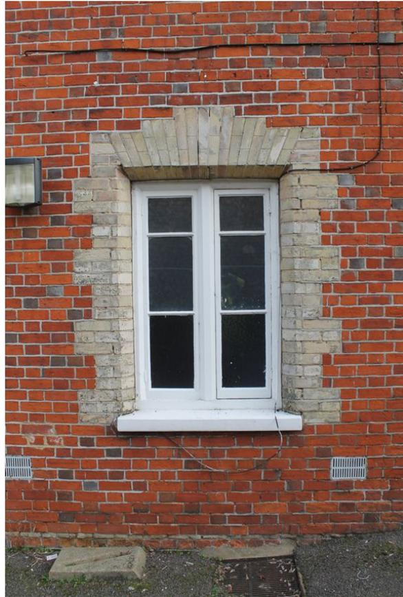
**Photograph 6** Original window and dressing on the south-west elevation of the Police Station. Photograph taken facing north-east.
