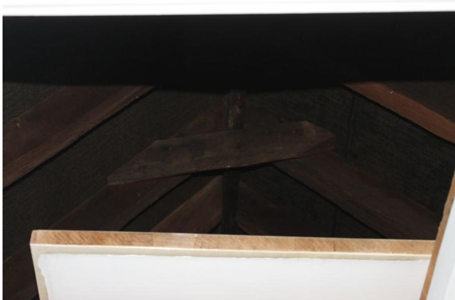
**Photograph 15** Detail of roof of outbuilding through loft hatch. Machine-cut rafters and upper collar visible. Photograph taken facing north-east.
