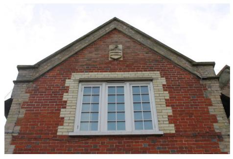
**Photograph 5** North-west gable end of the Police Station, showing the carved Essex crest original to the building, and the later inserted window with modern brickwork surrounding it. Photograph taken facing south-east.
