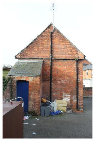
**Photograph 13** North-east elevation of outbuilding. Small bricked-in opening visible, and surviving lean-to. Photograph taken facing southwest.
