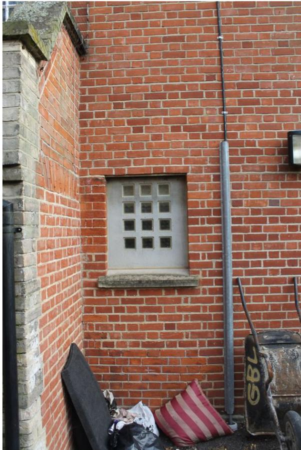
**Photograph 11** Inserted concrete-framed window on south-west elevation of extension to Police Station. Photograph taken facing north-east.
