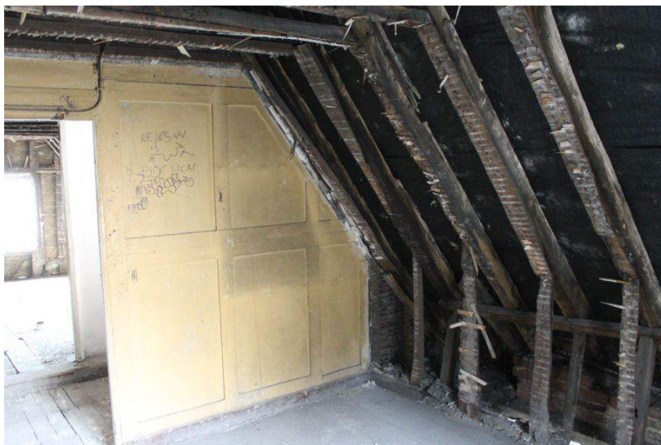
Photograph 34 East room on second-floor of Building A. smoke-blackened rafters visible. Photograph taken facing north-west.
