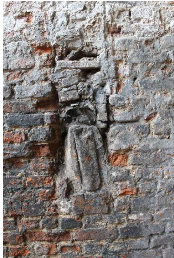
Photograph 48 Detail of worked stone in northern wall of cellar.
