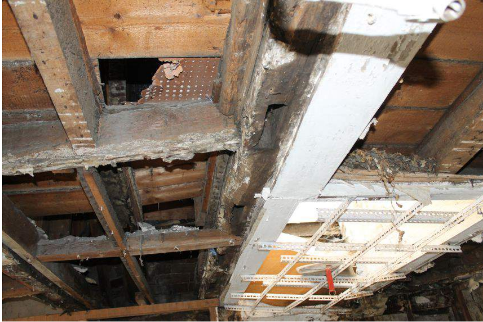
Photograph 22 Underside of north-south binding-beam supporting the second-floor, showing unused mortices. Photograph taken facing north.
