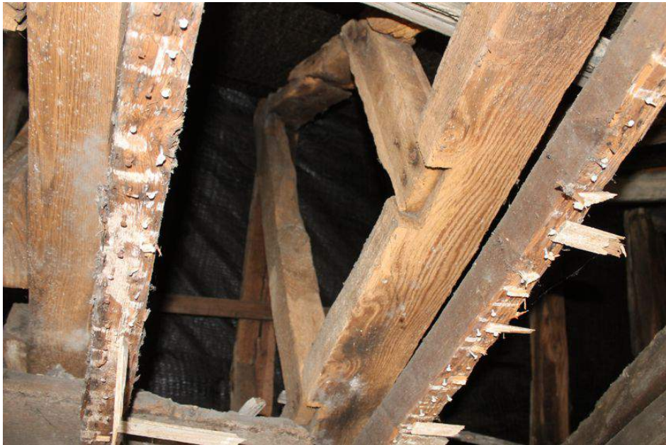
Photograph 31 Queen and king-posts nailed in place on the two westernmost collars in Building A.
