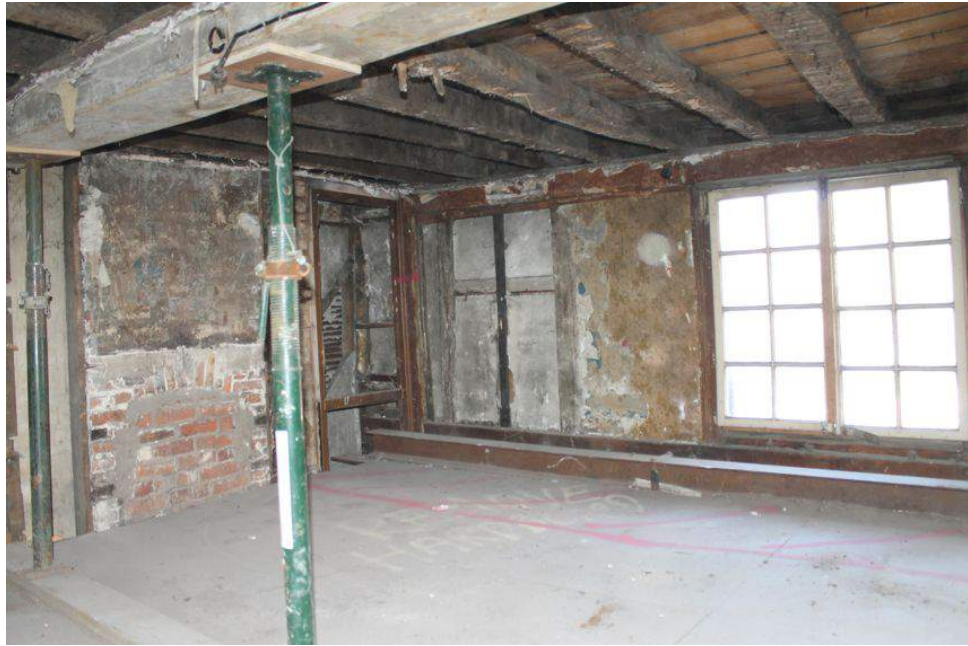
Photograph 54 First-floor of Building B, showing blocked fireplace and raised floor level. Photograph taken facing south-west.
