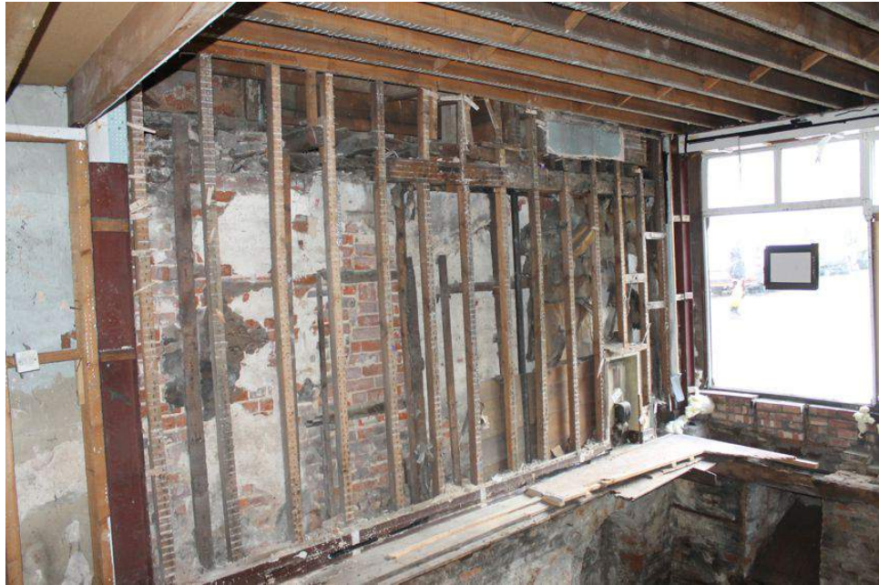
Photograph 52 Southern elevation of ground-floor of Building B, showing timber-frame partially surviving but obscured by later brickwork. Partially surviving girding-beam visible. Photograph taken facing south-west.
