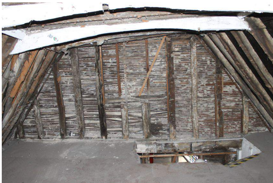
Photograph 64 East gable end in Building B, showing inserted window opening that has been covered in lath and plaster. Photograph taken facing east.
