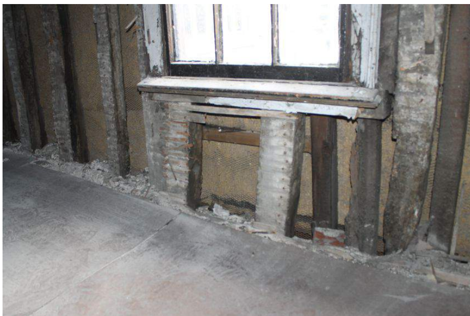
Photograph 65 Cut studs beneath inserted window in west gable end of Building B. Diamond mullions visible on left stud. Photograph taken facing south-west.
