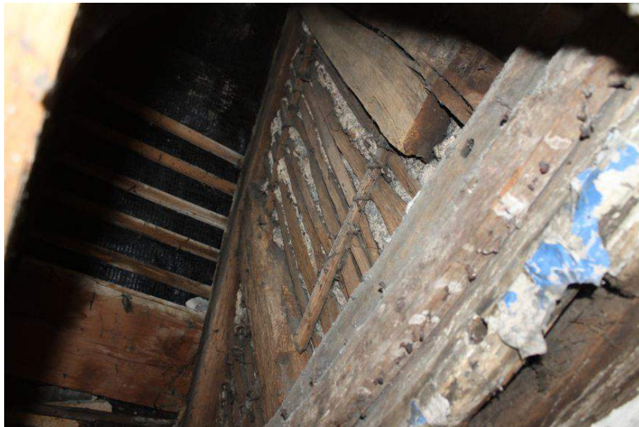
Photograph 33 Possible original rudimentary lath and plaster on west side of the modern skylight in Building A. Photograph taken from first-floor looking up.
