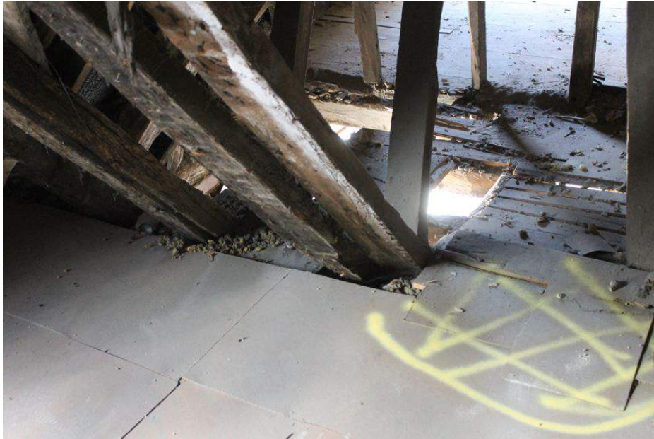
Photograph 66 Two rafters rising from one point on wall-plate to north of Building B. Photograph taken facing north-west.
