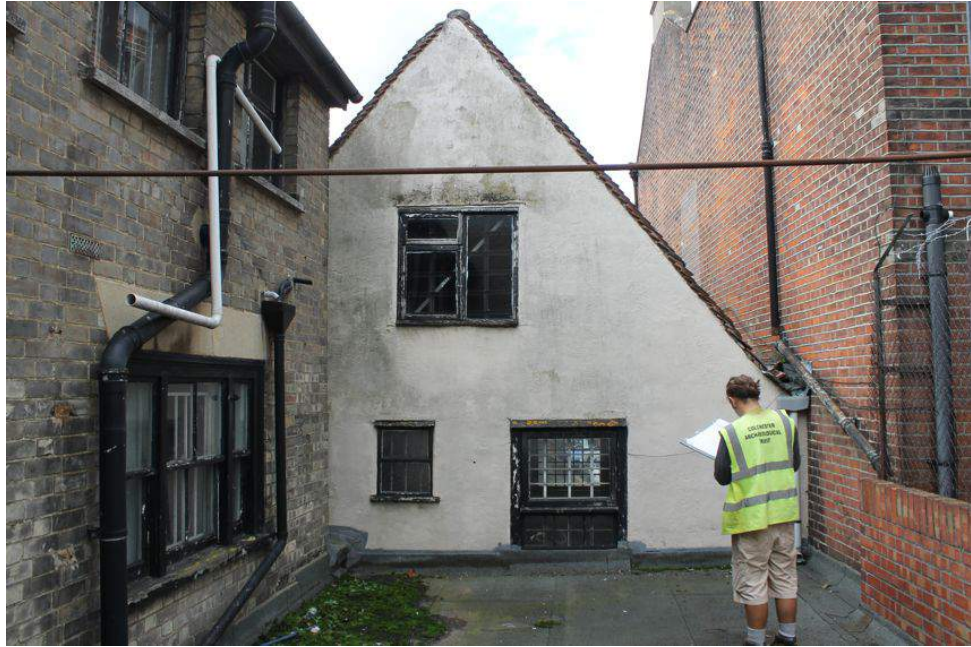
Photograph 3 Eastern elevation of Building A. Photograph taken facing west.
