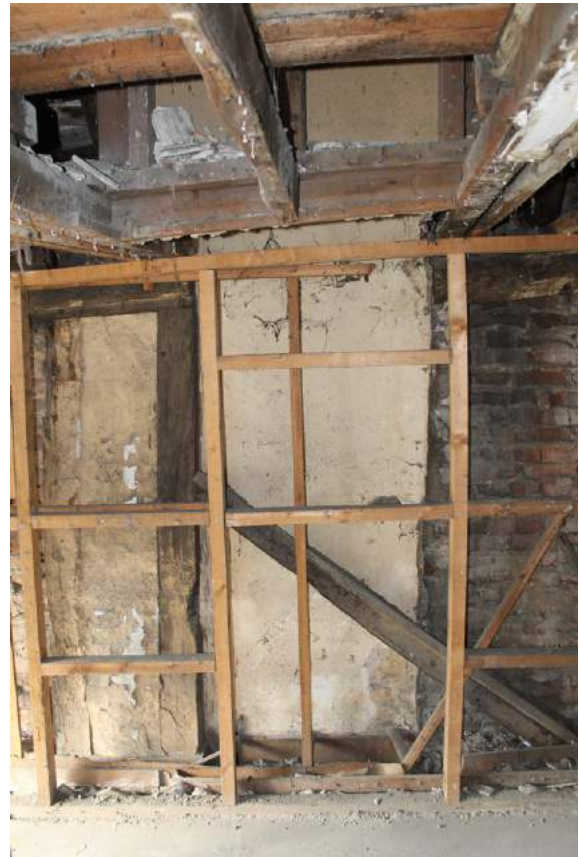
Photograph 17 Wall-plate cut and lath and plaster added behind on first-floor of Building A. Photograph taken facing north.
