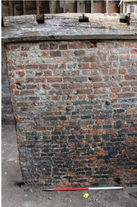
Photograph 49 Detail of dividing wall in cellar, showing two phases of brickwork. Photograph taken facing south.
