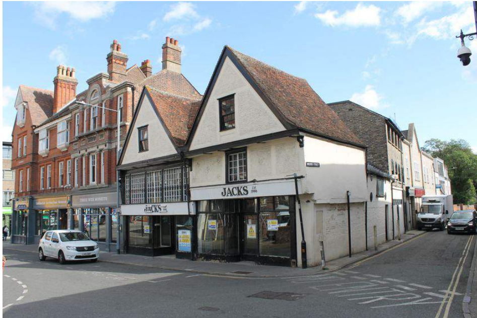
Photograph 36 Entire site, showing Buildings A, B, C and D. Underbuilding in brick below Building B's southern jetty visible. Photograph taken facing north-east.
