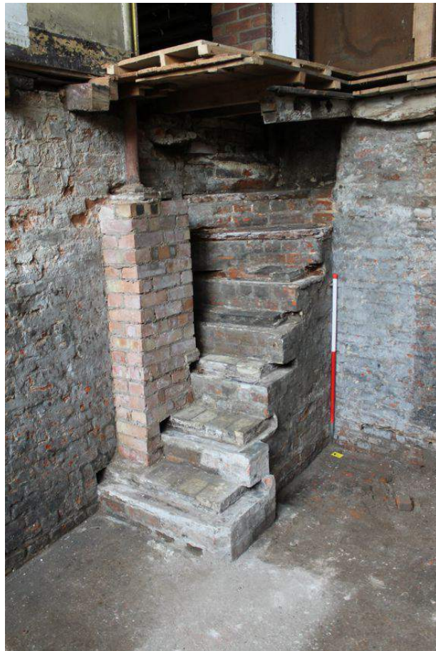
Photograph 43 Brick stairway into cellar. Also visible is brick pillar added to support metal post. Photograph taken facing north-east.
