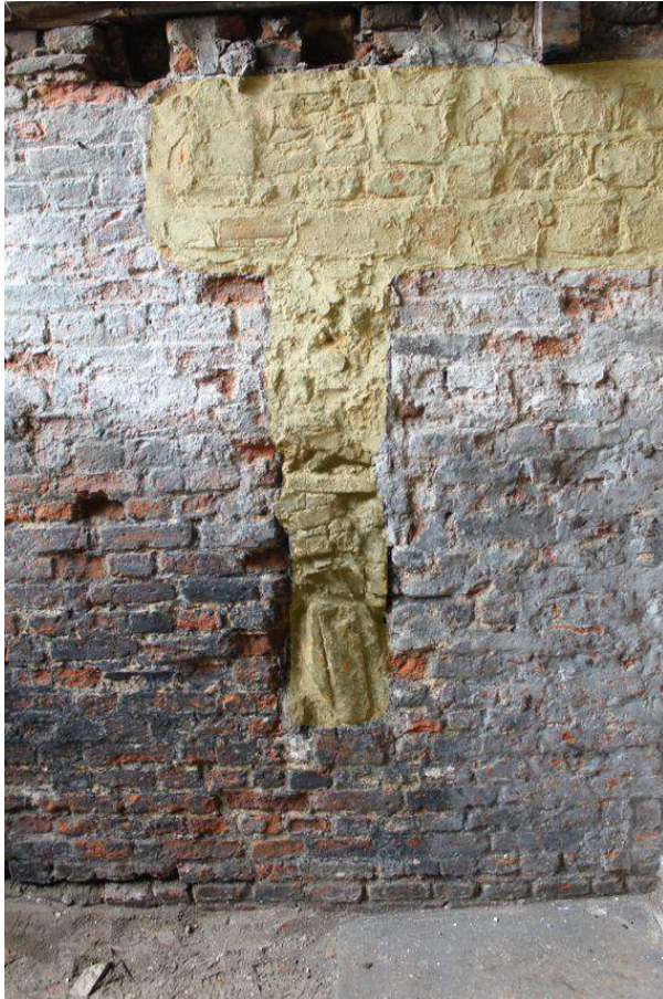
Photograph 47 Northern elevation of cellar, with repaired section of wall highlighted. Photograph taken facing north.
