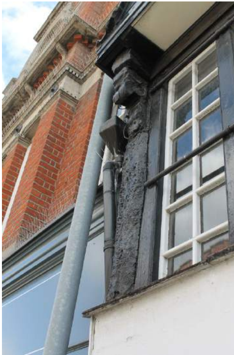
Photograph 5 North-west corner-post supporting second-floor jetty. Note carved top. Photograph taken facing north-east.
