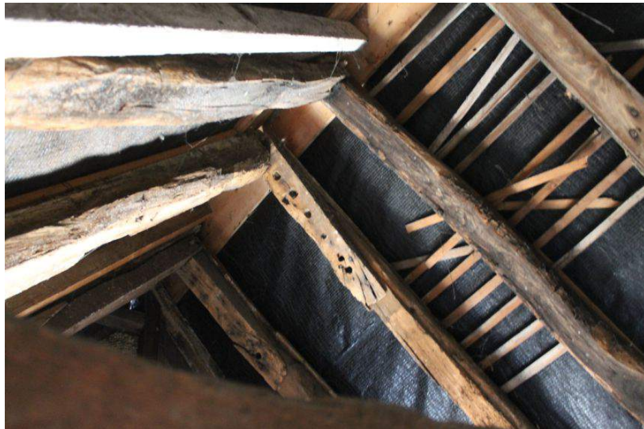
Photograph 61 Roof of Building B with scarf joints on rafters. Photograph taken facing south-east.
