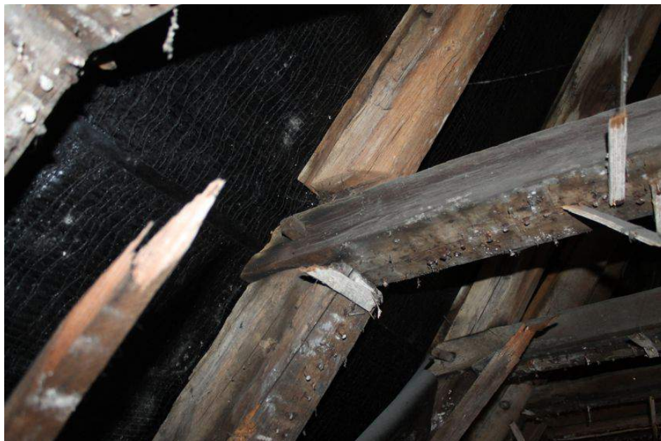
Photograph 25 Detail of peg joining collar and rafter in east room of Building A. Photograph taken facing north-east.
