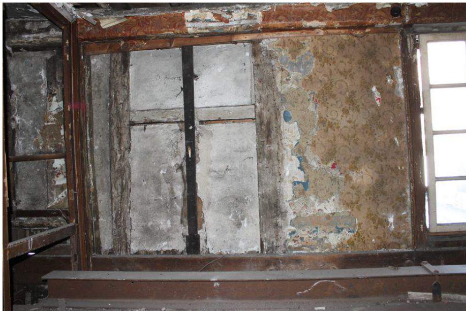
Photograph 58 Western wall of first-floor in Building B, showing possible infilled window opening. Photograph taken facing west.
