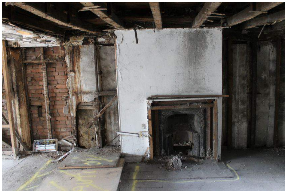
Photograph 16 Chimney-stack and later fireplace in first-floor of Building A. Photograph taken facing north.
