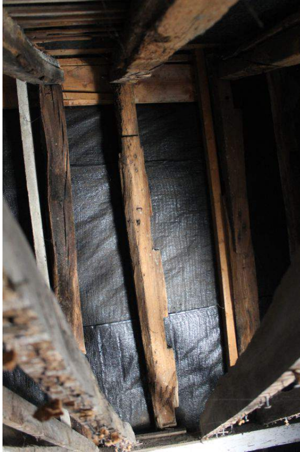
Photograph 62 Reused timber in roof of Building B, and evidence of smoke-blackening. Photograph taken facing south.
