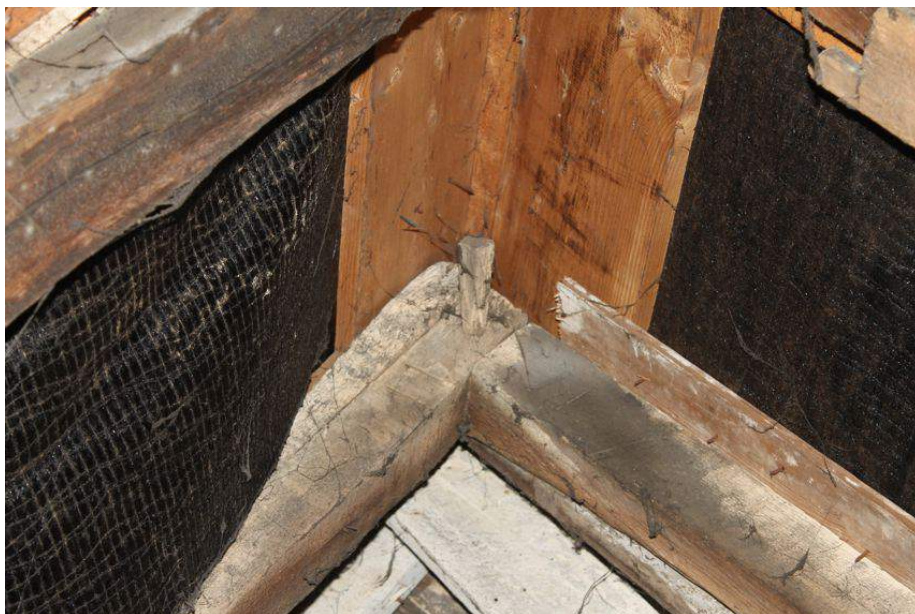
Photograph 63 Carpenter's mark "III" at apex of roof in Building B. Photograph 63 Carpenter's mark 'III' at apex of roof in Building B.
