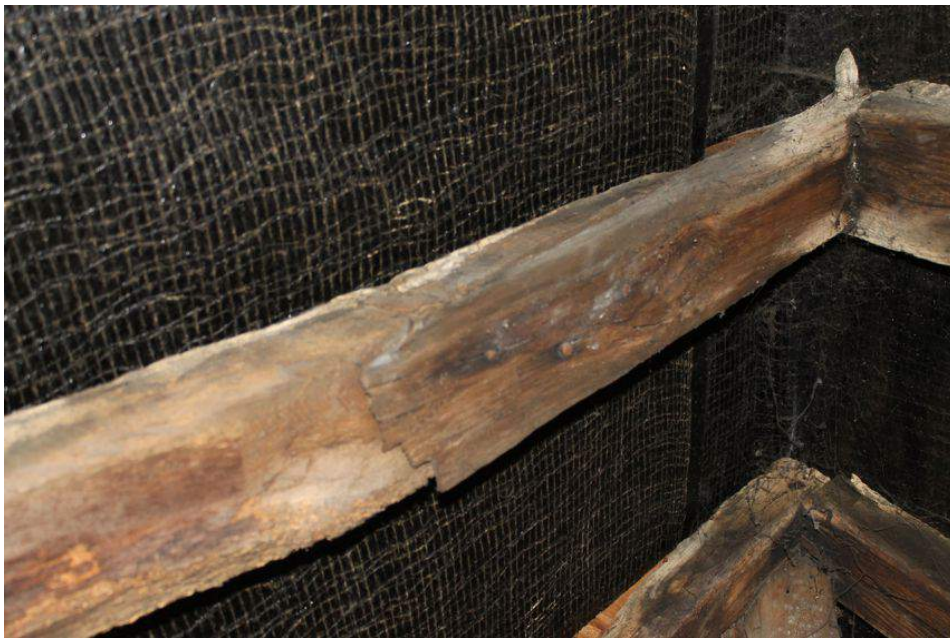
Photograph 24 Detail of rafters in Building A. Peg at apex visible, along with scarf joint/repair to rafter.
