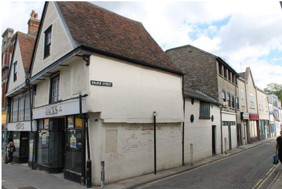
Photograph 40 Southern elevation of Building B, showing brick underbuilding. Photograph taken facing north-east.
