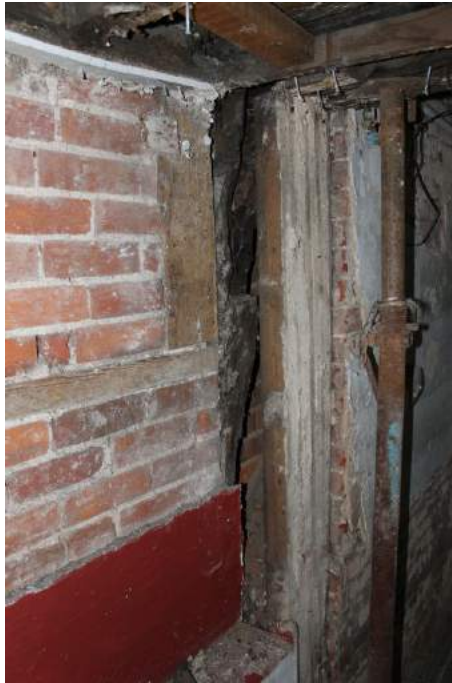
Photograph 7 Remains of north-east corner-post of Building A at the ground floor. Photograph taken facing north-east.
