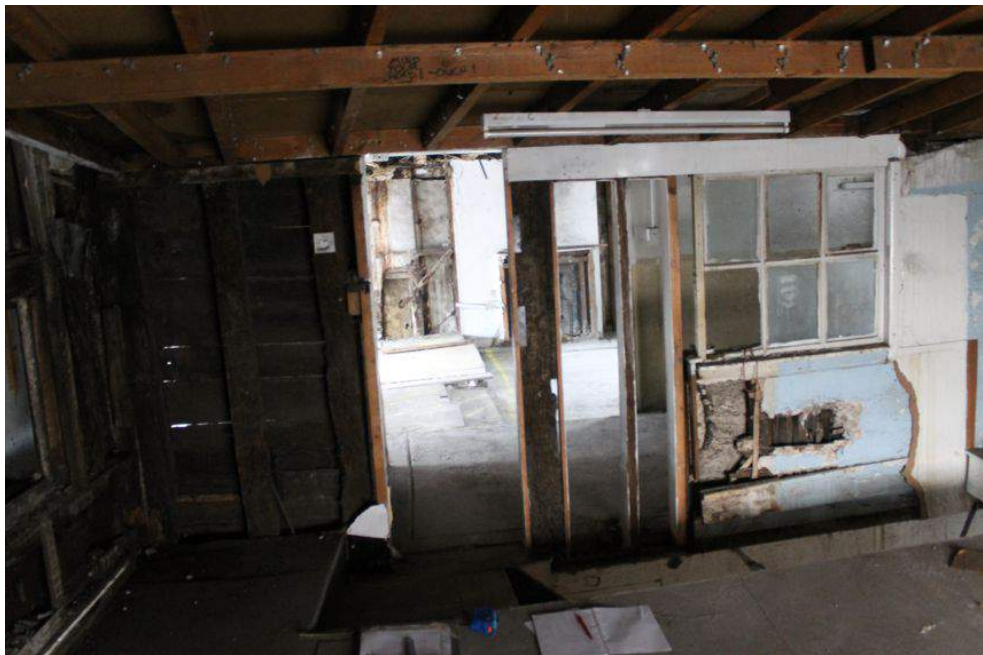
Photograph 4 Southern exterior elevation of the first-floor of Building A, with exposed lath and plaster below inserted window. Photograph taken inside Building C, facing north.
