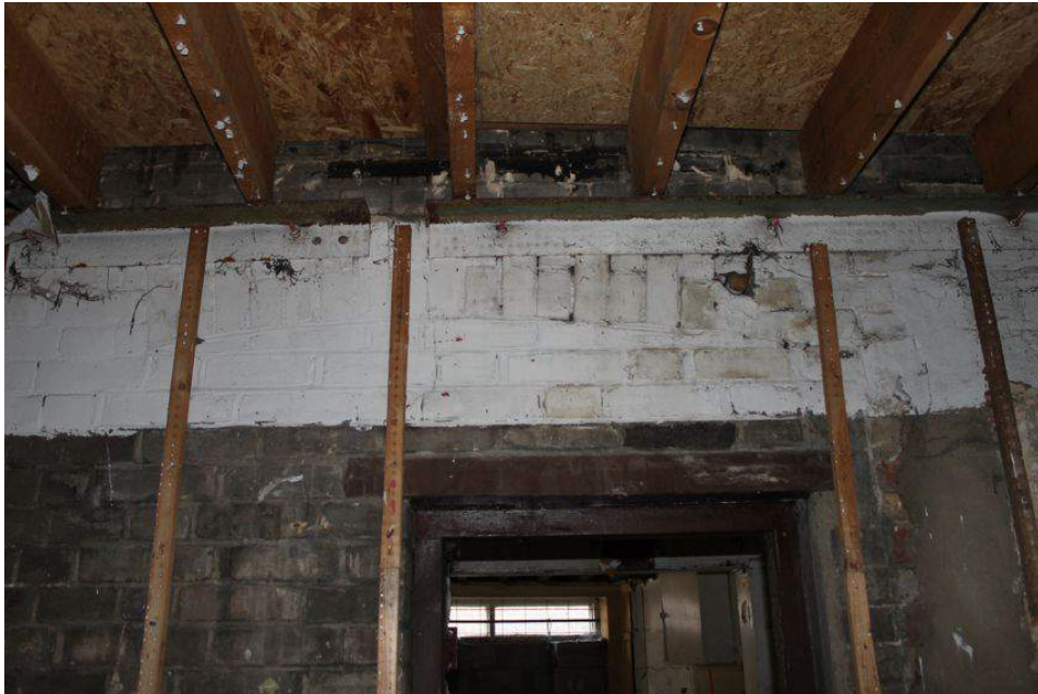
Photograph 71 Archway above inserted doorway in northern elevation of Building D, showing location of original window. Photograph taken facing south.
