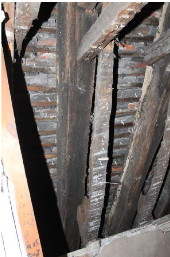
Photograph 26 Detail of smoke-blackening on rafters in centre of Building A. Photograph taken facing south-west.
