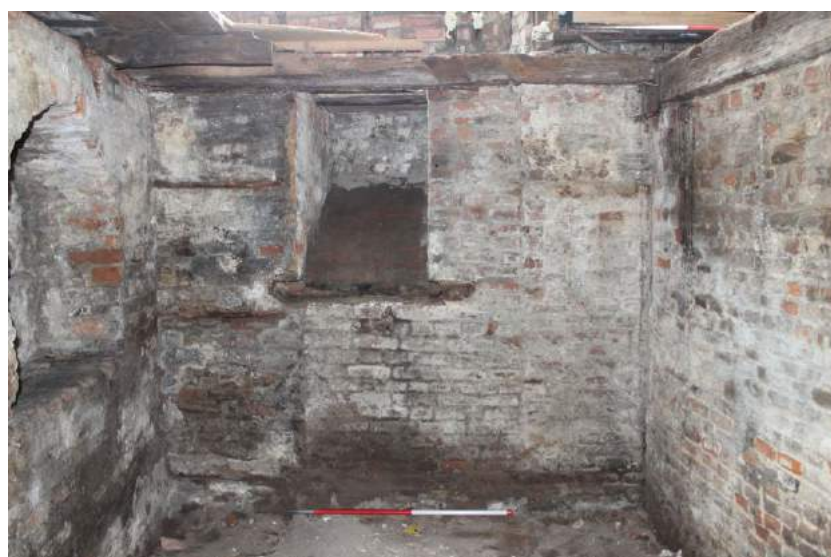
Photograph 45 Western elevation of southern room, showing coal chute inserted into an earlier, bricked up, opening. Photograph taken facing west.
