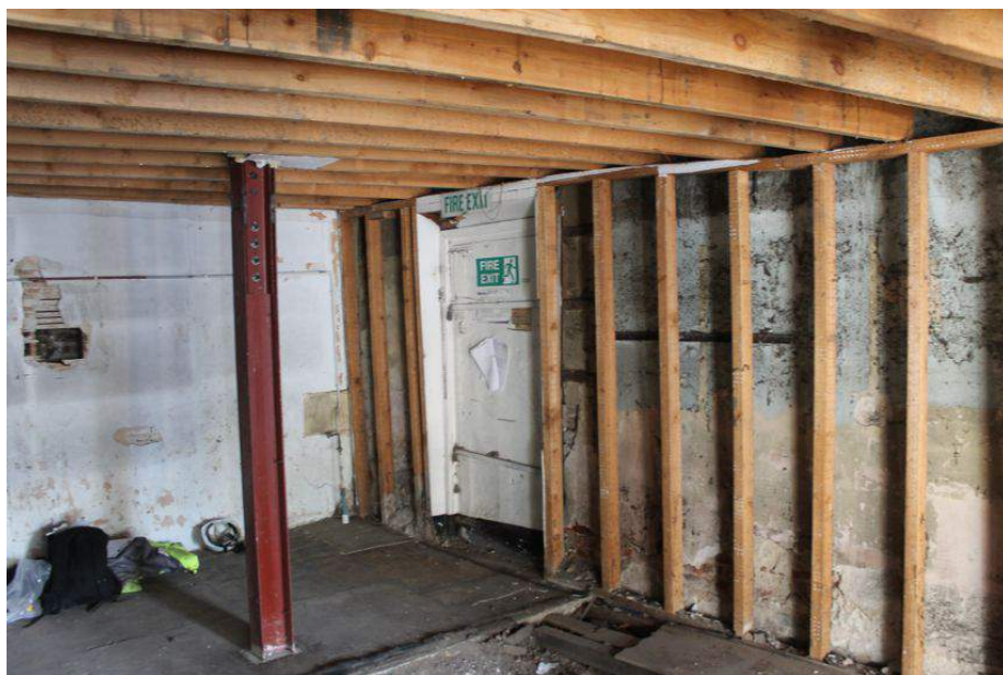
Photograph 68 Ground-floor of Building C, showing modern timber-frame in inside brickwork exterior. Photograph taken facing south-east.
