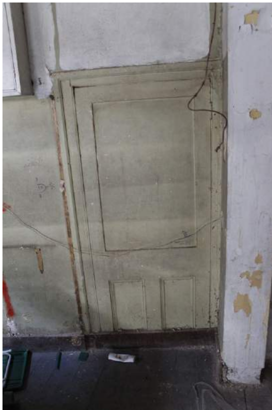
Photograph 73 Blocked door in western wall of ground-floor of Building D. Photograph taken facing west.
