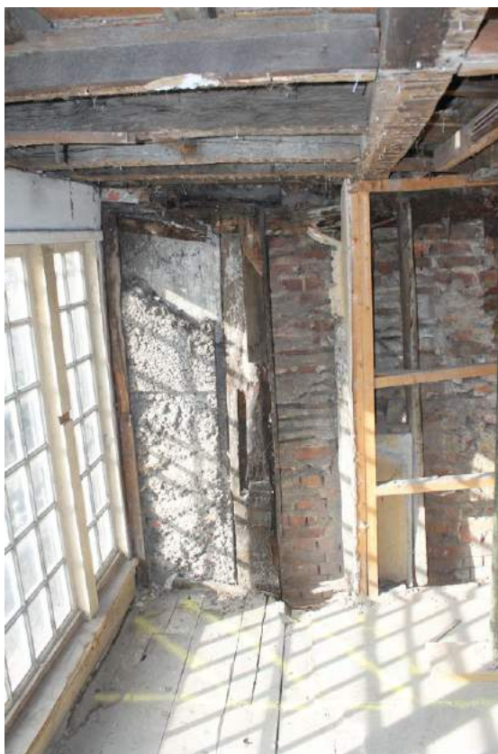
Photograph 18 North-west corner-post of Building A, showing unused mortice for arch brace and scarf joint above. Photograph taken facing north.
