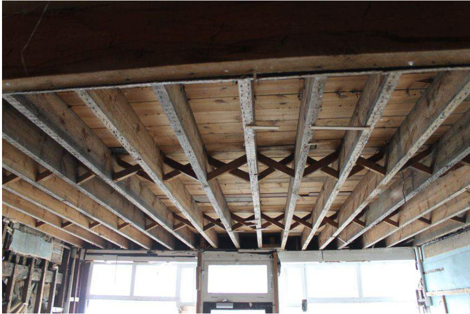
Photograph 53 Underside of raised first-floor in Building B, showing herringbone strutting supporting joists. Photograph taken facing west.
