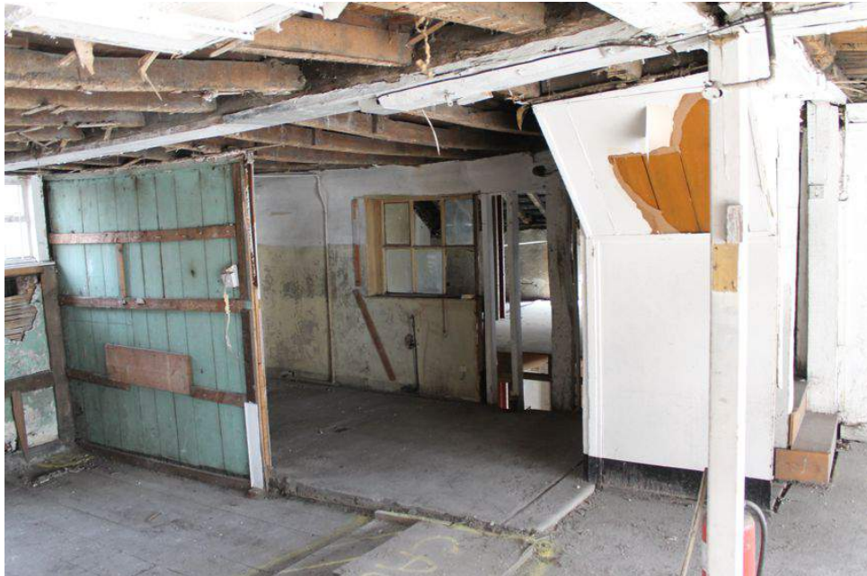
Photograph 21 First-floor of Building A, with binding-beams visible supporting floor above and modern post in centre of building. Photograph taken facing south-east.
