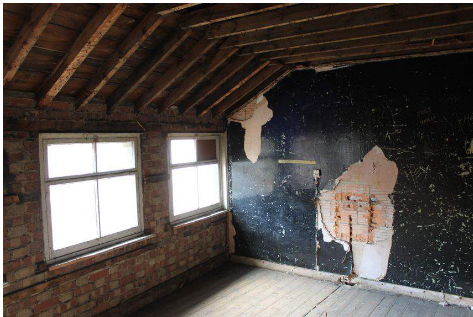
Photograph 76 Second-floor of Building D. Hollow-tile bricks visible beneath plaster to right. Photograph taken facing south-west.
