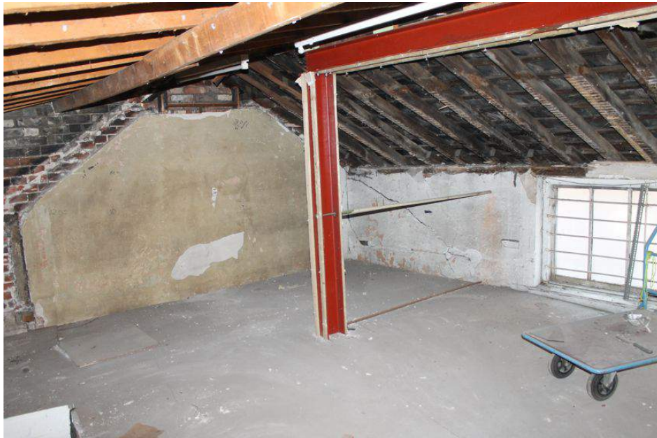
Photograph 69 First-floor of Building C, with original outline of roof against Building D visible. Photograph taken facing south-east.
