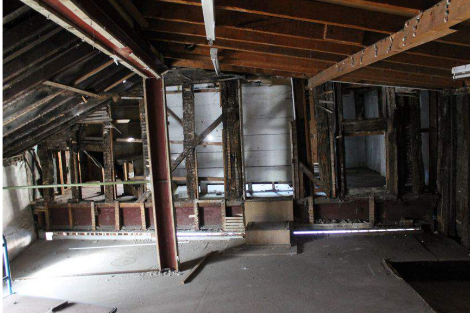
Photograph 39 Eastern elevation of exterior of first-floor of Building B, showing inserted doorway and window-frame. Also visible is metal beam supporting raised first-floor. Photograph taken facing west.
