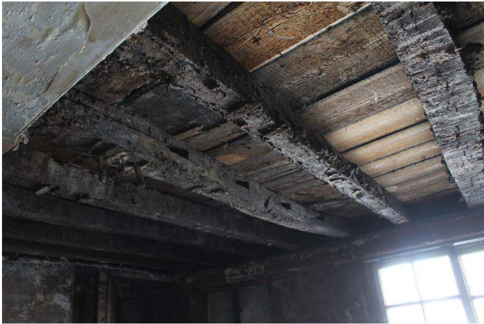
Photograph 59 Unused mortices on joist of second-floor of Building B. Photograph taken facing south-west.
