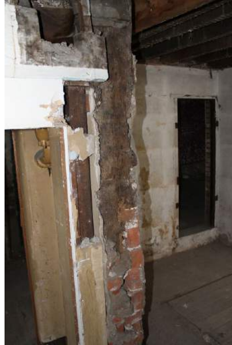
Photograph 8 Remains of south-east corner-post of Building A at the ground floor. Photograph taken facing north-east.
