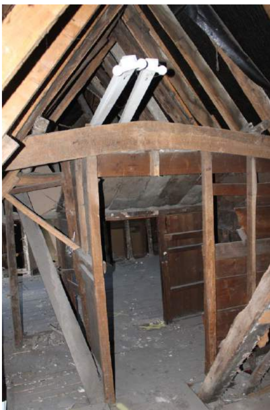
Photograph 32 Small timber room in the joining section of roof between the second-floor of Buildings A and B. Arched collar used as part of the structure. Photograph taken facing north.
