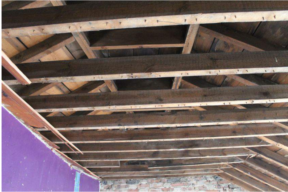
Photograph 77 Detail of roof in Building D, showing the tapering of the gambrel roof to a gable. Photograph taken facing east.
