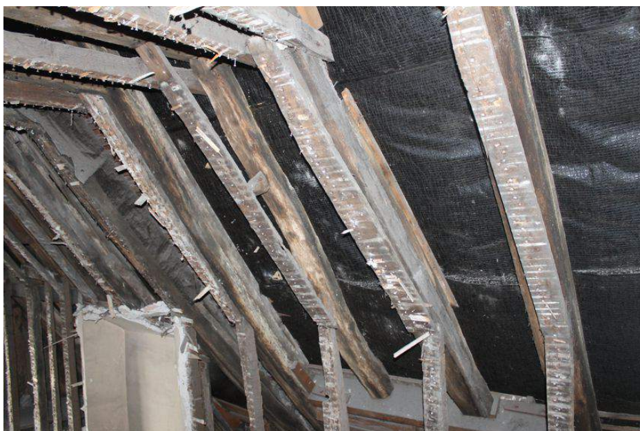
Photograph 27 Smoke-blackening on rafters in Building A. Shows variation in smoke-blackening from centre of building (right) outwards. Photograph taken facing north-west.
