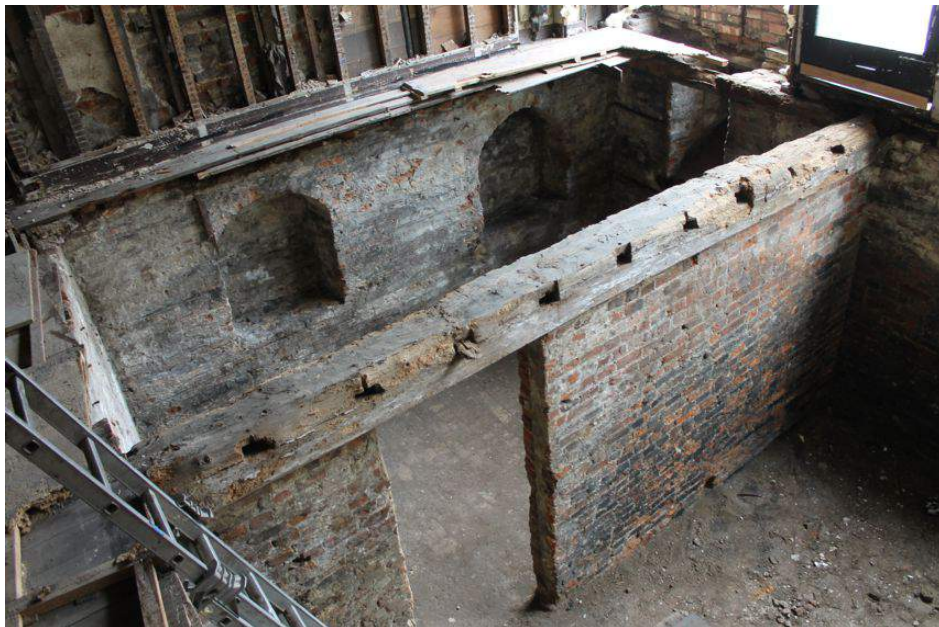
Photograph 41 Cellar beneath Building B, showing recesses for shelving. Photograph taken facing south-east.
