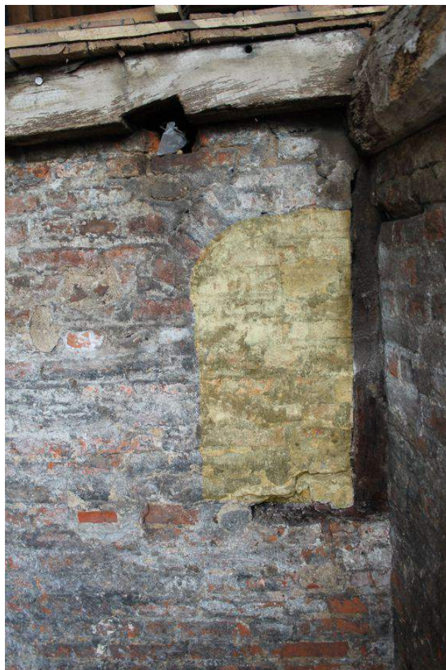
Photograph 50 Highlighted blocked archway in eastern wall of cellar, including post supporting binding-beam. Photograph taken facing east.
