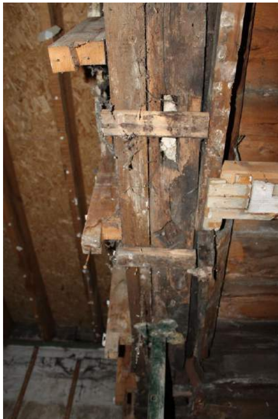
Photograph 13 Underside of girding-beam on eastern side of Building A. Diamond window mullions visible.
