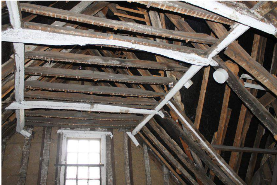
Photograph 60 Roof of Building B, showing original collars and purlins, as well as later braces. Photograph taken facing west.
