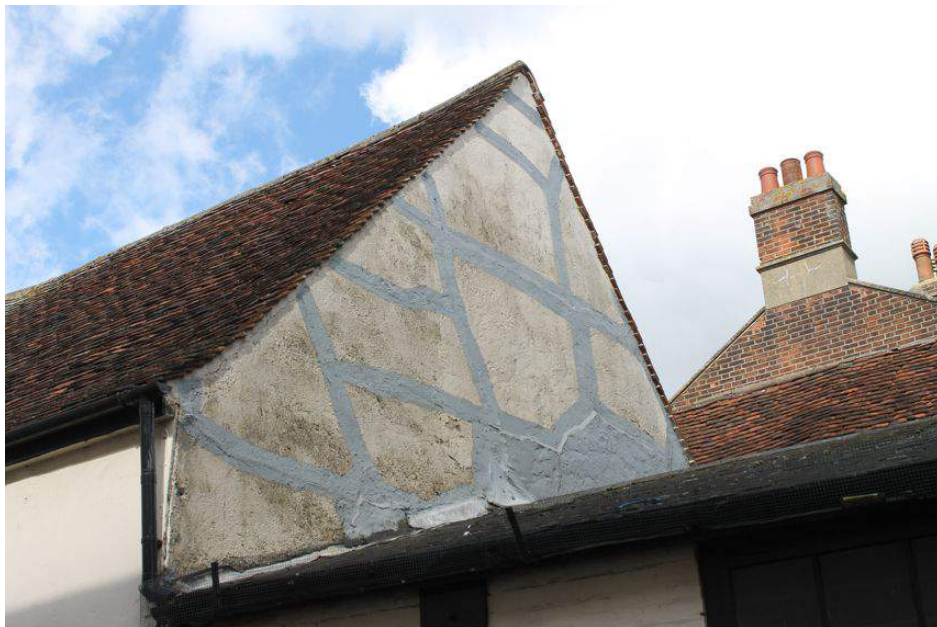
Photograph 38 Eastern gable-end of Building B, showing repairs to plaster. Photograph taken facing north-west.
