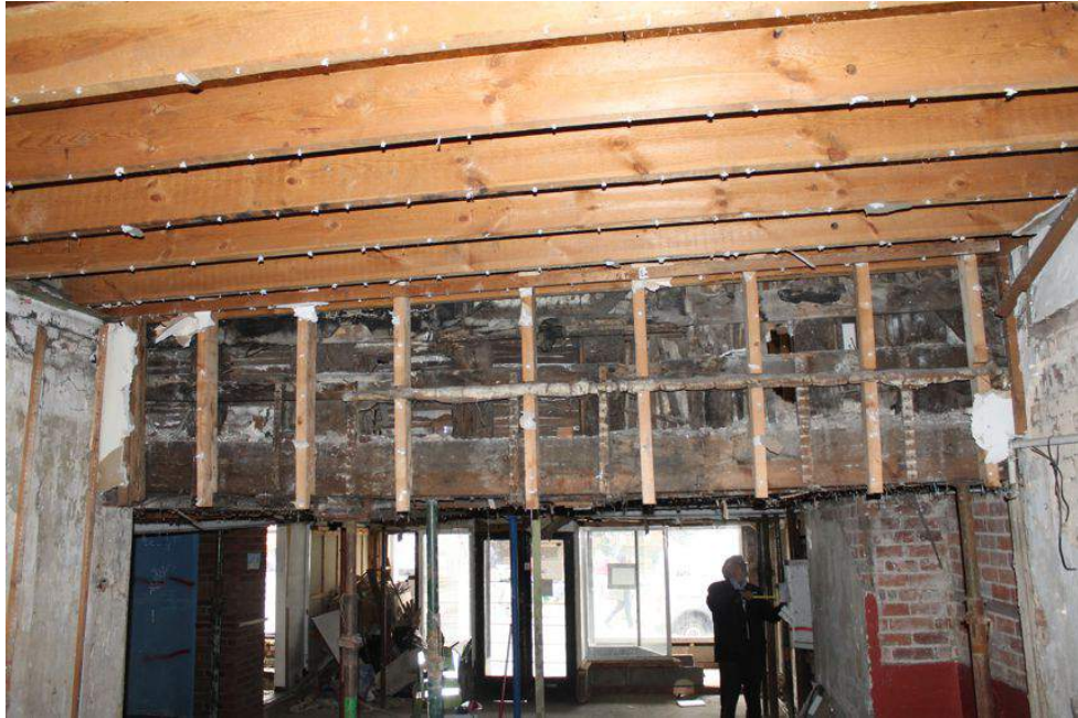
Photograph 12 Eastern elevation of Building A at ground level. Photograph taken within Building E and facing west.
