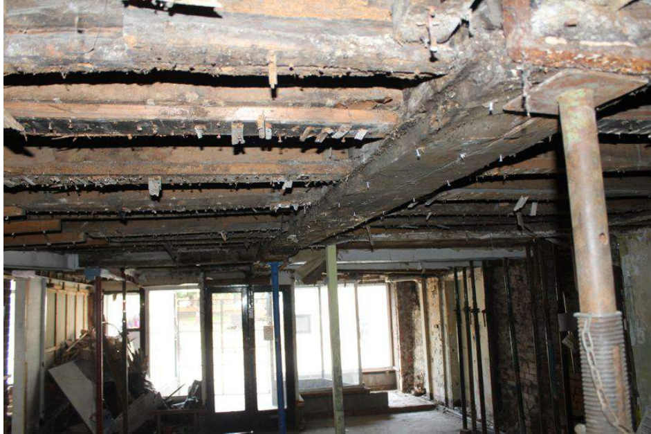
Photograph 14 Underside of first-floor in Building A. Chamfered binding-beam and supporting iron strap visible. Photograph taken facing west.
