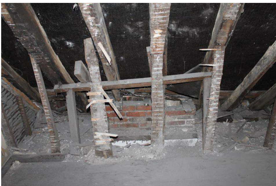
Photograph 35 Remaining top of chimney-stack in Building A. Possible original lath and plaster on east side of modern skylight visible to left. Photograph taken facing north.
