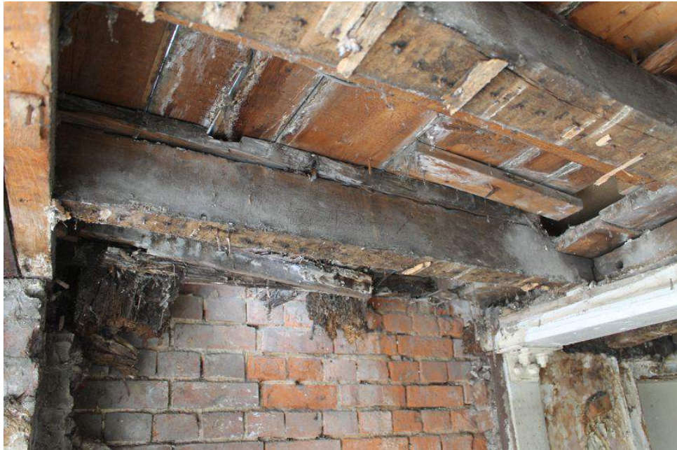
Photograph 11 Remains of current corner-post (left) and possible original corner-post projecting from first-floor (centre) on ground-floor on the northern elevation of Building A. Photograph taken facing north.
