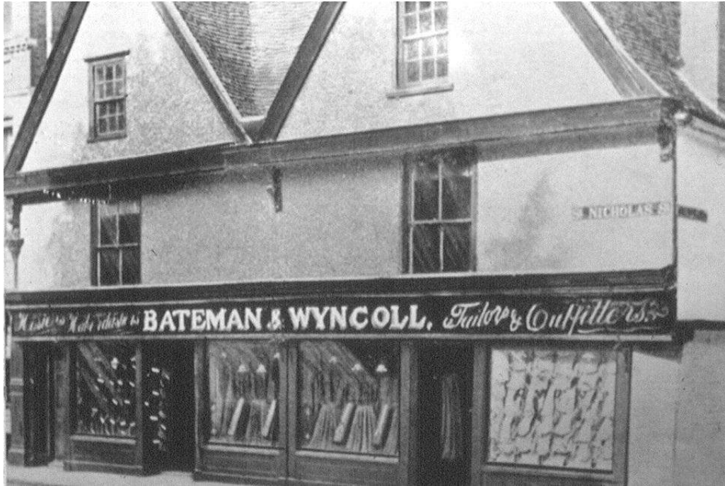
Photograph 1 Western elevation of 5 & 6 St Nicholas Street (Buildings A and B), taken in 1908. Note different windows and shop front (and lack of pargeting) compared to modern appearance (Photograph 2). Taken from www.gazette-news.co.uk/history/1528359.NOSTALGIA_Pictures_of_the_1d_JacksHardware_store_as_it_used_to_be Labelled as being from a Colchester Guide book in 1908.
