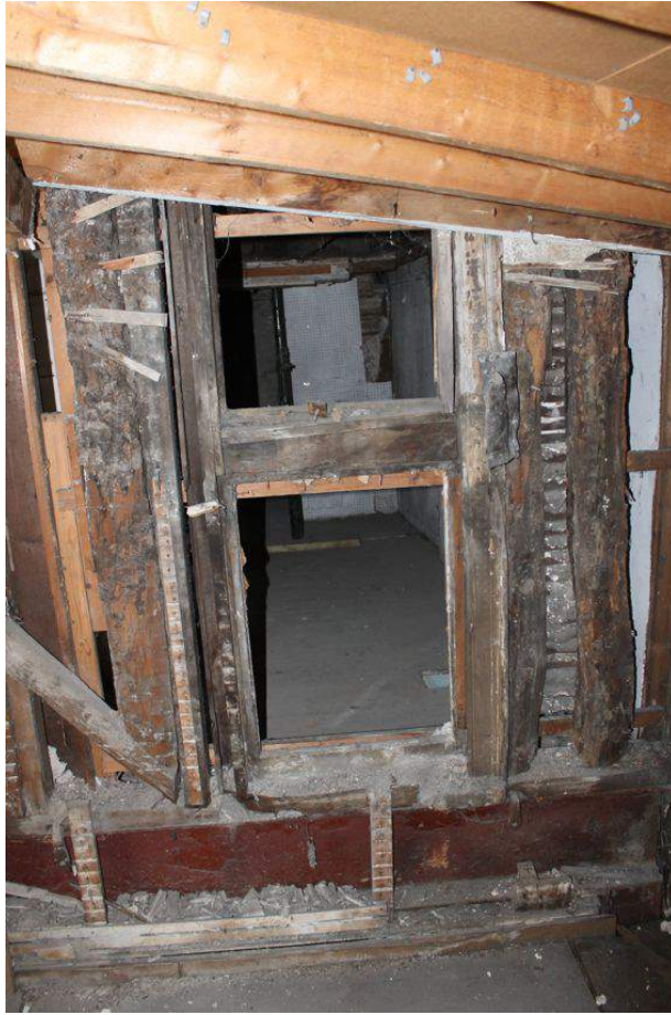
Photograph 55 Detail of inserted window-frame in east wall of Building B's first-floor. Photograph taken facing west.
