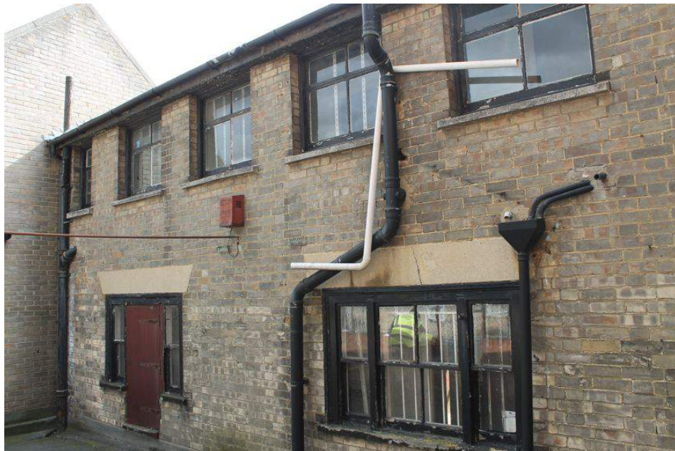
Photograph 72 Northern elevation of Building D. Photograph taken from roof of Building E, facing south-east.
