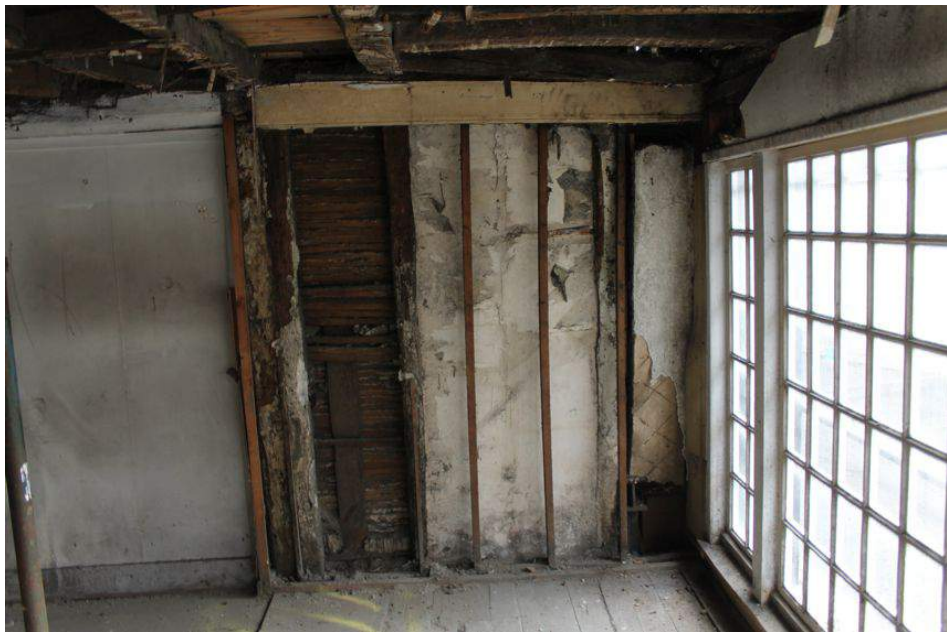
Photograph 20 Photograph of internal southern elevation of first-floor in Building A. Exposed lath and plaster render visible on exterior of building, as well as bricked over inserted door between Buildings A and B. Photograph taken facing south.
