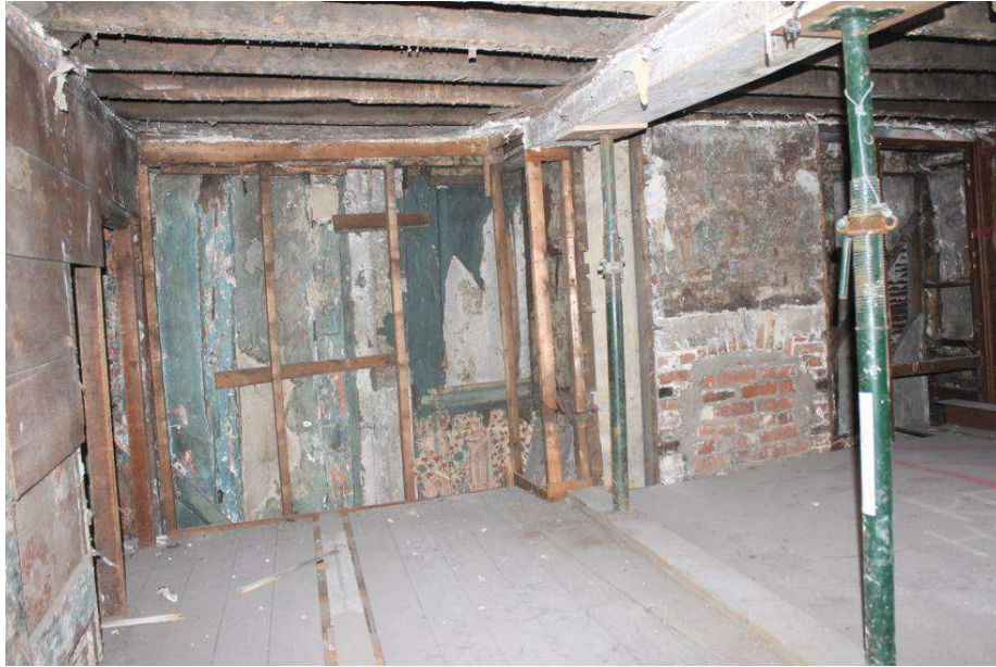
Photograph 57 Internal southern elevation of first-floor in Building B. Photograph taken facing south.
