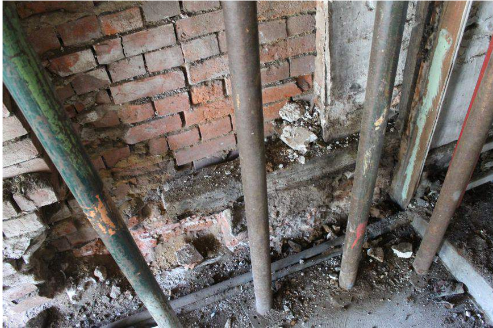
Photograph 9 Remains of sill-beam and brick plinth on northern elevation of Building A. Photograph taken facing north.
