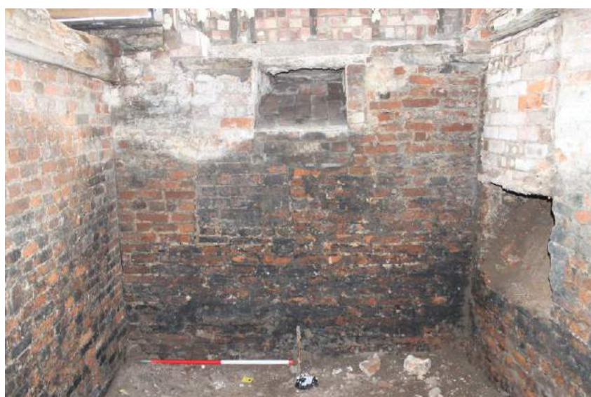
Photograph 46 Western elevation of northern room, showing coal chute replacing an earlier, bricked up, opening. Photograph taken facing west.
