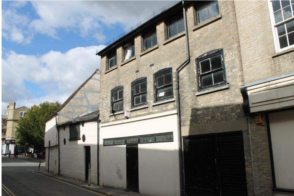
Photograph 70 Southern elevation of Building D in foreground, with Buildings D and B in background. Photograph taken facing north-west.
