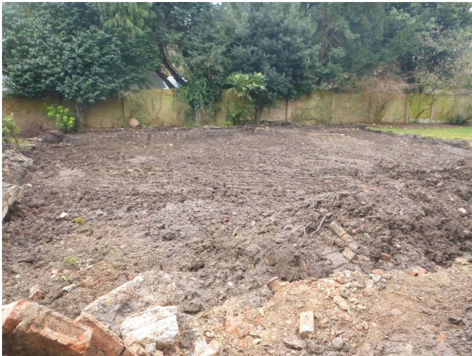
Photograph 1 Area of ground reduction
