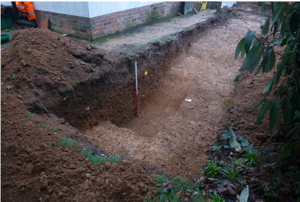
Photograph 1 F1, the central ditch of the Triple Dyke, looking SW
