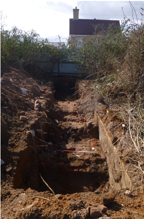
Photograph 1 Trench T1, showing the remains of the unexcavated demolished cellar, looking SW
