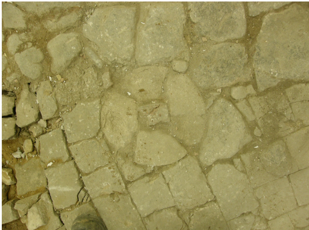
Photograph 3 Room 3, stone repair to brick pavior floor – view north-east.
